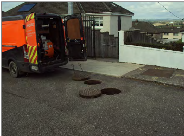
Manhole / Access Point: MHS.1 Location
