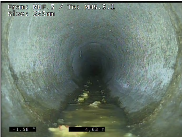
Debris 0% cross-sectional area loss
