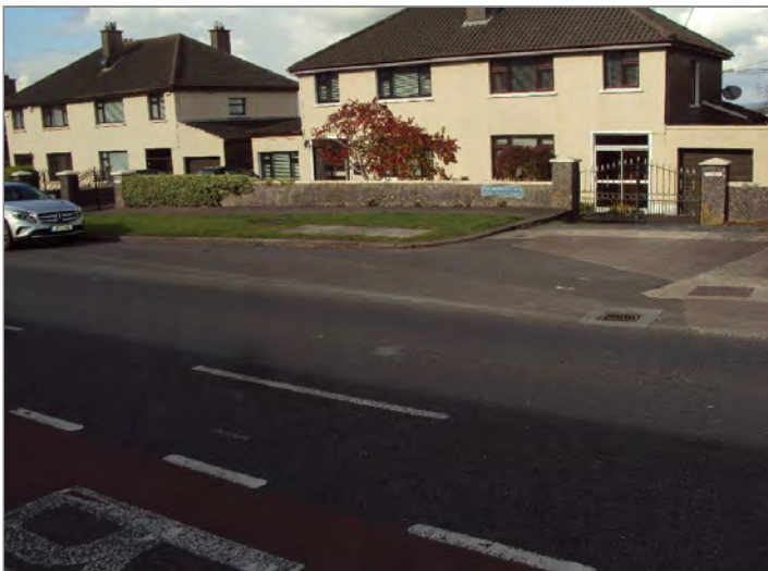
Manhole / Access Point: MHC.3 Location
