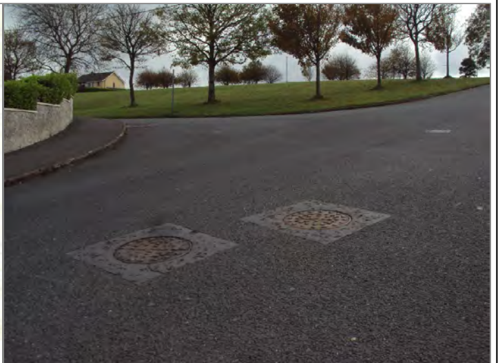
Manhole / Access Point: MHF.3 Location
