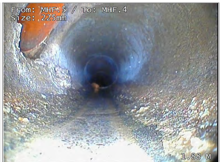
Connection at 10 o'clock, diameter 100mm - Remark: PVC
