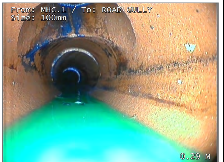
Connection at 12 o'clock, diameter 100mm - Remark: EW
