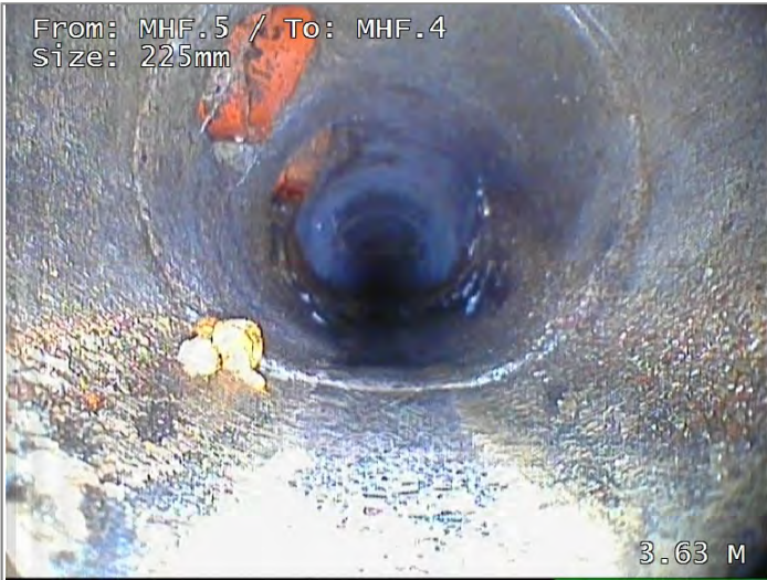
Connection at 11 o'clock, diameter 100mm - Remark: PVC
