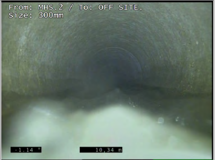
Manhole Finish (OFF SITE.)
