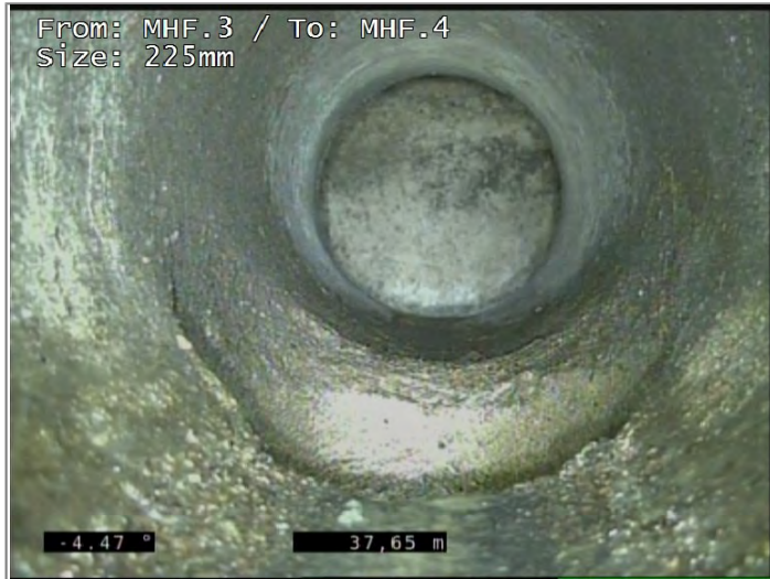
Line of sewer deviates down - Remark: DROP SHAFT INTO MHF.4
