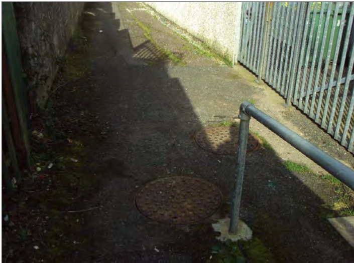
Manhole / Access Point: MHS.2 Location
