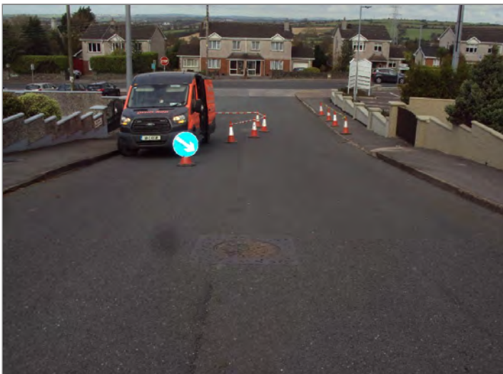
Manhole / Access Point: MHF.4 Location
