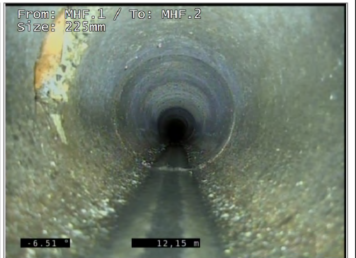
Connection at 10 o'clock, diameter 100mm - Remark: EW
