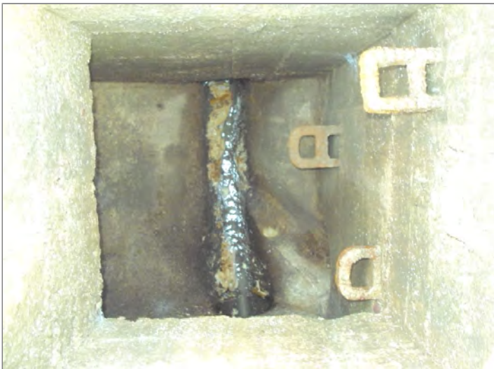
Manhole / Access Point: MHF.3 Internal
