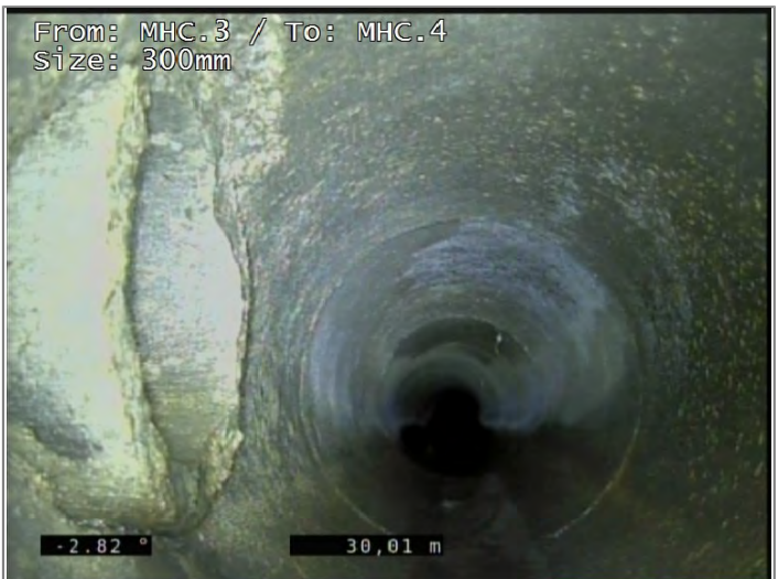
Connection at 9 o'clock, diameter 150mm
