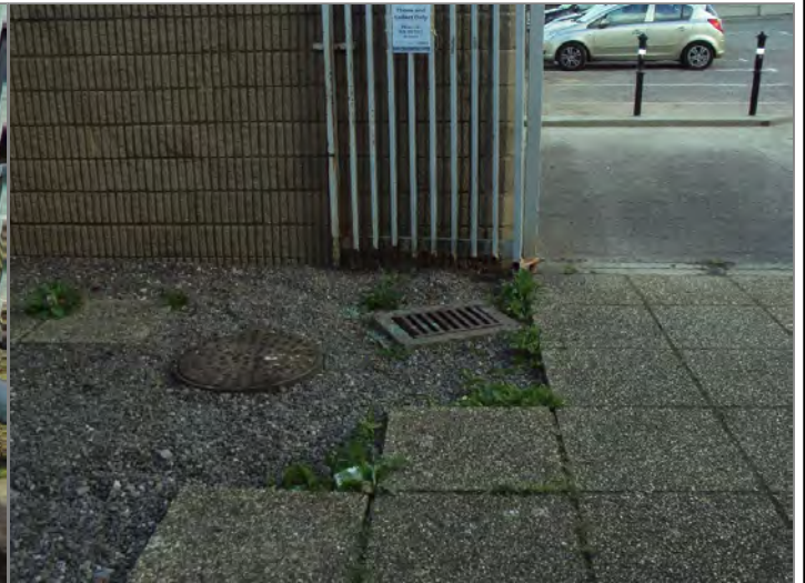
Manhole / Access Point: MHC.1 Location
