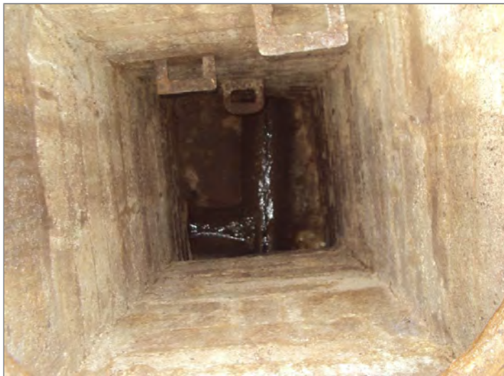
Manhole / Access Point: MHF.1 Internal
