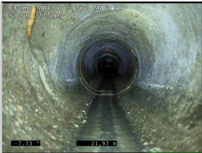
Connection at 10 o'clock, diameter 100mm - Remark: EW
