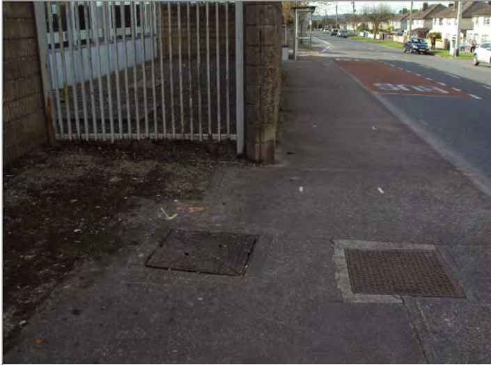
Manhole / Access Point: MHC.2 Location
