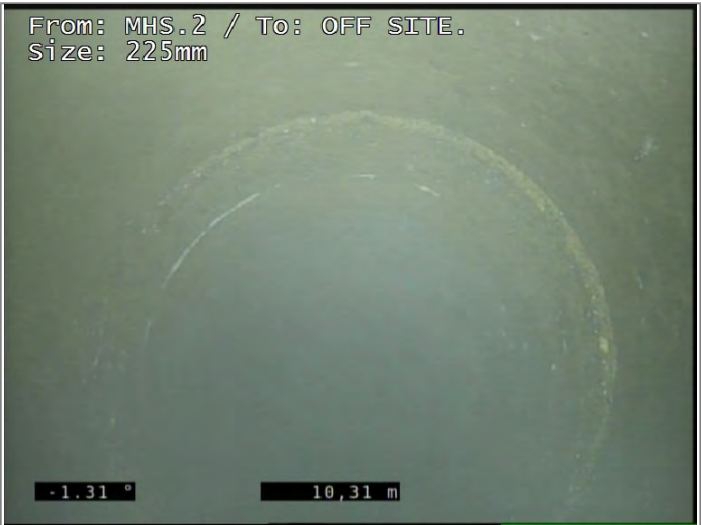
Manhole Finish (OFF SITE.)
