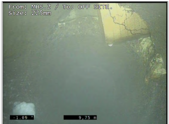
Connection at 2 o'clock, diameter 100mm - Remark: EW
