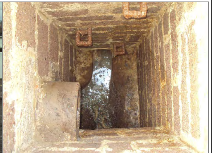
Manhole / Access Point: MHF.2 Internal
