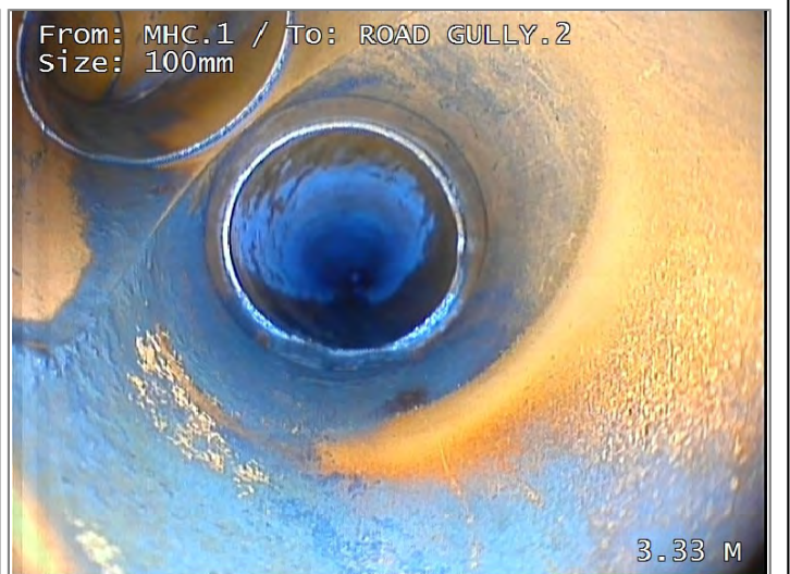
Connection at 11 o'clock, diameter 100mm - Remark: PVC.. ROAD GULLY.3
