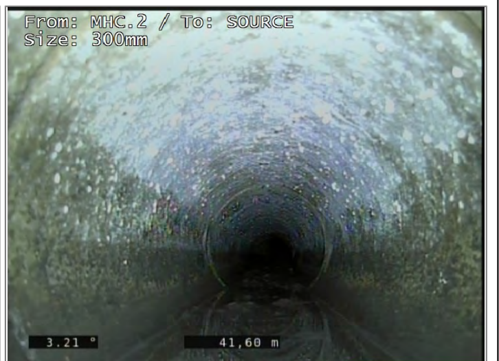
Survey abandoned - Remark: 15% DEBRIS + SILT IN LINE, VACTOR UNIT NEEDED TO DESILT LINES.
