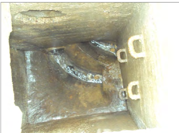
Manhole / Access Point: MHF.5 Internal
