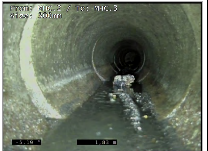
Joint displaced medium
