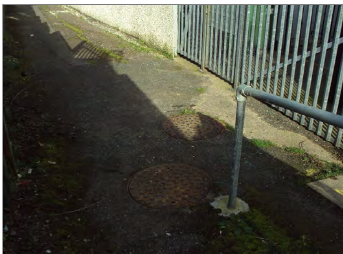
Manhole / Access Point: MHF.2 Location
