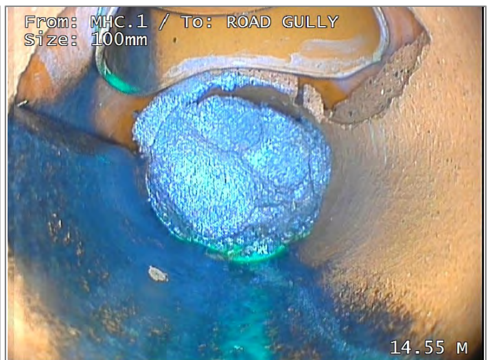
Manhole Finish (GULLY IN CAR PARK.)
