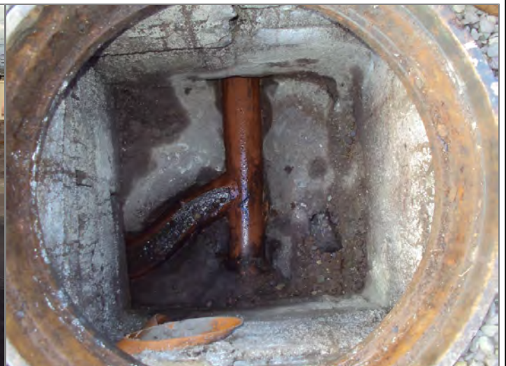
Manhole / Access Point: MHC.1 Internal
