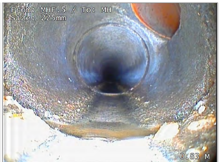
Connection at 1 o'clock, diameter 100mm - Remark: PVC
