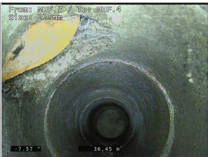
Connection at 10 o'clock, diameter 100mm
