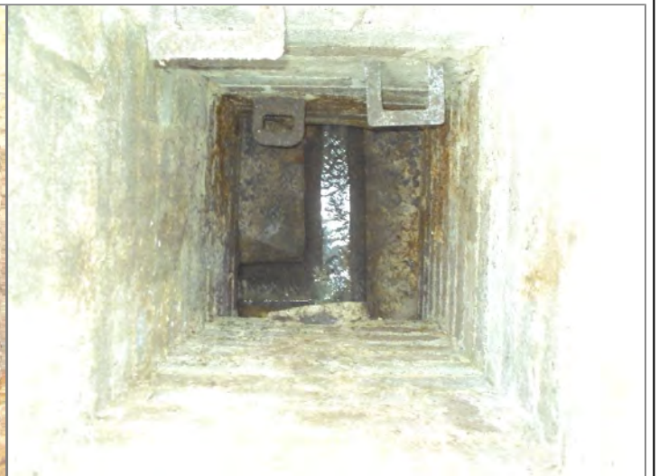
Manhole / Access Point: MHS.1 Internal
