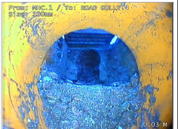
Manhole Finish (ROAD GULLY. 4)
