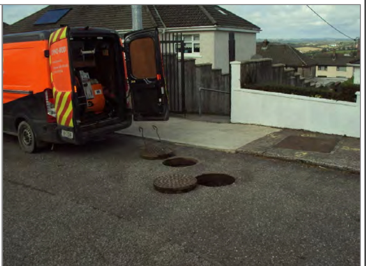
Manhole / Access Point: MHF.1 Location
