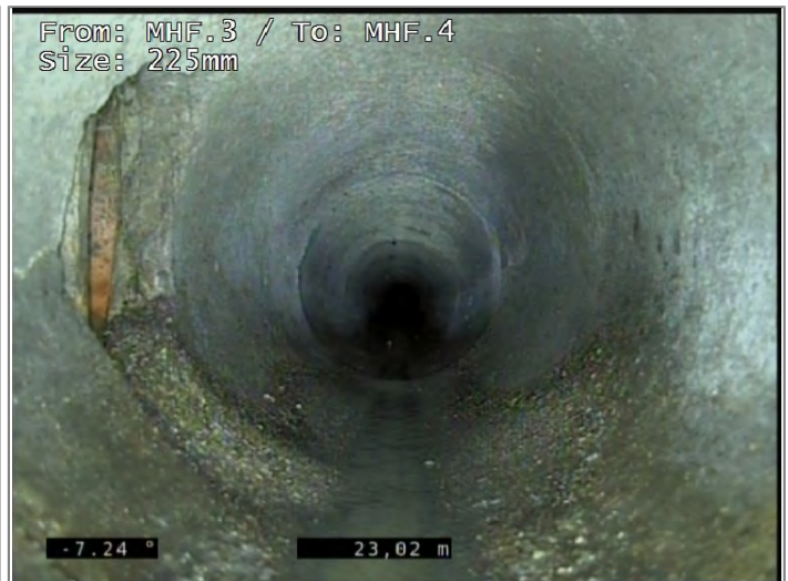
Connection at 9 o'clock, diameter 100mm - Remark: EW
