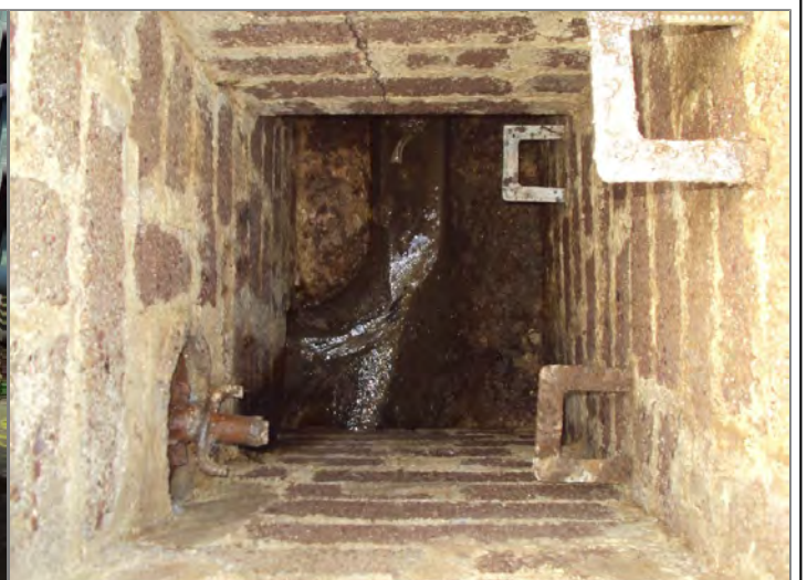
Manhole / Access Point: MHS.2 Internal
