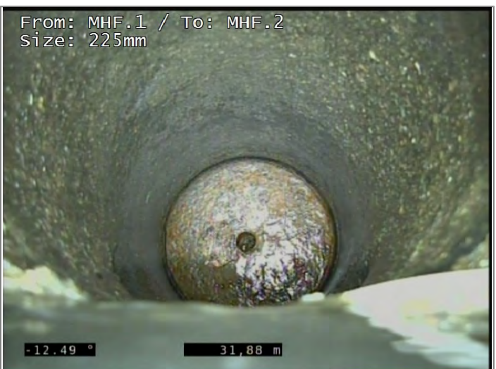
DROP SHAFT INTO MHF.2
