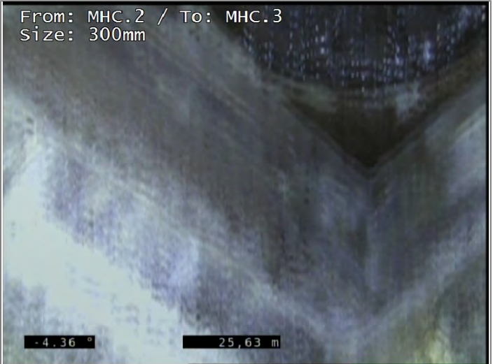
Manhole Finish (MHC.3)
