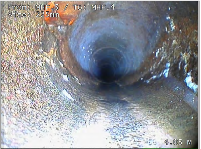
Connection at 11 o'clock, diameter 100mm - Remark: PVC
