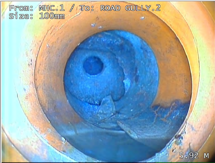
Manhole Finish (ROAD GULLY.2)
