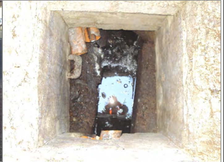
Manhole / Access Point: MHC.2 Internal
