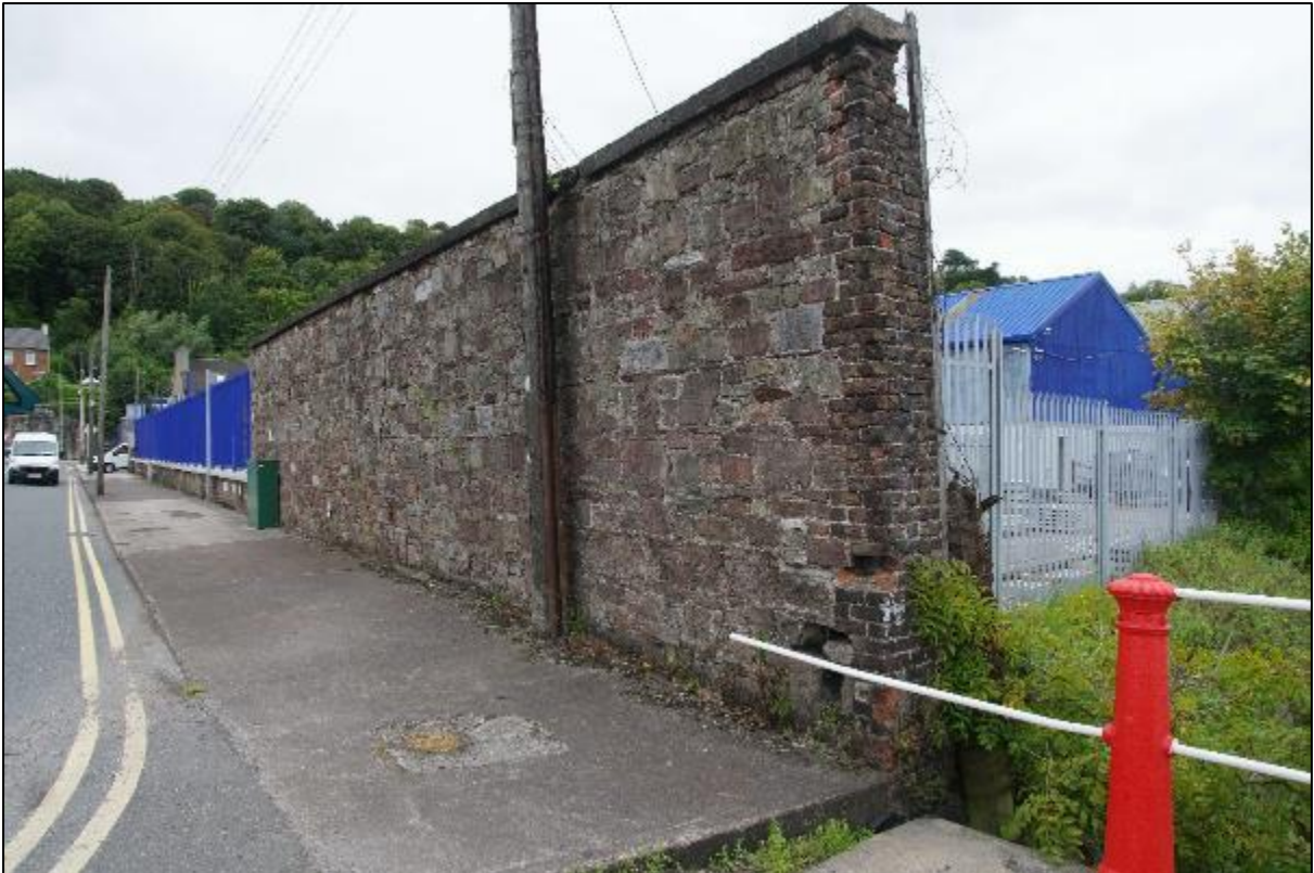
Plate 9: View from south of McMahon Builder Provision extant boundary wall on Water Street showing brick detail at south terminal and adjacent metal quay post to south.
