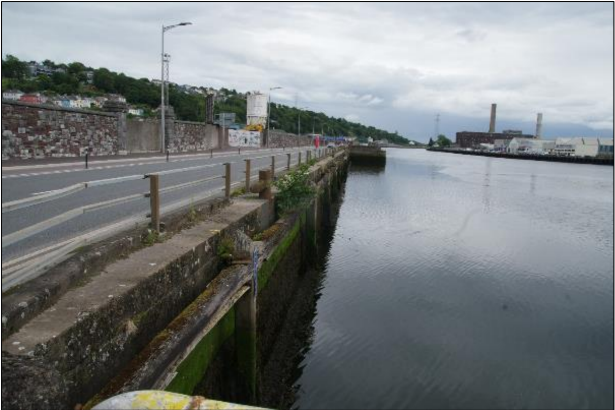
Plate 7: View of quay wall between wharves on Horgan's Quay
