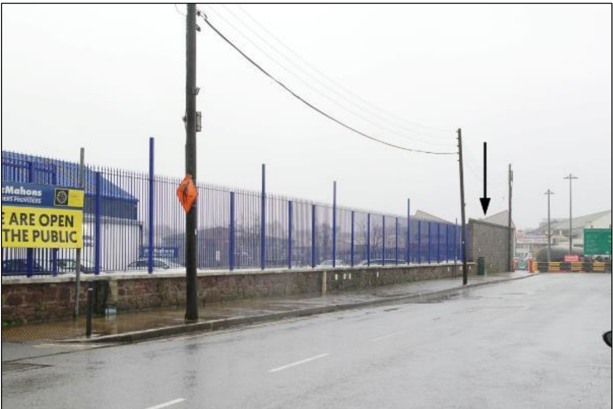
Plate 12: General view from north of McMahon Builder Provision extant boundary wall on Water Street showing modern fence set on top of basal remains of reduced boundary wall with section of south end of wall to be removed indicated by arrow (cross-refer with Figures 10 a and 10b)
