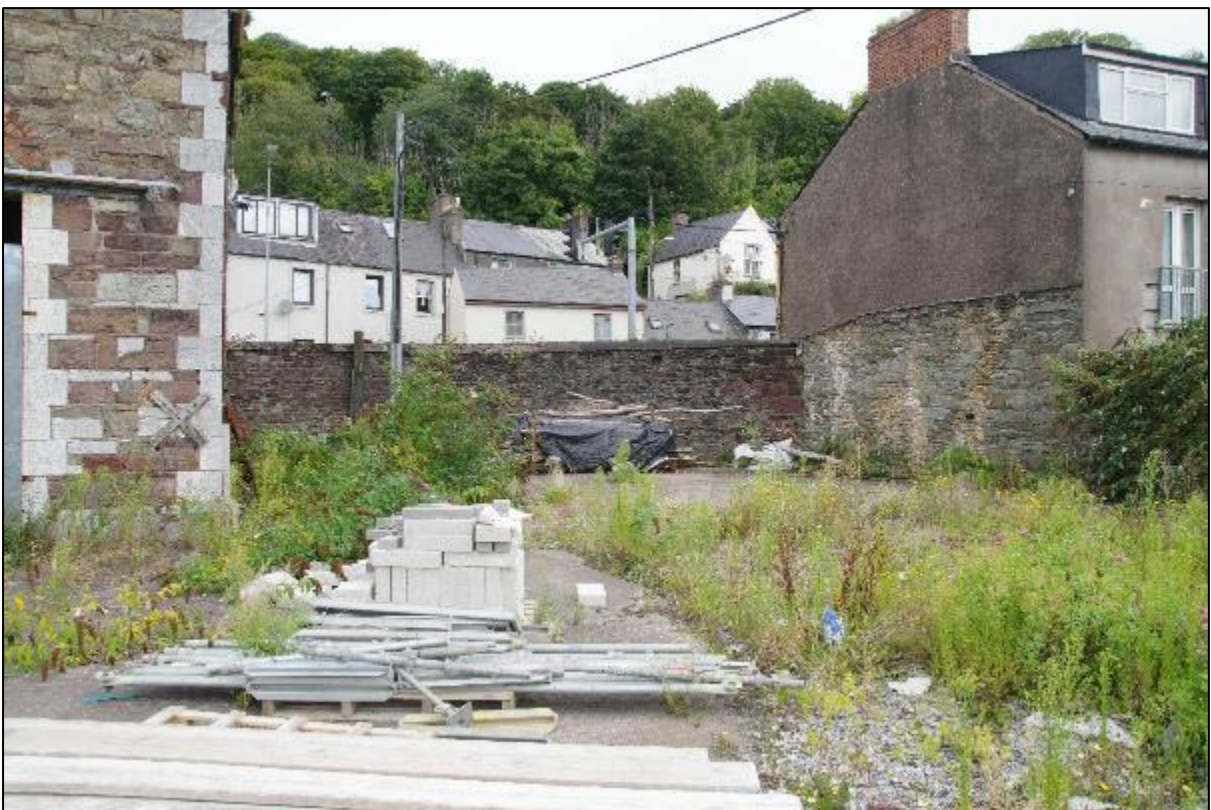
Plate 22: General view of northern boundary of the McMahon yard located on east side of workshop (CHC 7) visible on left side of frame
