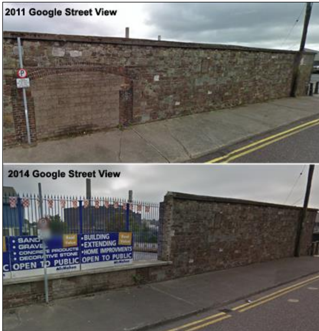
Figure 10b: Extracts from Google Street View images showing extent of modern removal of McMahon’s west boundary wall from northwest (section to be removed as part of proposed scheme on right)
