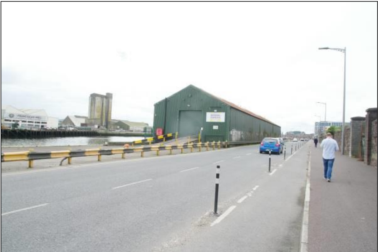
Plate 8: View of structure on west end of Horgan's Quay from east (to be retained)
