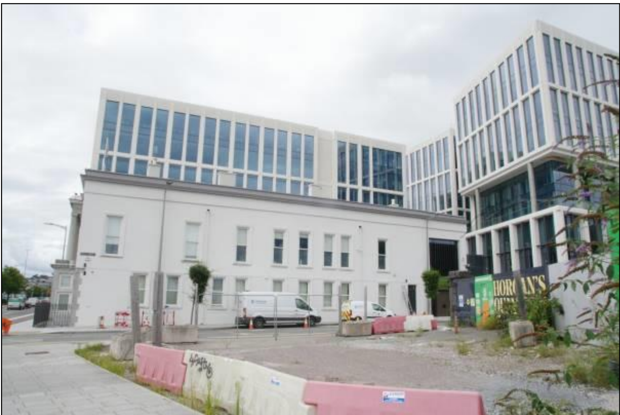
Plate 2: View of Steam Packet Office (CHC 1) from east
