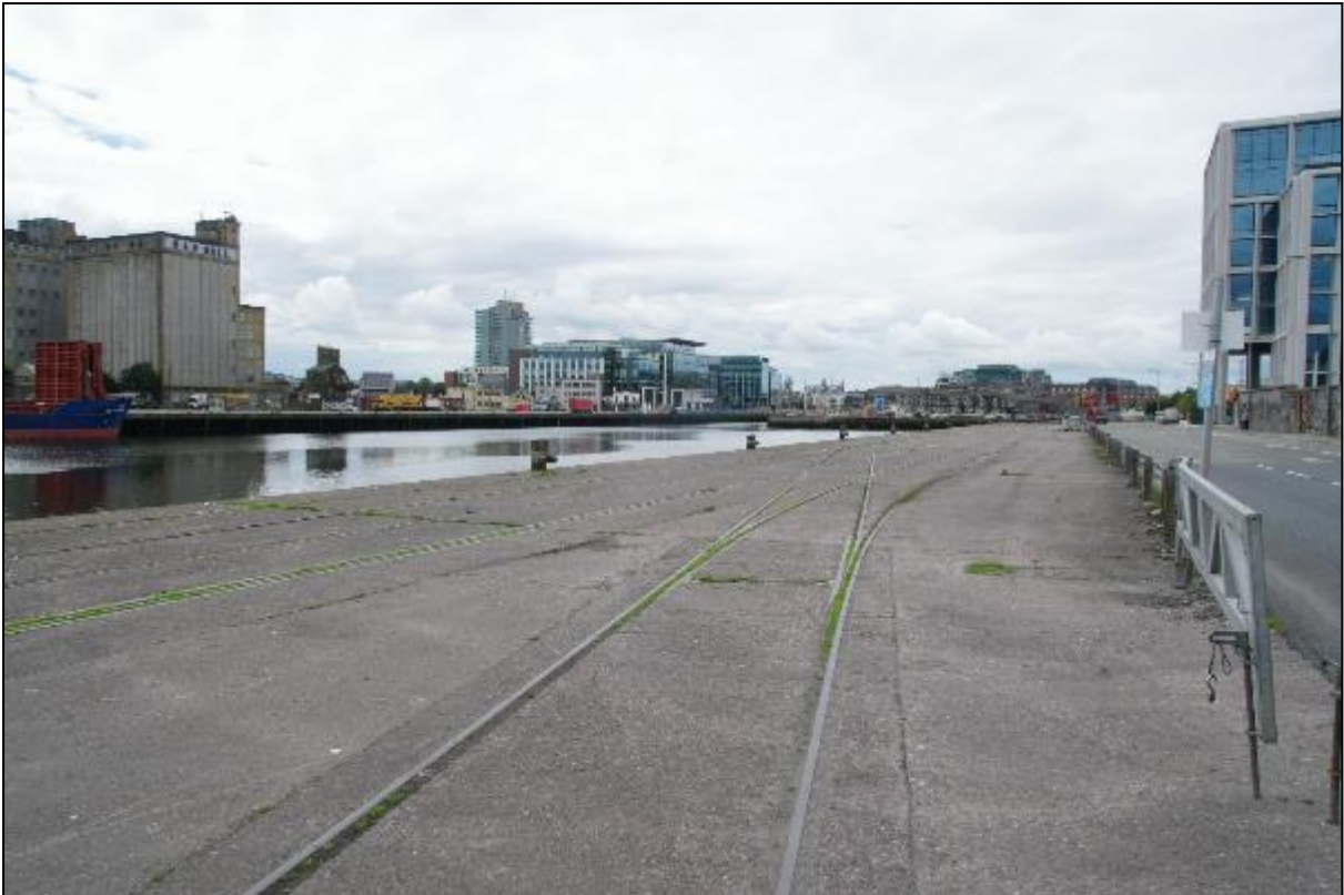
Plate 5: View of Horgan's Quay wharf (CHC 3) from east with crane rails visible in foreground
