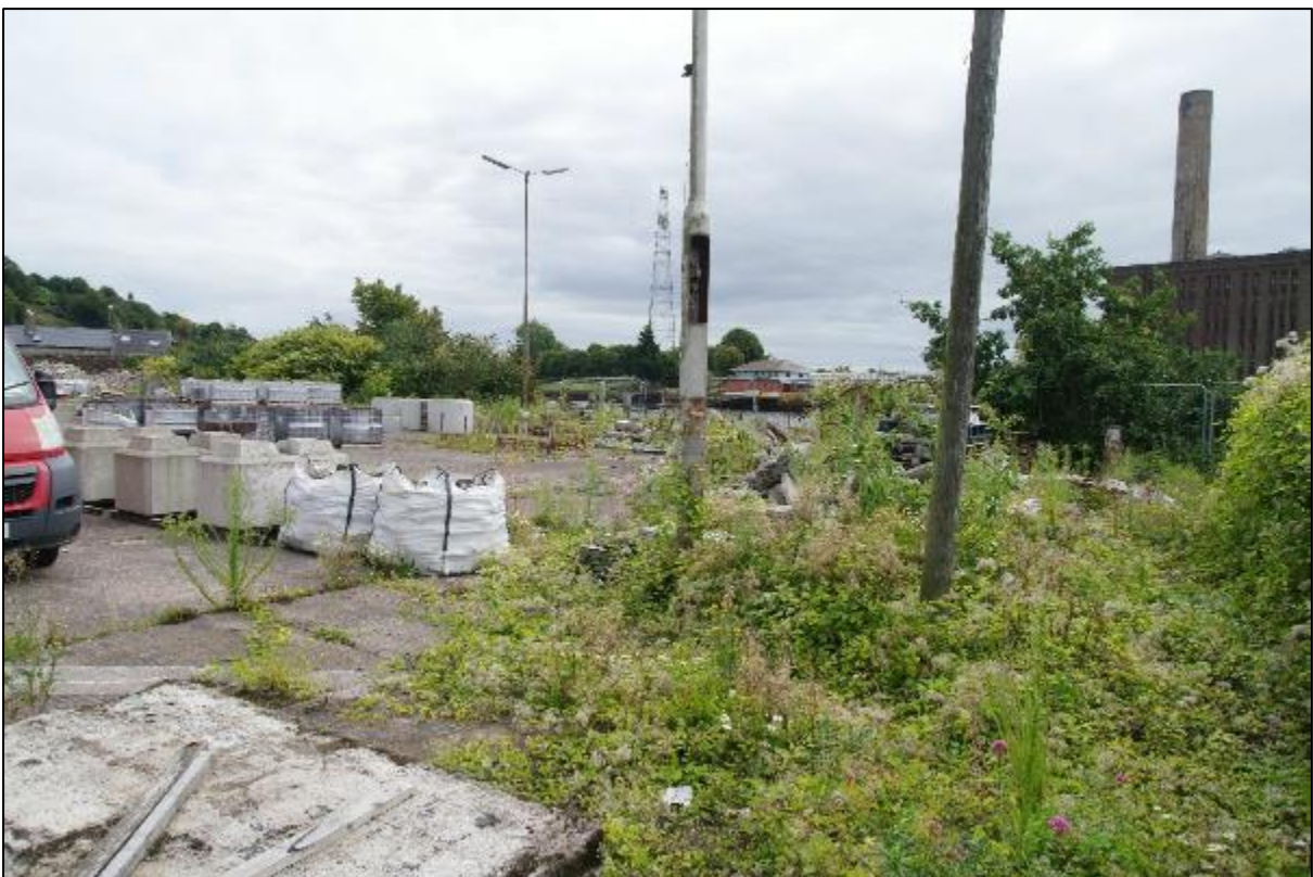
Plate 14: General view of former shipyard area within south end of McMahon Builder Provision premises from west with overgrowth and stored materials visible
