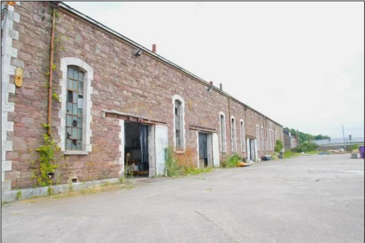
Plate 21: View of Port of Cork workshop (CHC 7) in north end of McMahon's yard from southwest (located outside scheme boundary)
