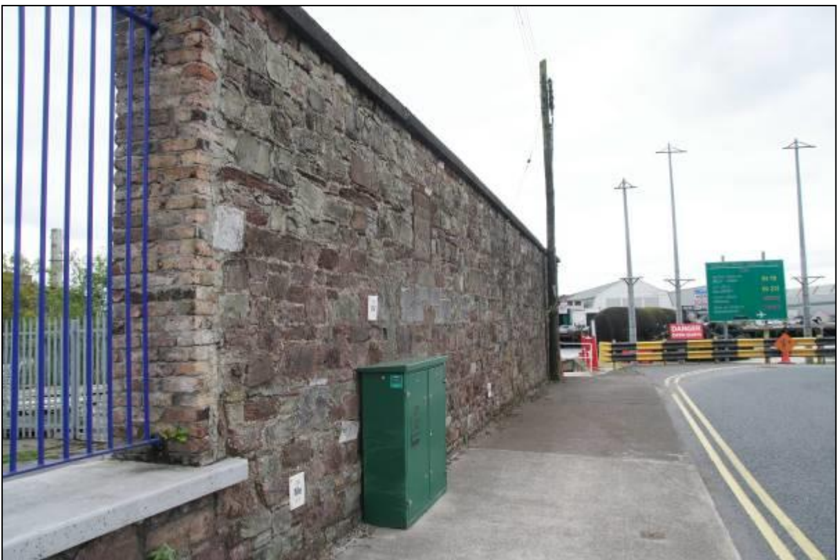
Plate 10: View from north of McMahon Builder Provision extant boundary wall on Water Street showing modern brick inset at north terminal
