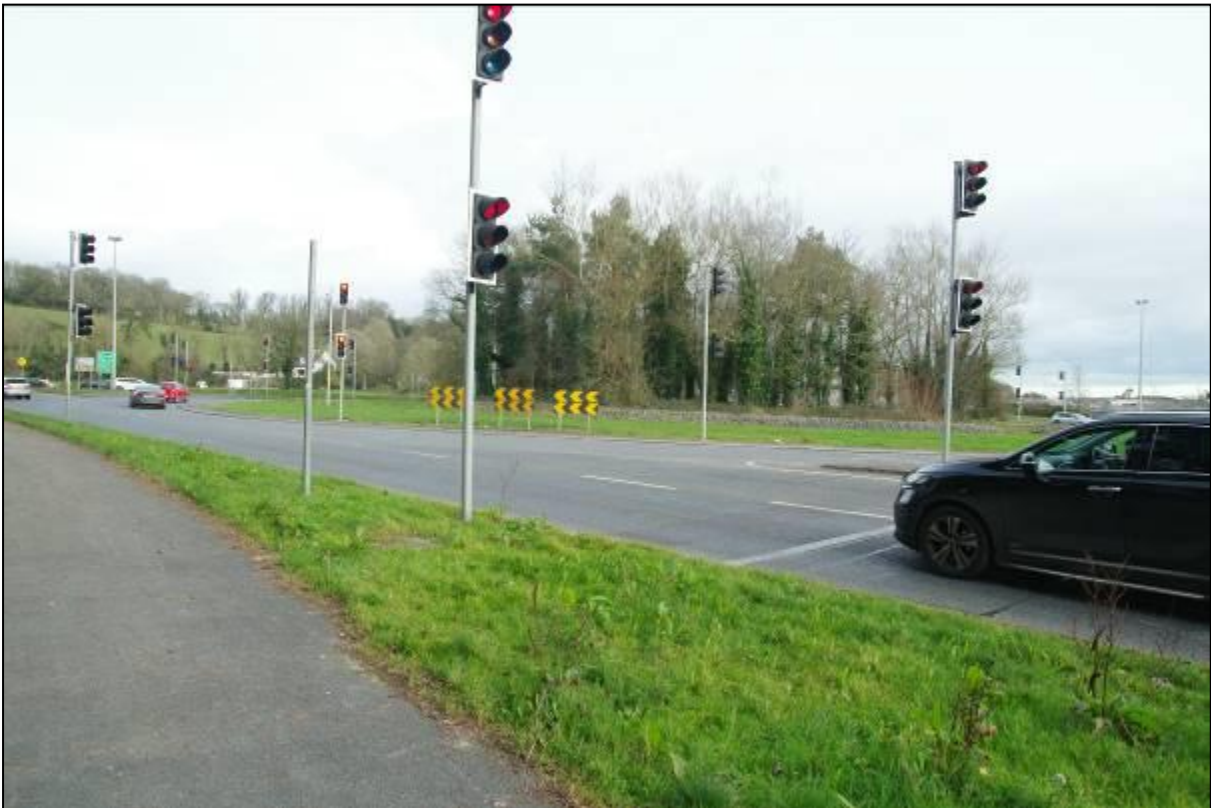
Plate 32: View of Lower Glanmire Road roundabout at east end of scheme
