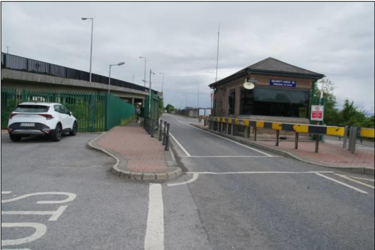
Plate 28: View of existing road within Tivoli Docks area from west
