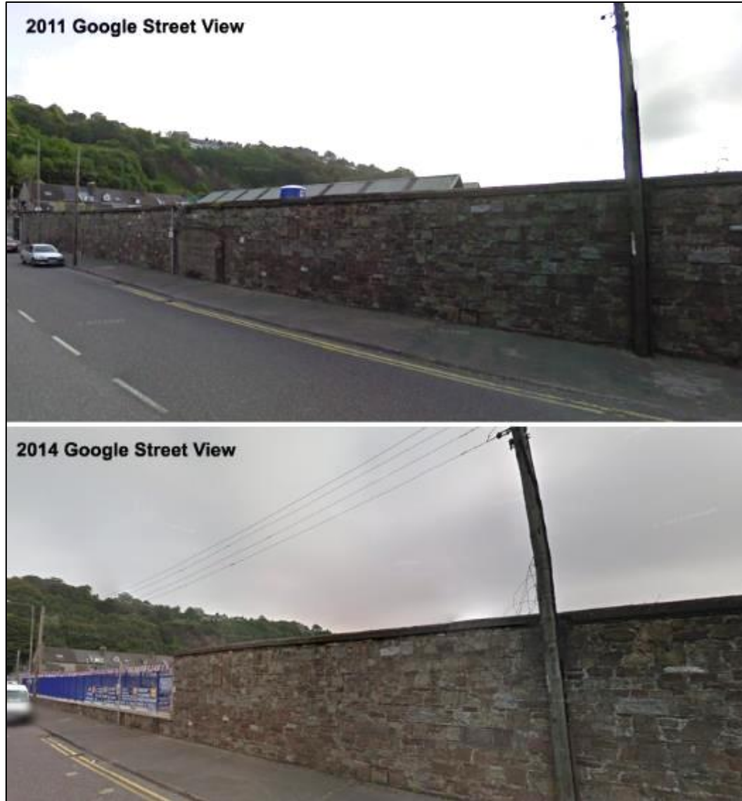
Figure 10a: Extracts from Google Street View images showing extent of alterations to McMahon's west boundary wall from southwest
