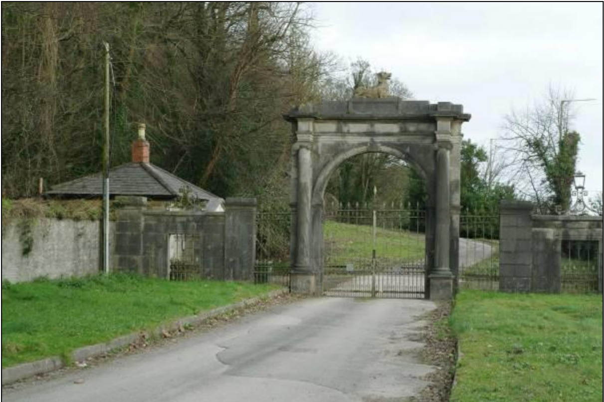
Plate 29: View of Lotabeg gateway (CHC 19) from west
