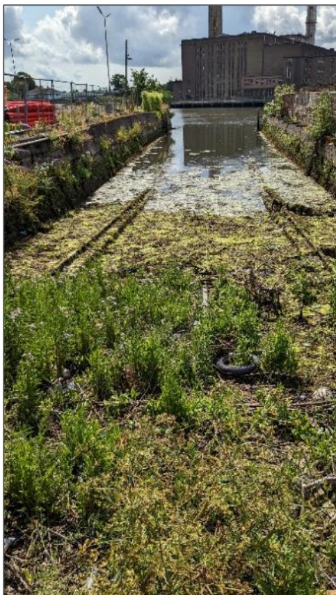
Plate 4-6 – Bridge will be installed to cross Dry dock.
