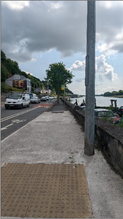
Plate 4-7 – Lower Glanmire Road heading East - existing Stone wall to be retained
