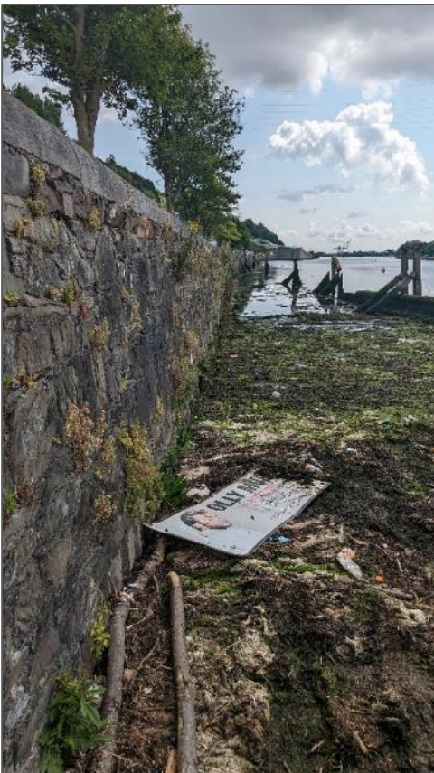
Plate 4-8 –Stone wall to be retained
