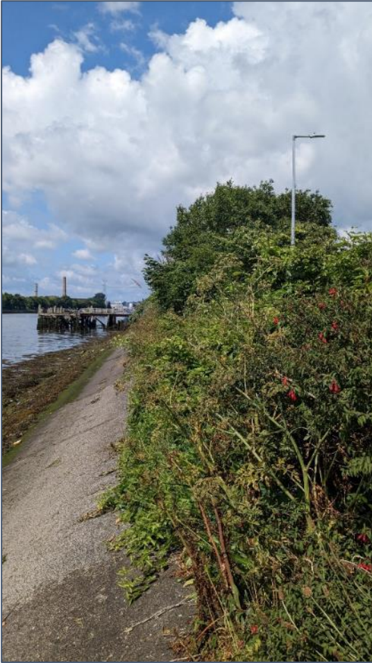
Plate 4-12 – Existing slope into the harbour ca. 3m
