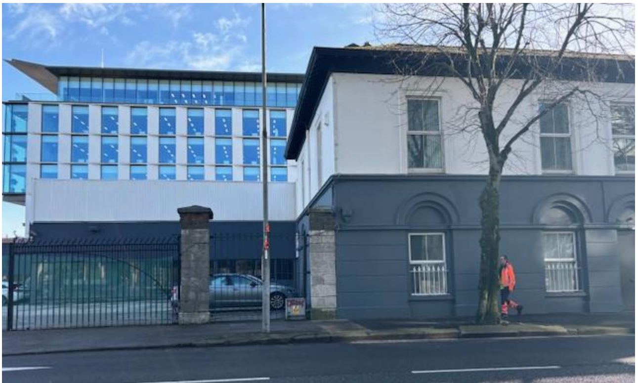
Photo A2 – Existing Footpath Damaged adjacent to the development site
