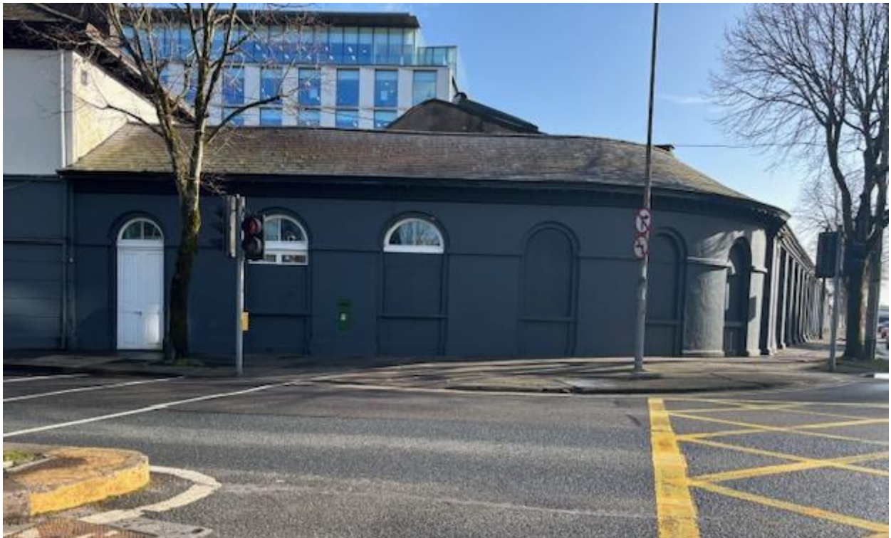
Photo A1 – Existing Footpath Damaged adjacent to the development site
