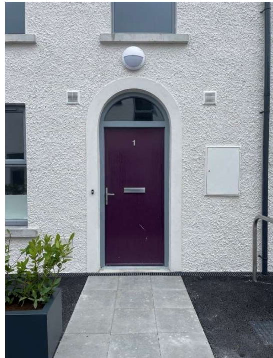
Example of pre-coloured wet dash finish with smooth plaster banding
