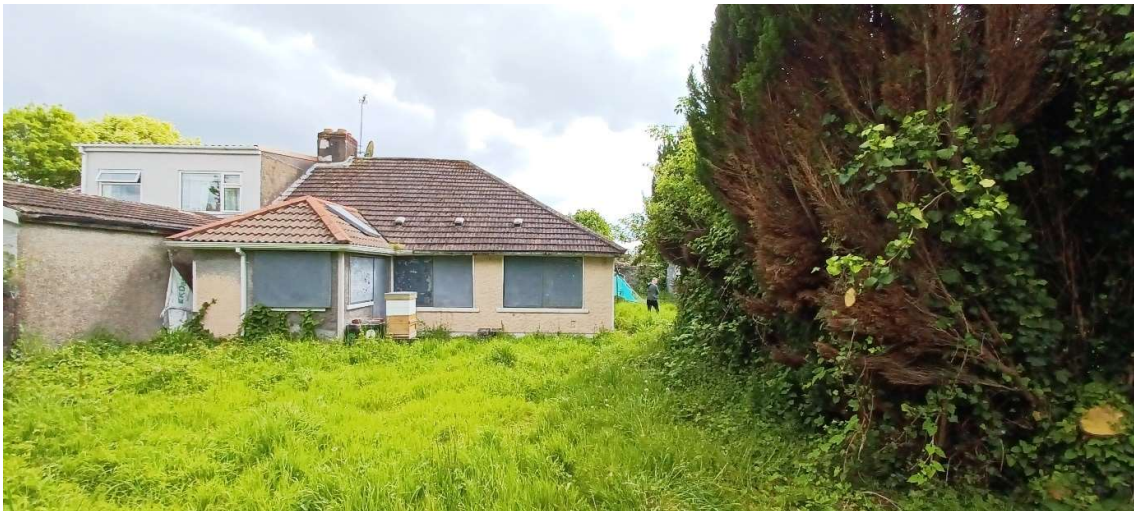
Fig. 10 : Rear view of the existing bungalow and adjacent bungalow looking East
