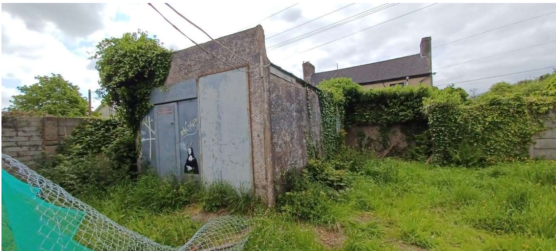
Fig. 11 : Detailed view of the existing shed and adjacent property looking South
