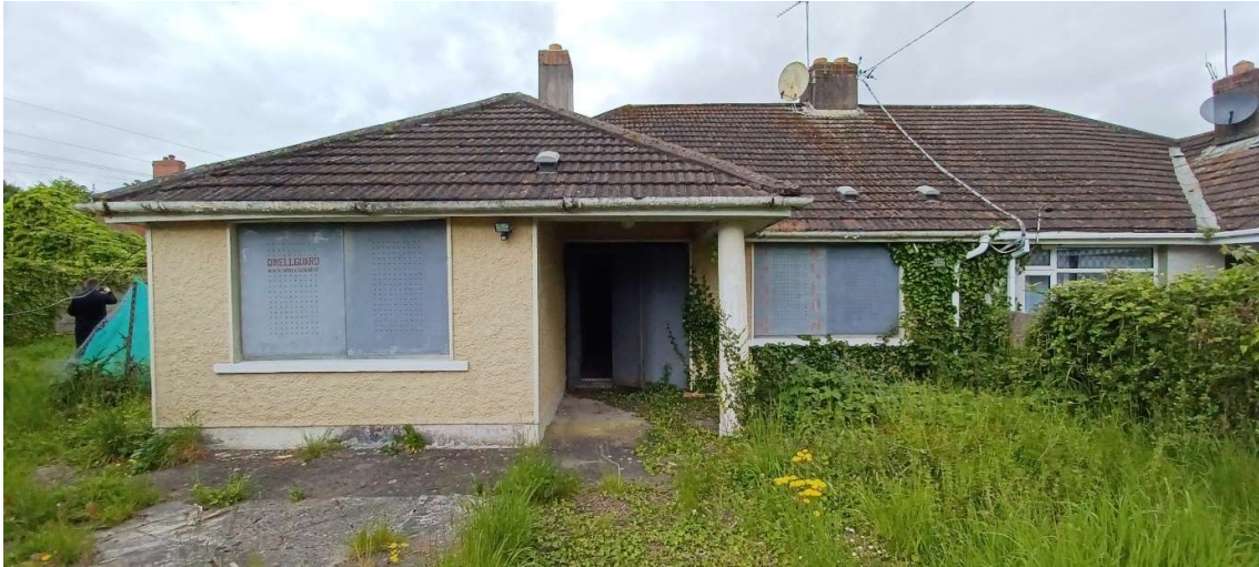
Fig. 22: Photo of existing bungalow to be demolished.
