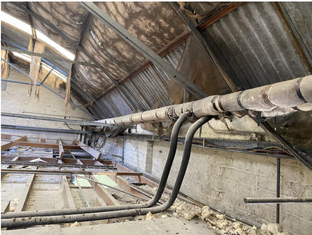
View of the asbestos cement sheeting internally
