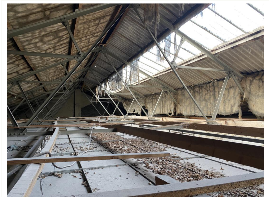
View of the asbestos cement sheeting internally
