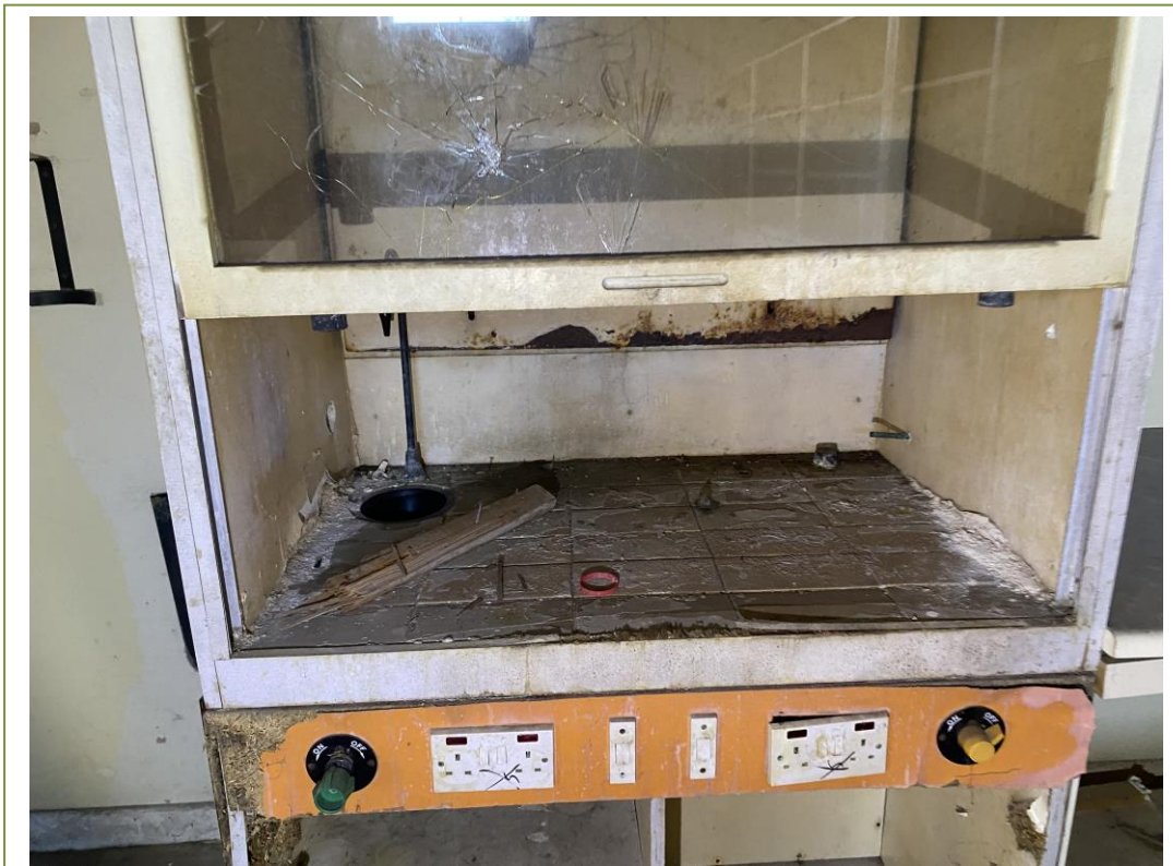
Insulation board sampled around flume hood in the lab
