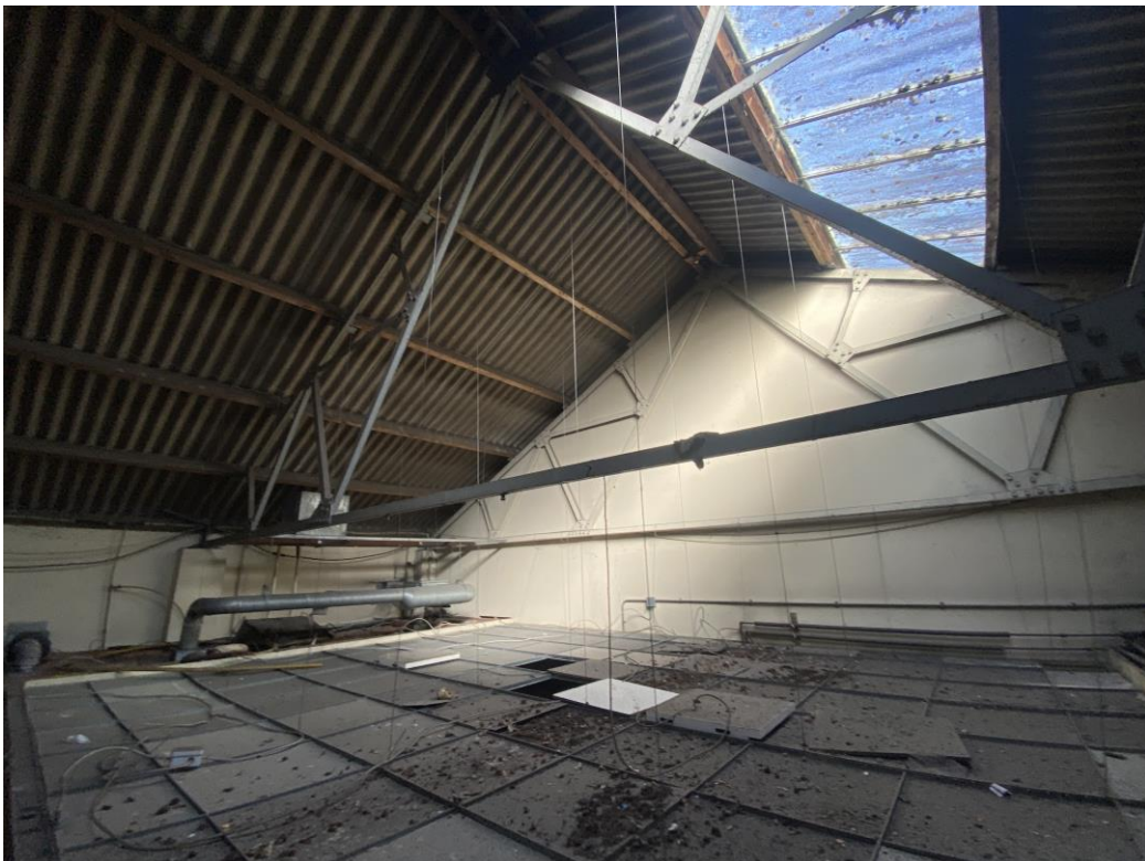
View of the asbestos cement sheeting internally
