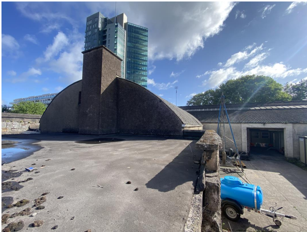
View of the asbestos cement sheeting externally
