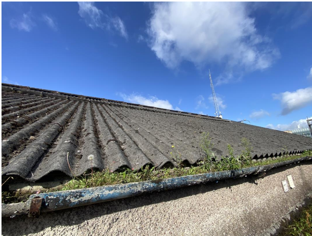
View of the asbestos cement sheeting externally
