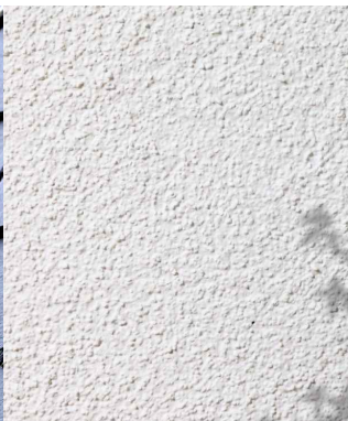
2. SMOOTH RENDER FINISH PAINTED WHITE (BLUE TO CIRCULATION TOWER).
