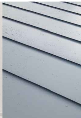
4. STANDING-SEAM ZINC CLADDING.
