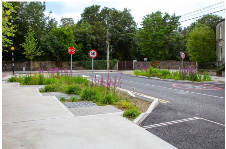
Raingarden to street verge Crescent Sea Rd, Galway City
