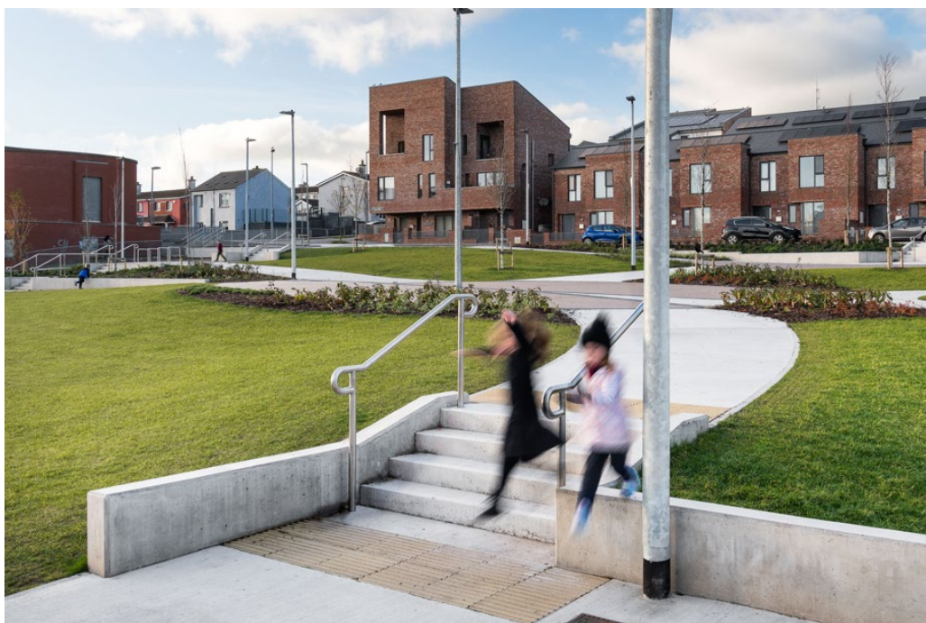
Changes in level creating opportunities for play CNWQR Phase 2A, Knocknaheeny, Cork by City Architects Department
