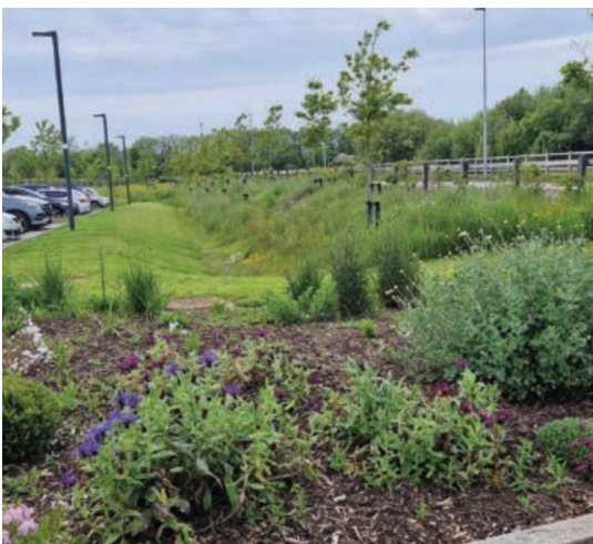
Dry Swale Min Ryan Park, Co. Wexford
