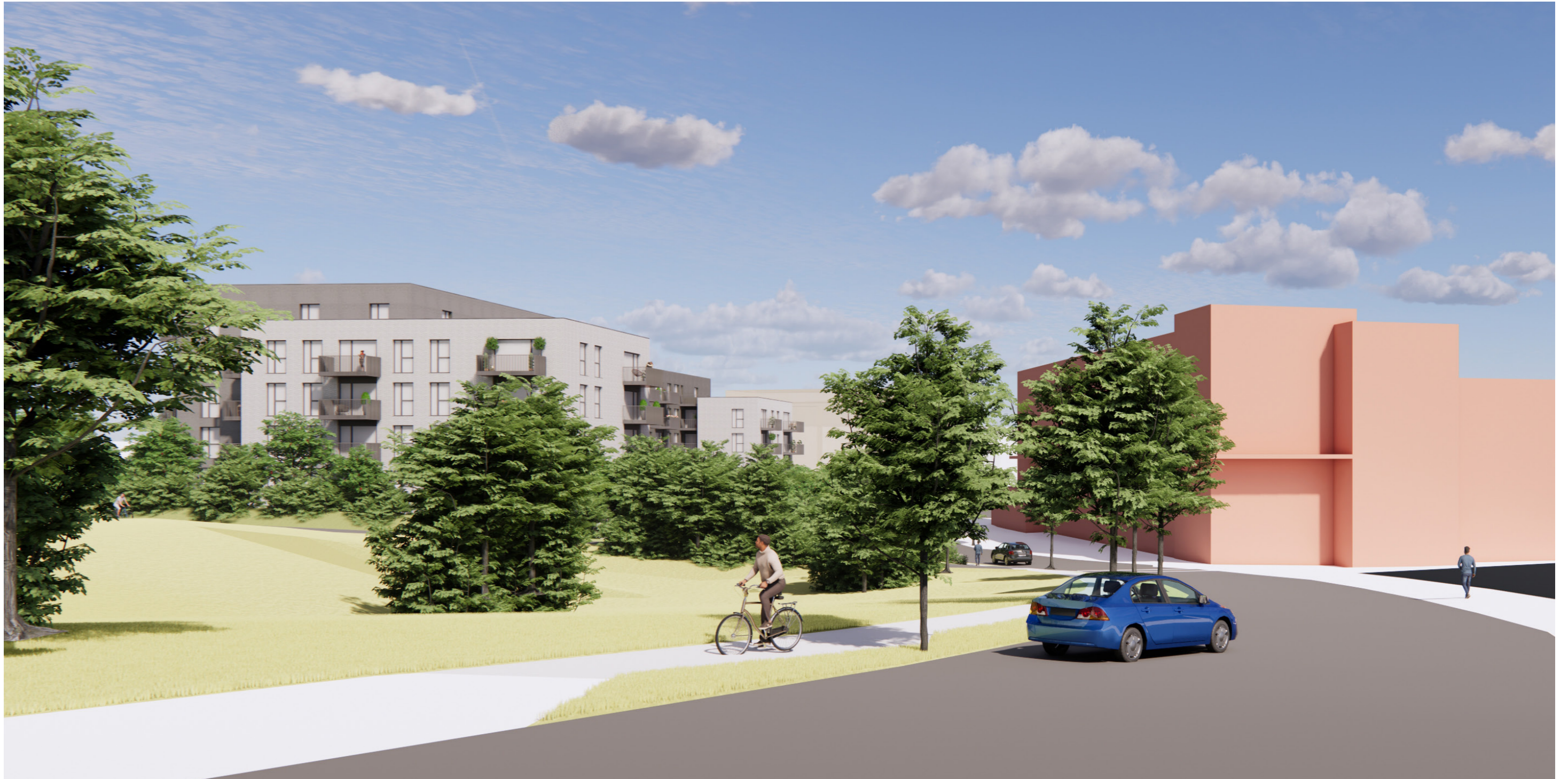
View 1 from Blackrock Avenue looking north
