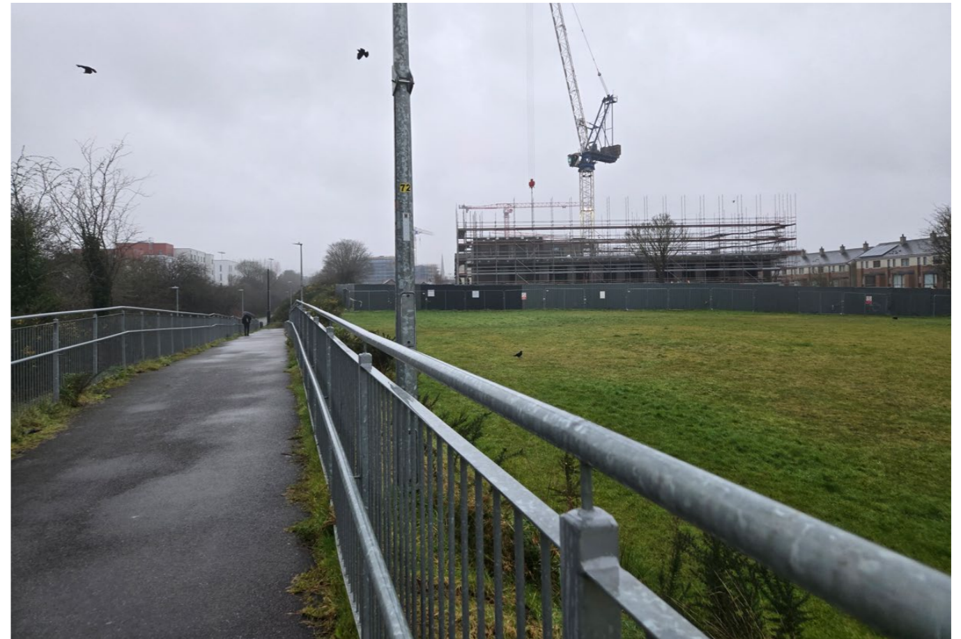
Fig. 4.0 – View north-eastwards from the Passage Railway Greenway 'slip' link with Eden Hall (under construction in the background)
