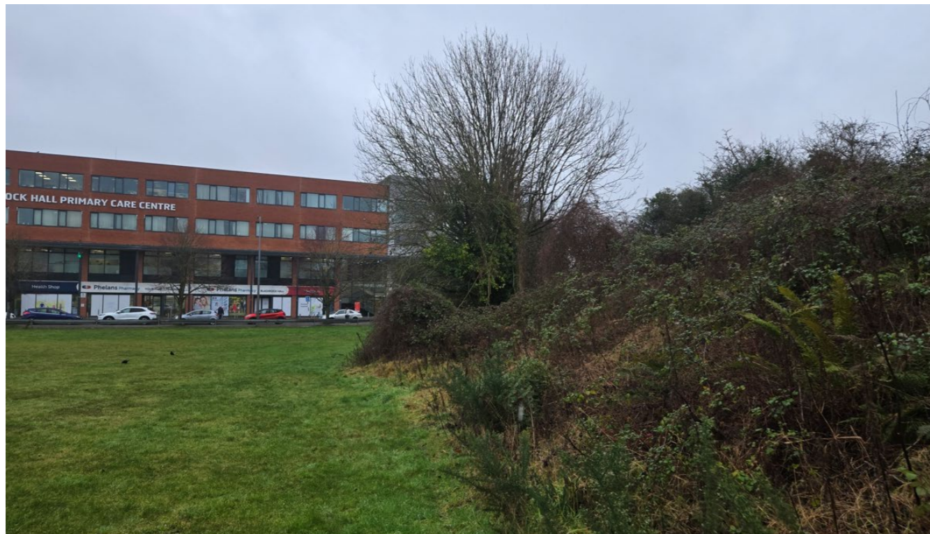
Fig. 3.0 – View eastwards along the southern site boundary; with Blackrock Hall to the east.
