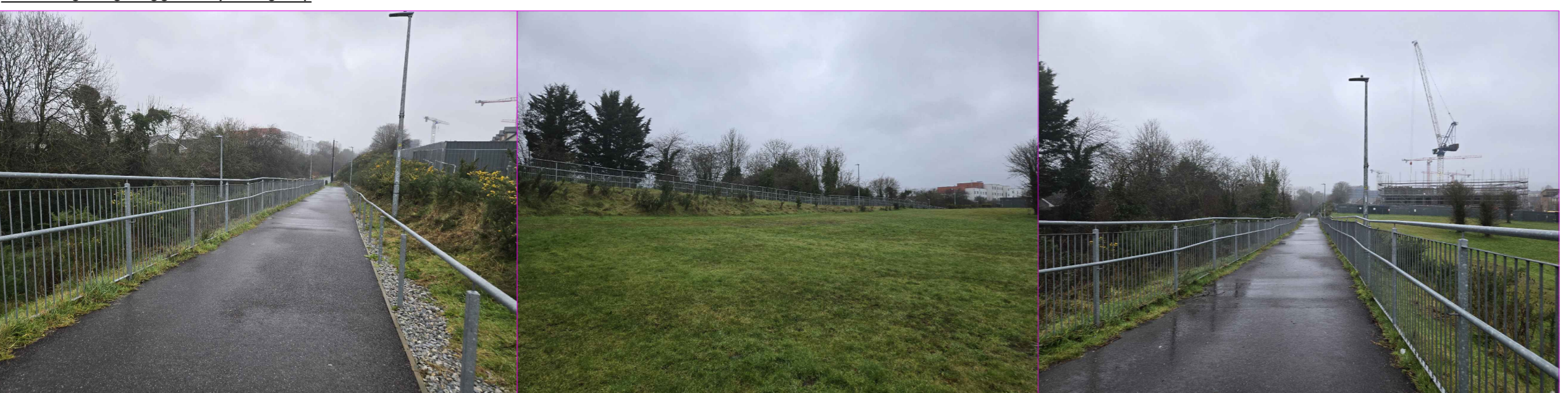
D01 Existing railing along green way walking ramp
