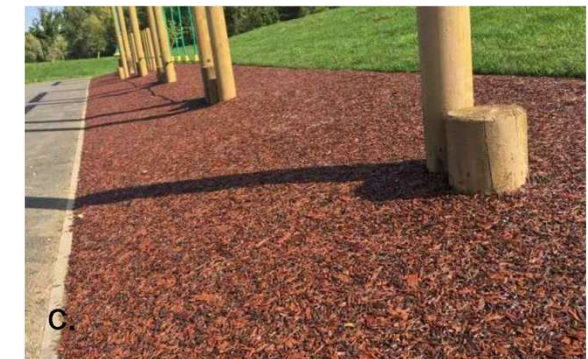
Safe Surfacing Bonded Rubber Mulch to Junior Play Area
