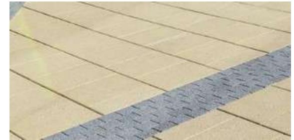
Concrete Paving to Doorways
