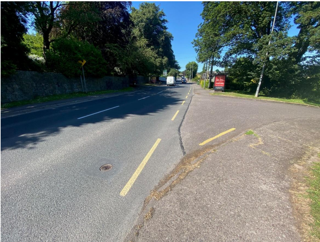
Figure 2.12: Existing Riverside junction.
