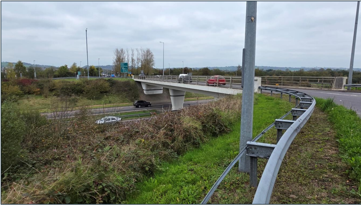
Plate 1-3 - View facing northeast from southern roundabout showing existing bridge.
