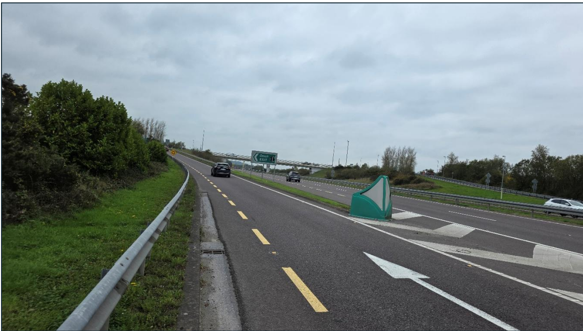
Plate 1-6 - South roundabout off ramp facing west.
