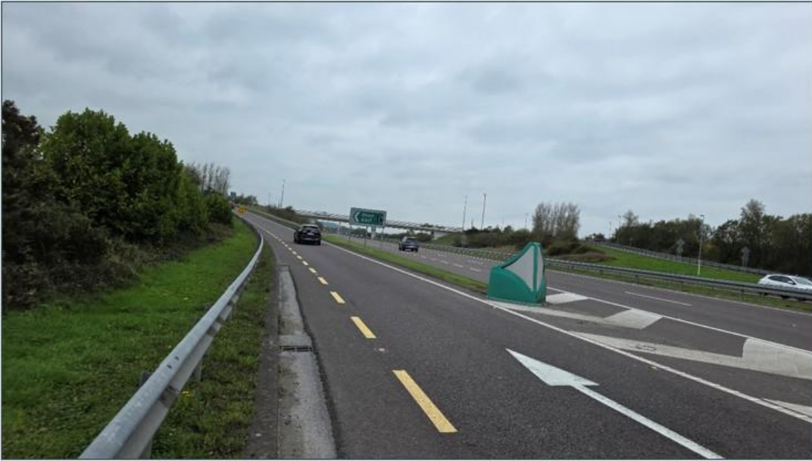
Plate 1-1 - From the N40 facing up the ramp to south roundabout of junction J01.
