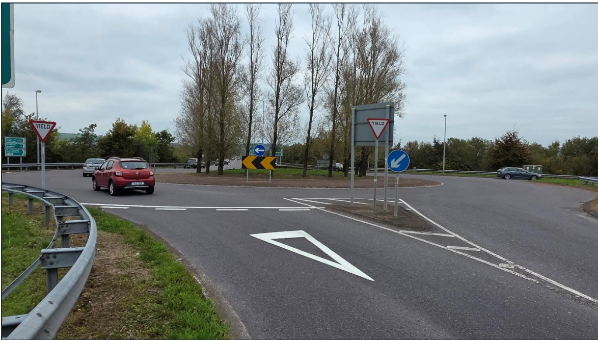
Plate 1-4 - Northern roundabout facing north from existing bridge at J01.
