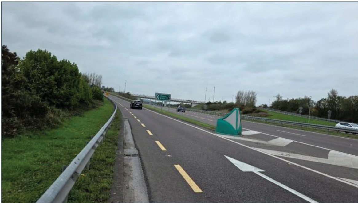
Plate 1 - From the N40 facing up the ramp to junction J01
