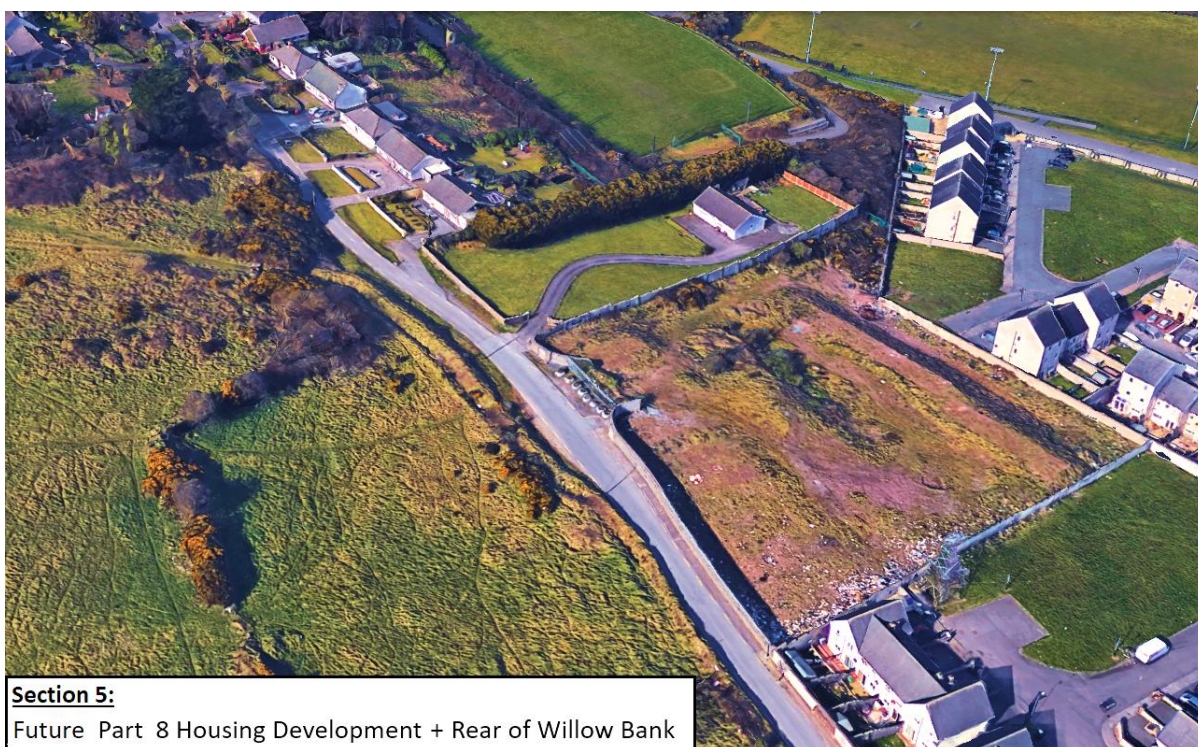
Figure 3-4: Aerial image of Section 5, showing the brownfield site (north of carriageway) planned to house the future Nash's Courtyard Part 8 Housing Development.
