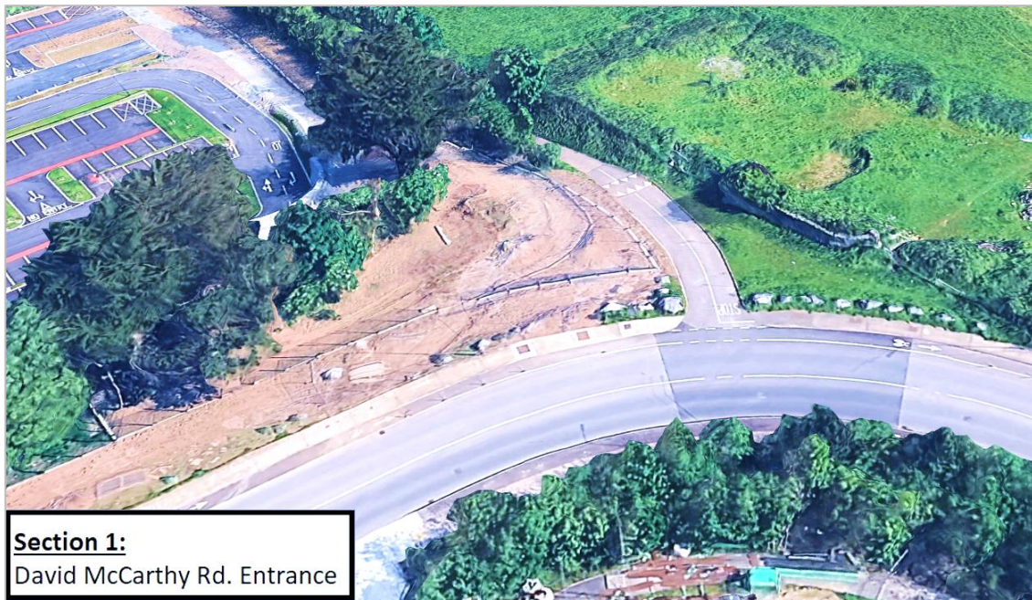
Figure 3-2: Aerial image of the entrance to Section 1 at the David McCarthy Road, showing how heavily sheltered by foliage this segment of the route is.
