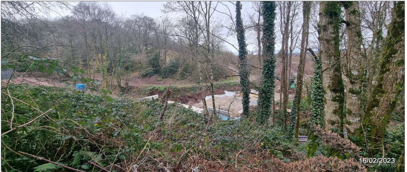
Plate 4.3 Area of proposed works facing west onto the Grange Road to Tramore Valley Park greenway currently under construction [Source: Atkins, 2023].
