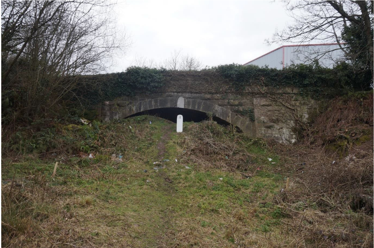
Bridge East elevation
