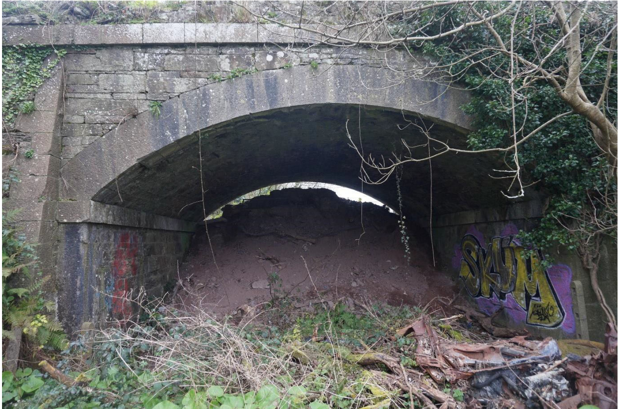
Arch in West elevation with earth mound blocking access
