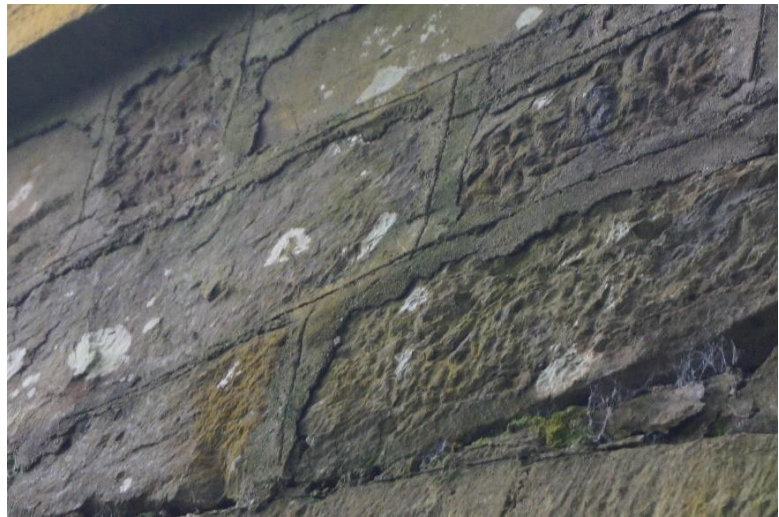
hard cement later mortar repairs with lining to define stone edge
