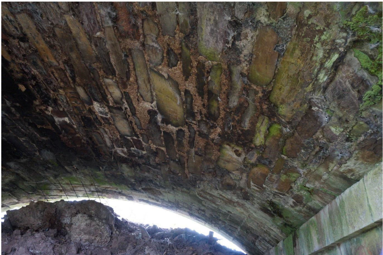
Underside of barrel vault in generally good condition
