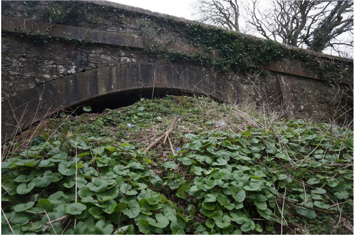
Earth mound concealing East elevation and access through arch
