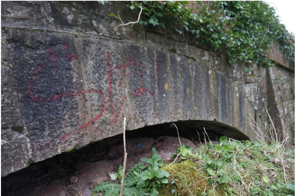
Detail of arch
