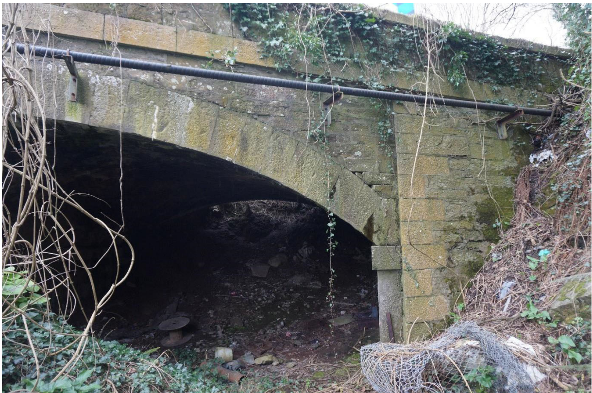
Section of West elevation visible
