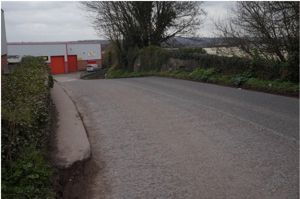
Roadway and bridge parapets looking North
