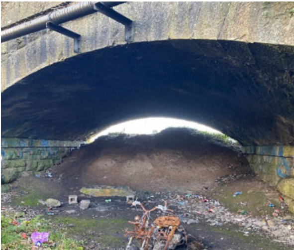
Image 3-5: Earth Mound Beneath Bridge Post
