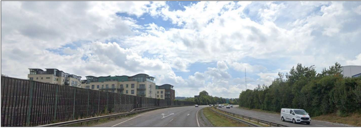
Plate 5.1 View from N25 over estuary at western end of the works area close to Jacob’s Island ((c) Google Earth).
