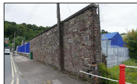
Figure 6-6 – Existing Stone Wall at McMahons Builders Providers Yard
