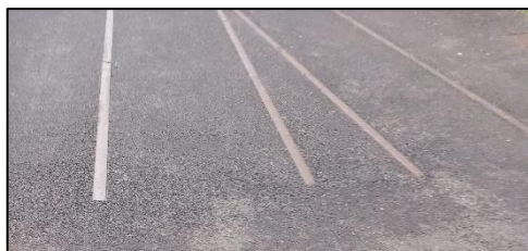
Figure 6-2 – Example of rails treatment at Blackrock, Cork
