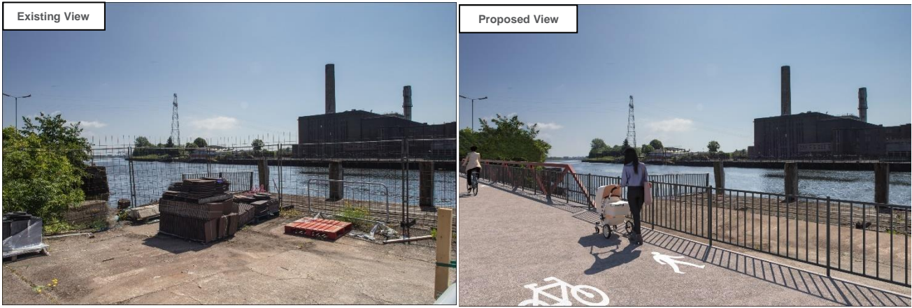
Figure 3-7 – Option A Photomontage: Before and After View at Dry Dock Crossing within McMahons Builder Providers
