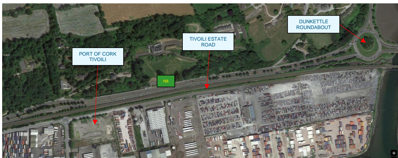
Figure 5-4 - Existing Infrastructure along the Dual Carriageway up to the Dunkettle Roundabout
