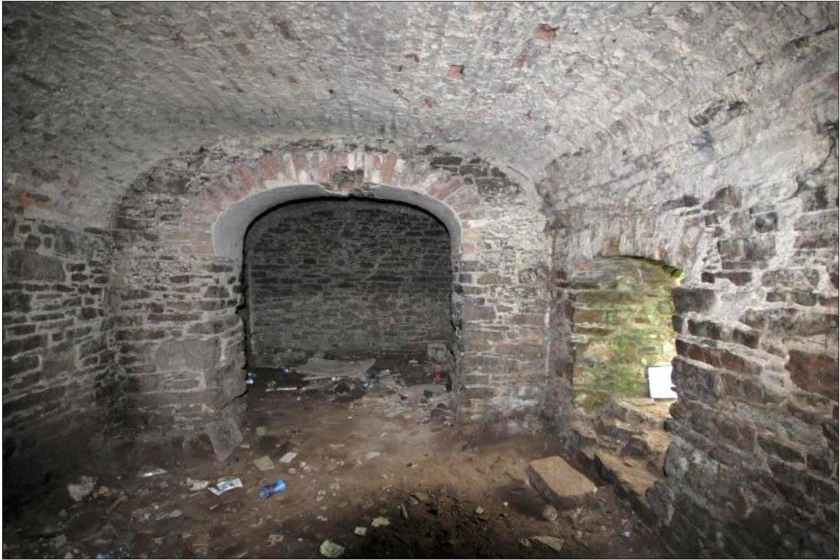
Plate 11: Lower ground floor level LGF01 looking west
