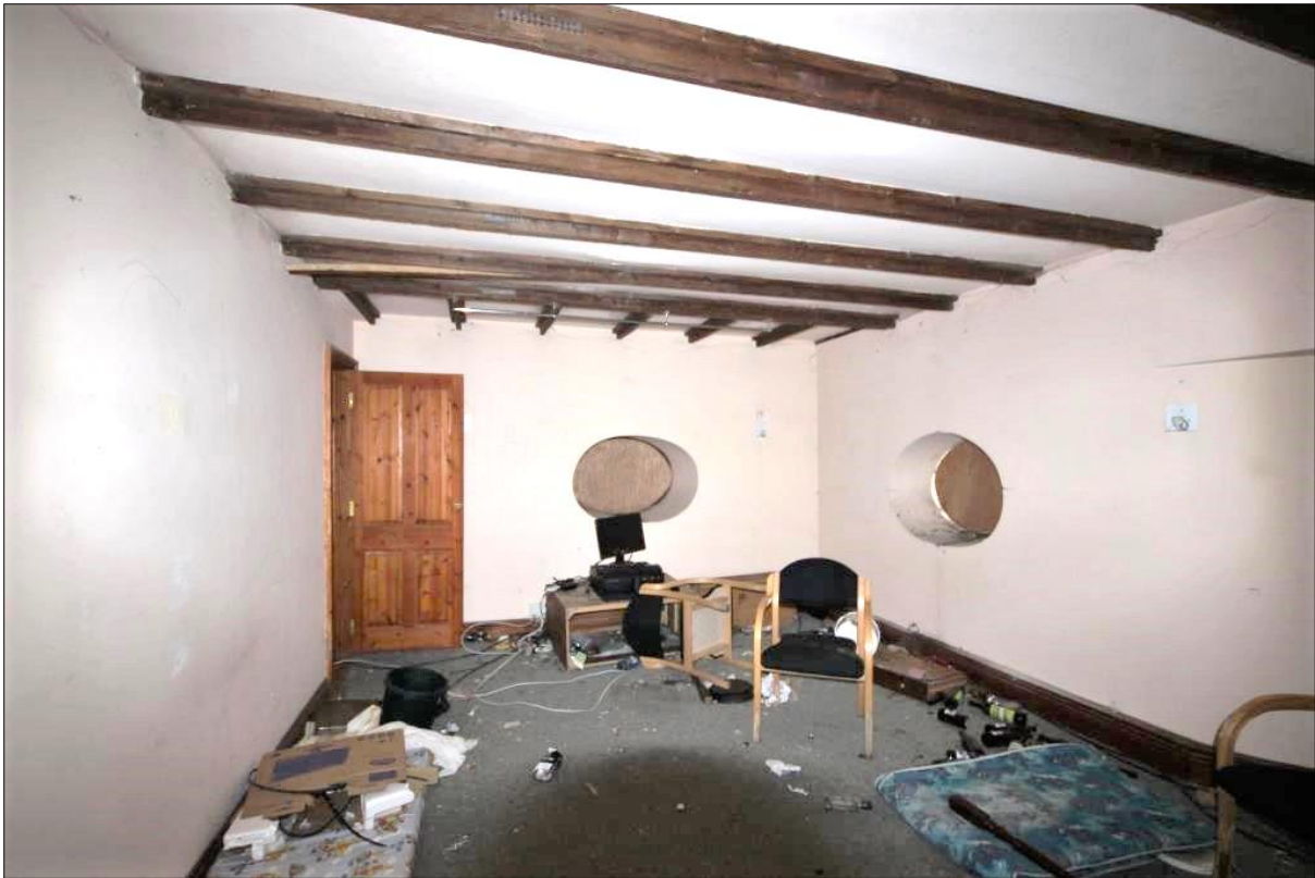
Plate 23: First floor room FF04
