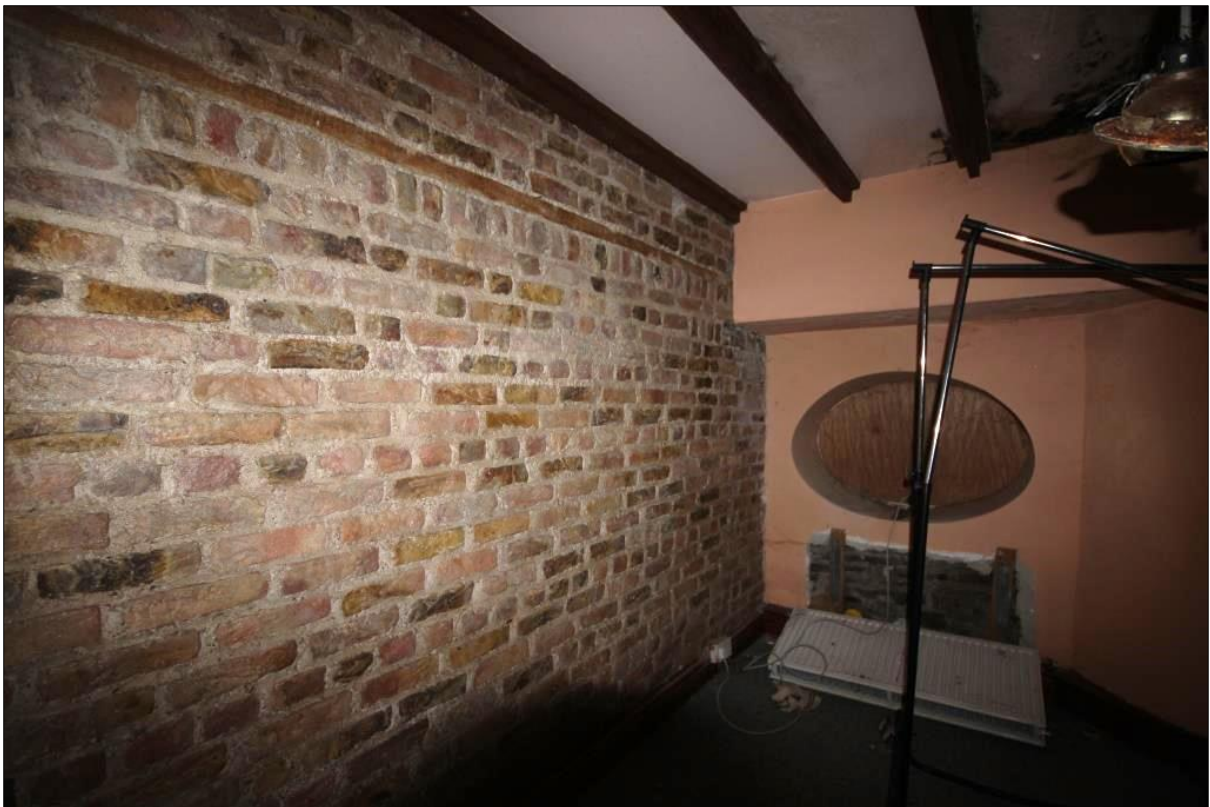
Plate 26: Original brick wall and oculus in FF06
