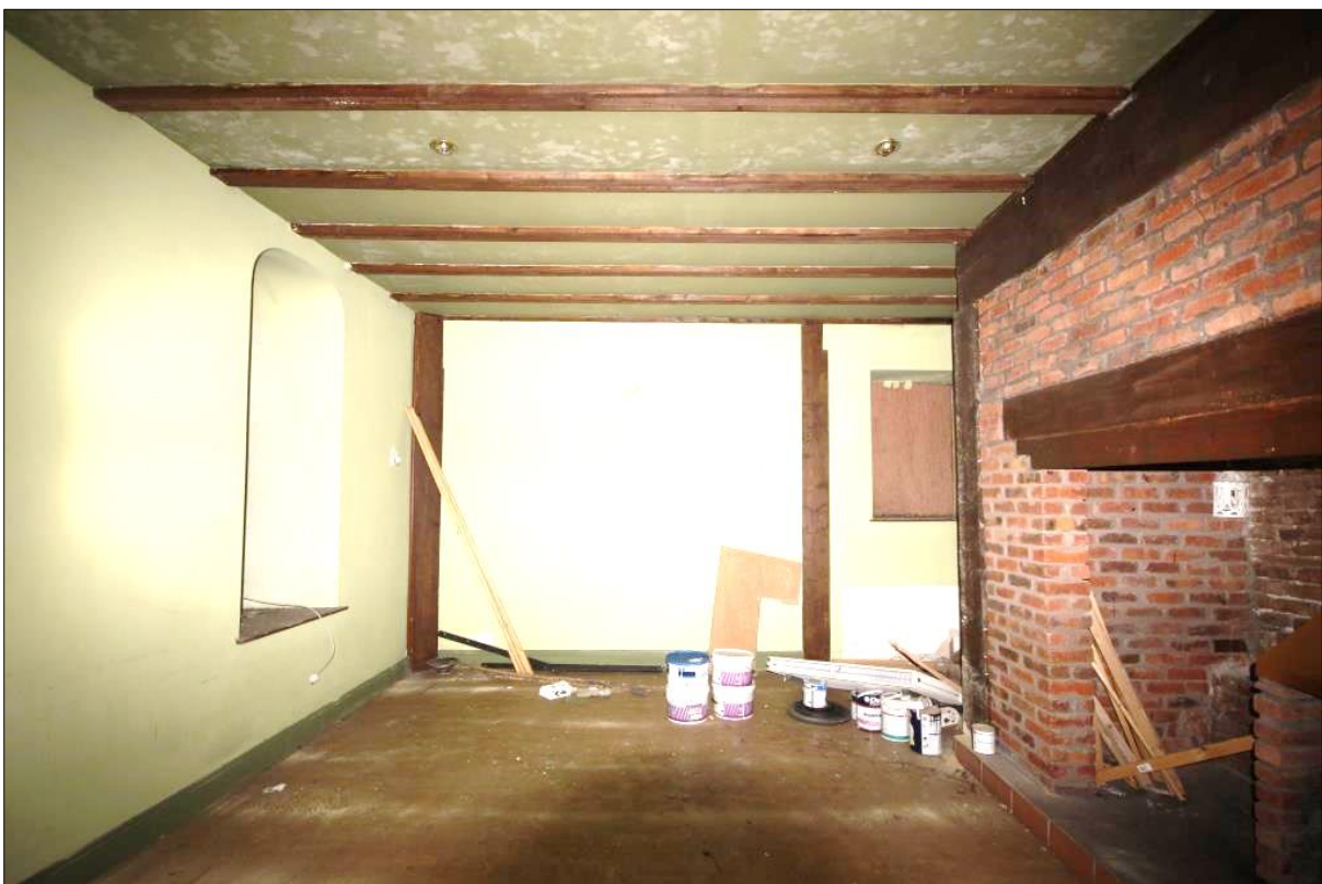
Plate 16: Ground floor room GF02 looking to rear
