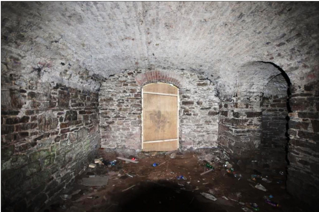
Plate 10: Lower ground floor level LGF01 looking east
