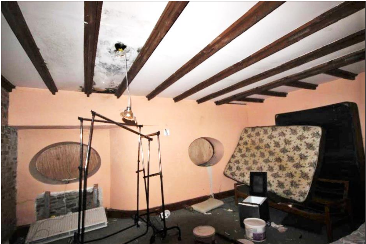
Plate 25: First floor room FF06
