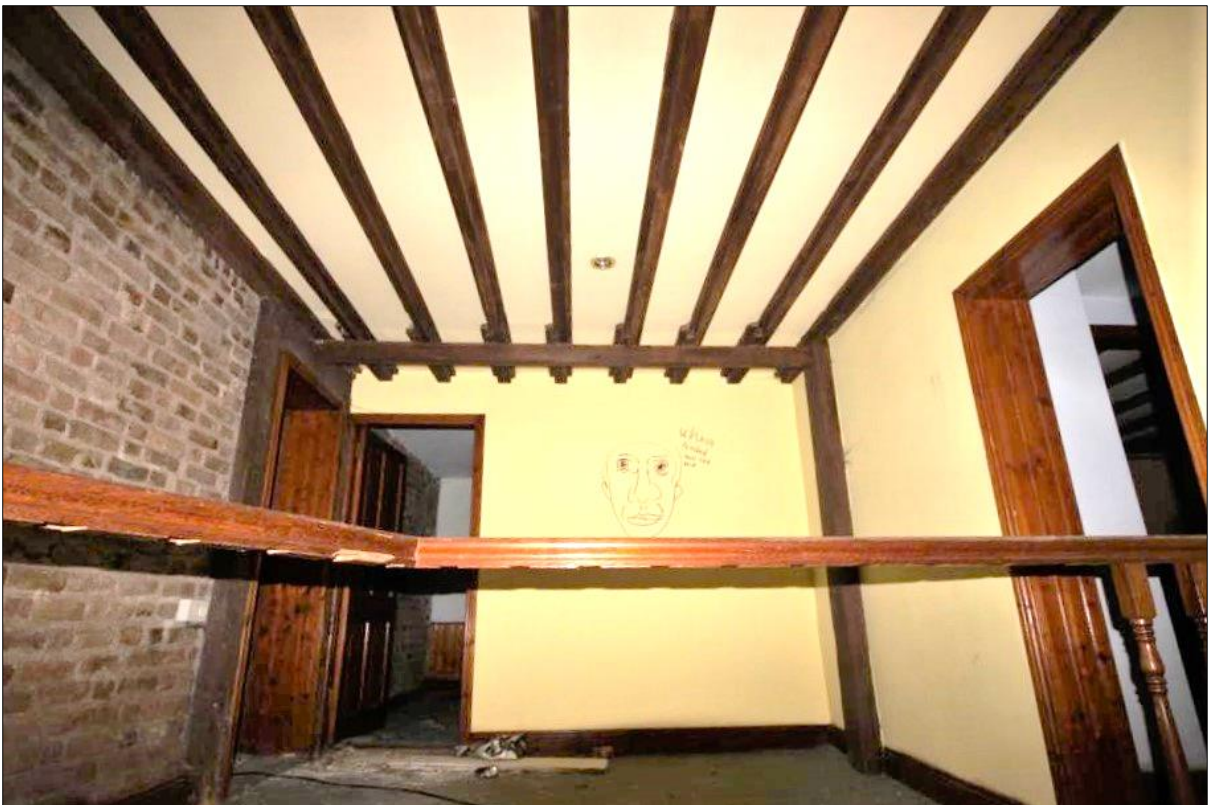
Plate 22: First floor landing FF01 looking to front
