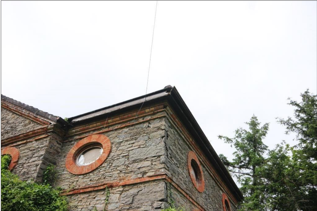
Plate 9: Detail of south-eastern corner
