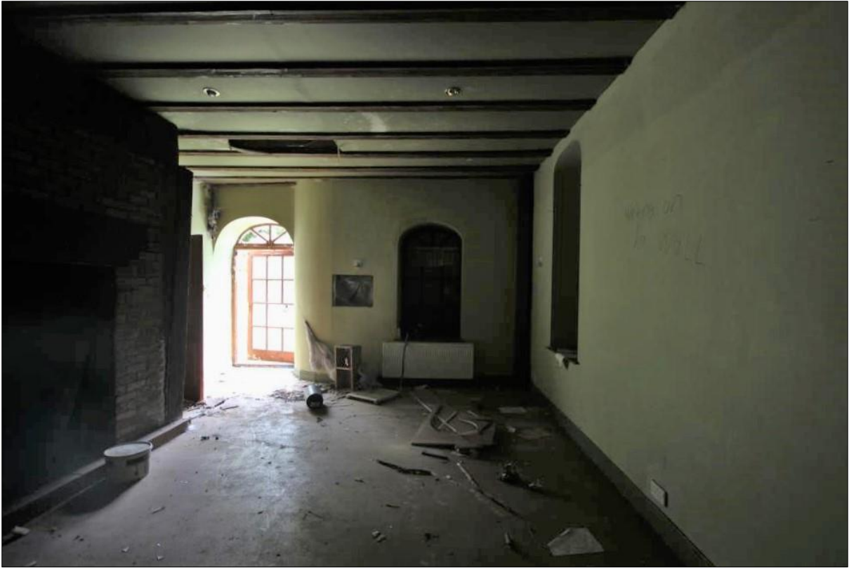
Plate 19: Ground floor room GF02 looking to front
