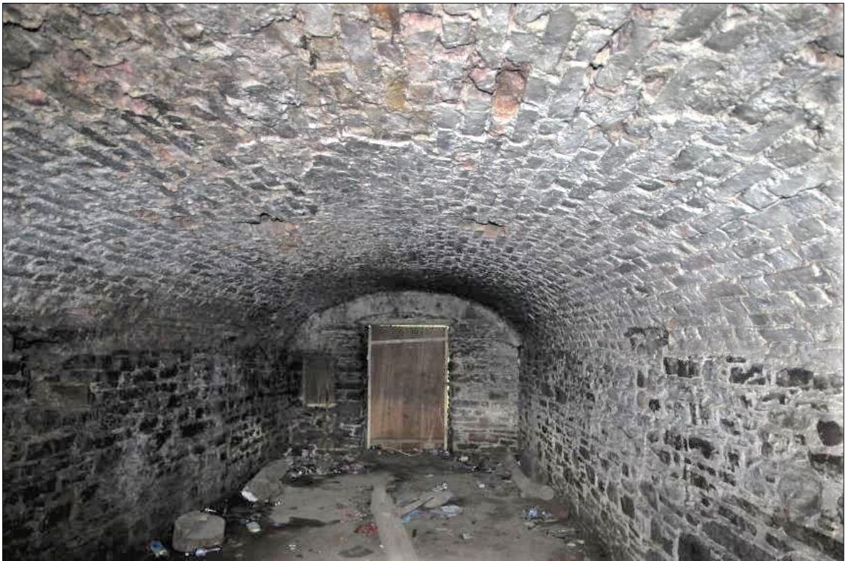
Plate 12: Lower ground floor level LGF03 looking west
