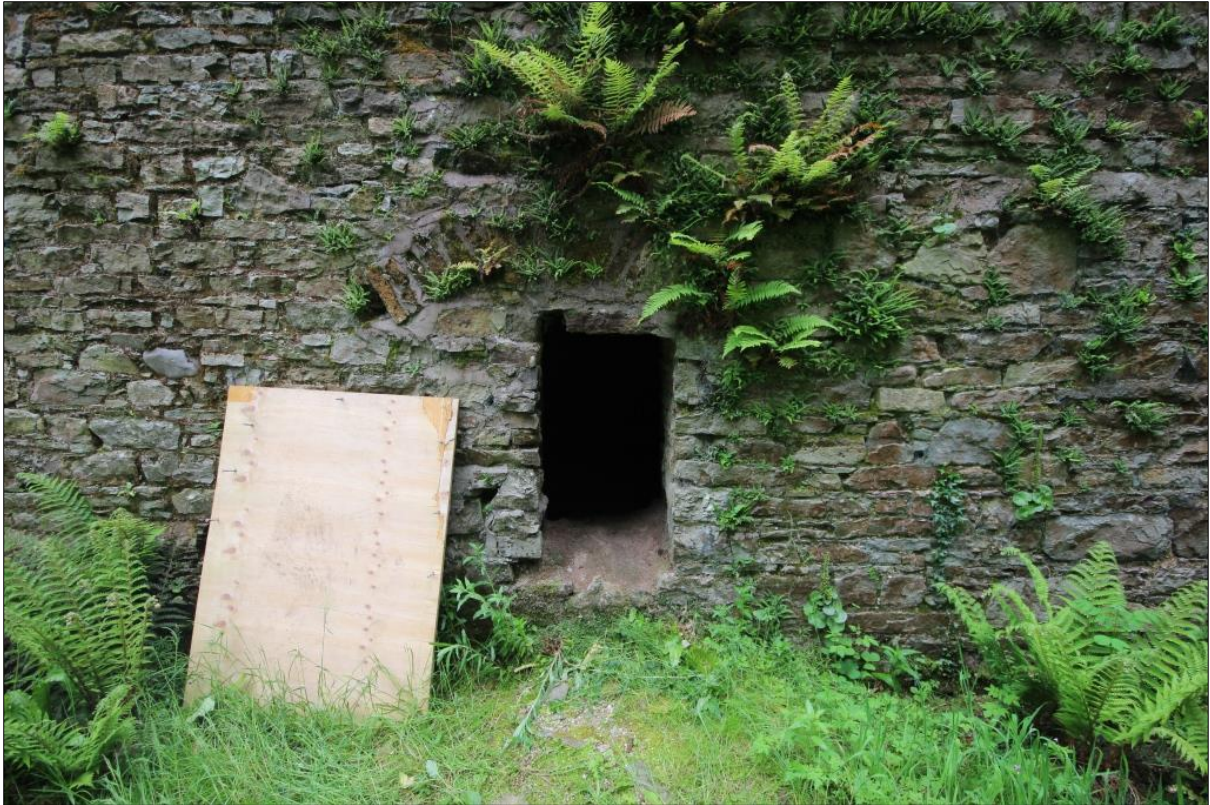
Plate 7: Opening in lower ground floor of northern elevation
