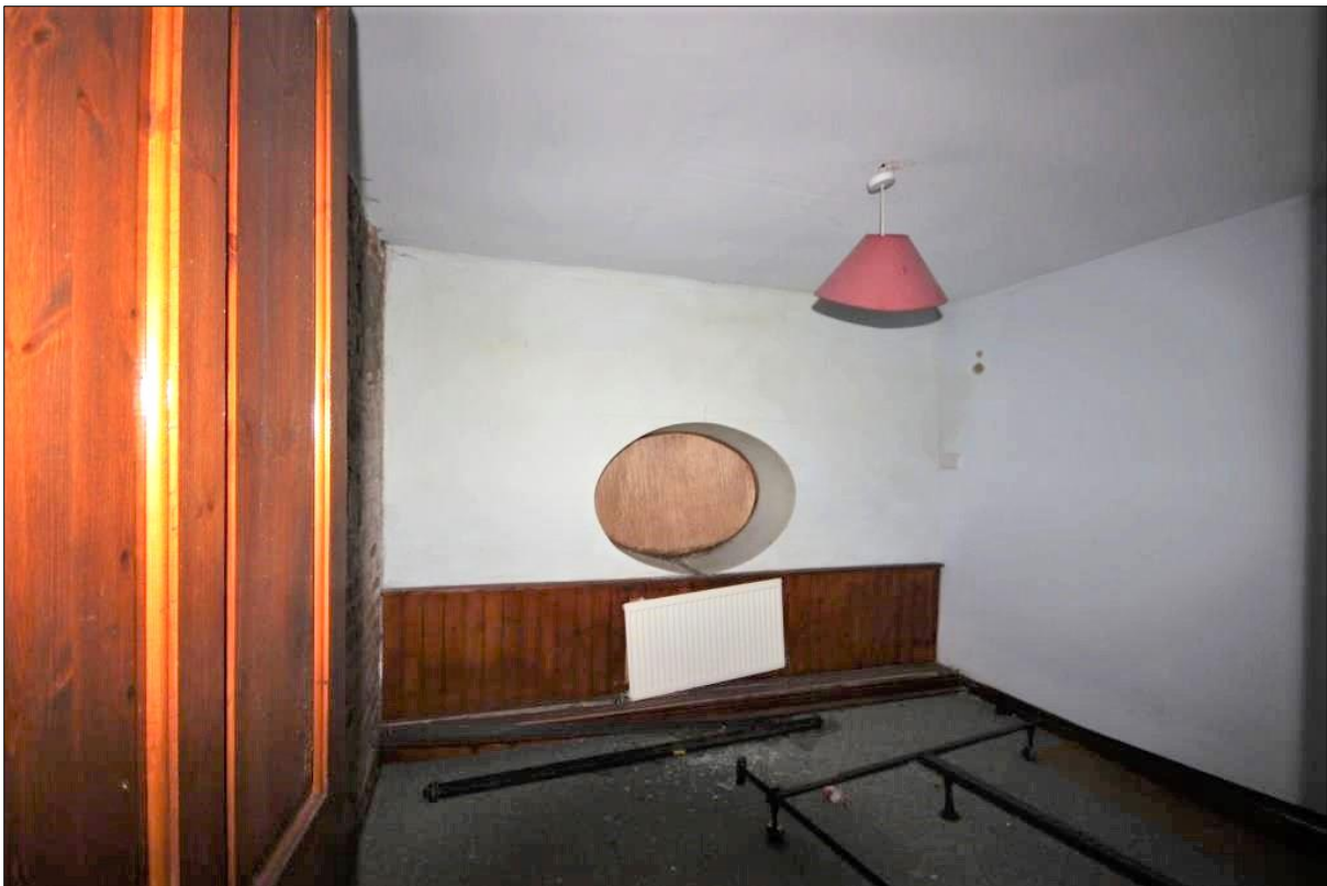
Plate 24: First floor room FF05
