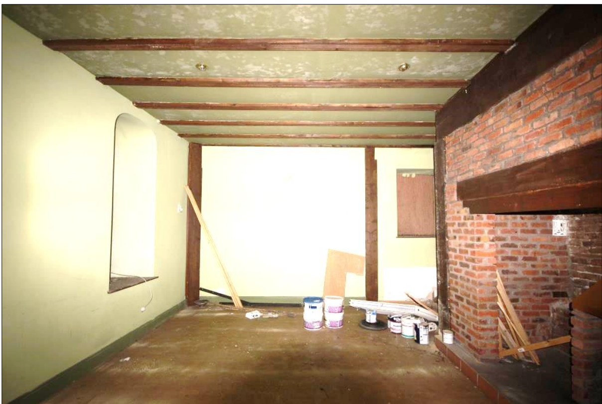
Plate 16: Ground floor room GF02 looking to rear
