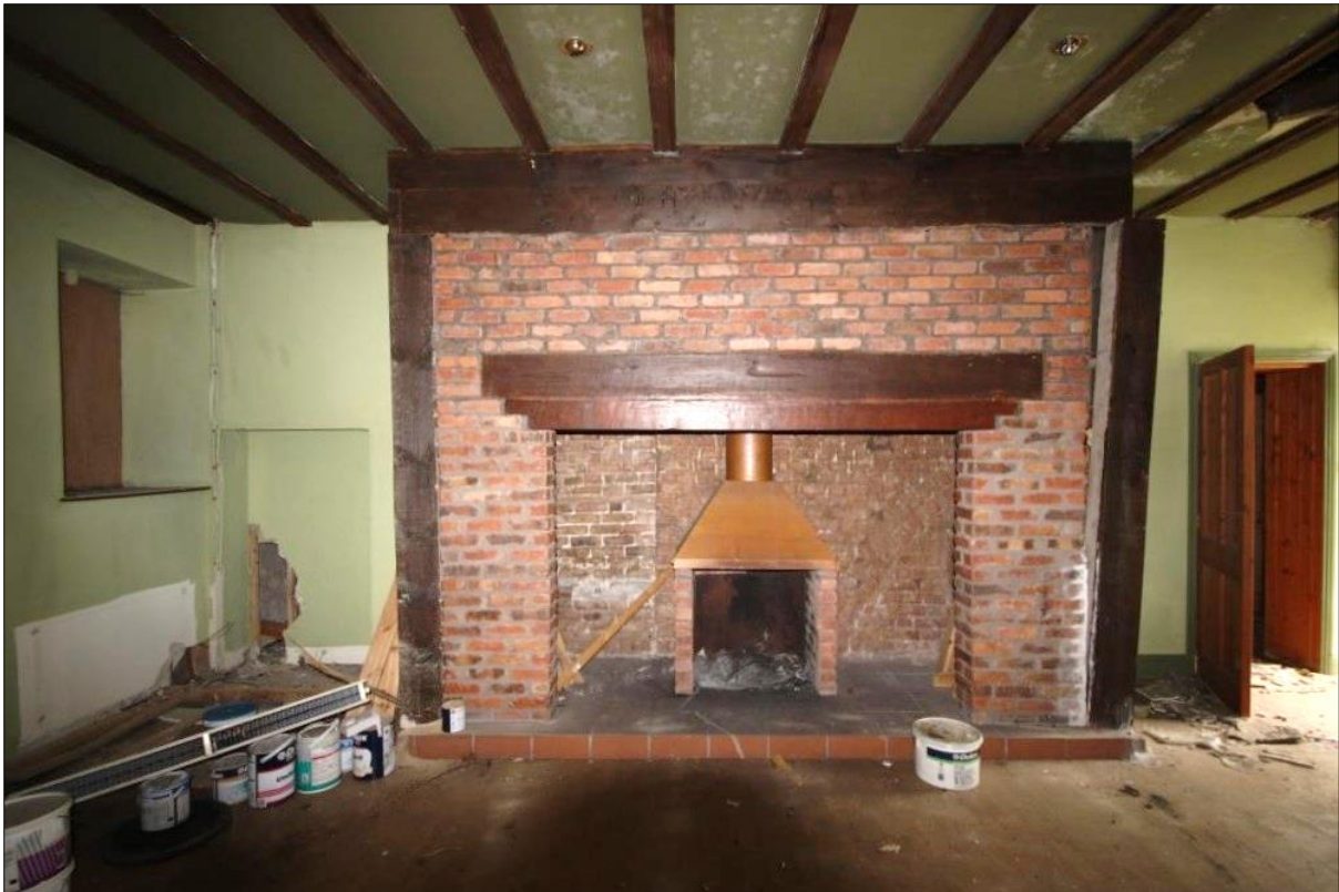
Plate 17: Modern brick fireplace built up against original brick wall in GF02
