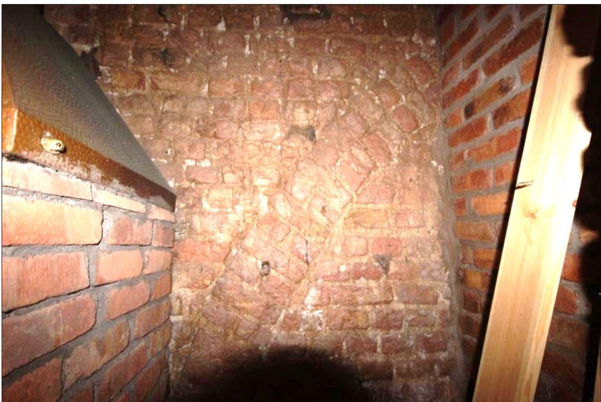
Plate 18: Relieving arch detail in original wall GF02
