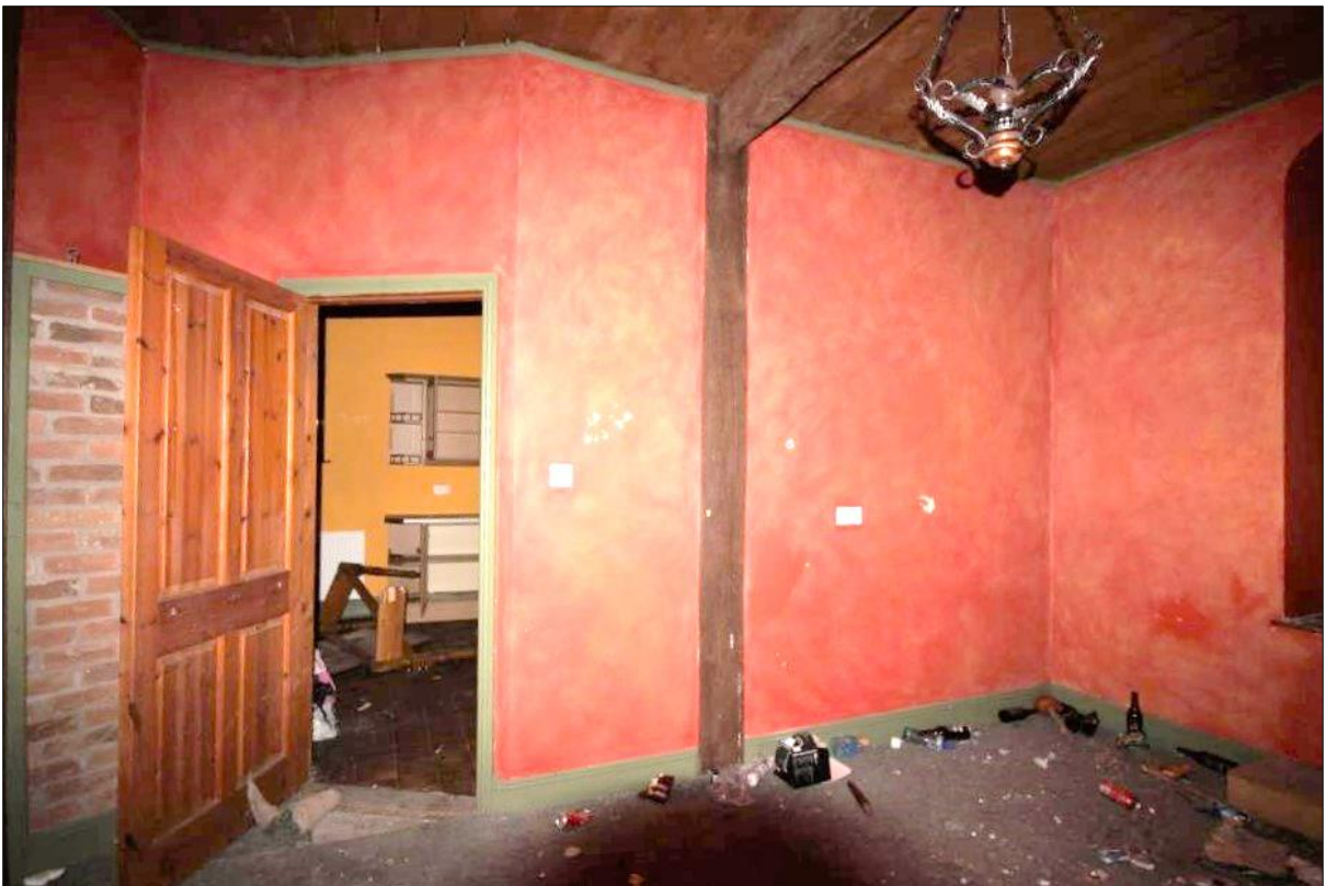
Plate 20: Ground floor room GF03 looking to GF04
