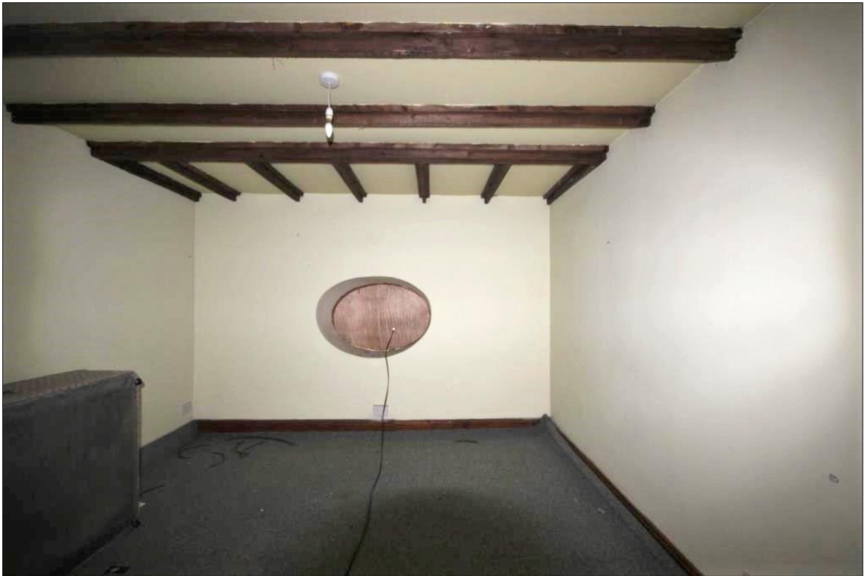
Plate 27: First floor room FF07
