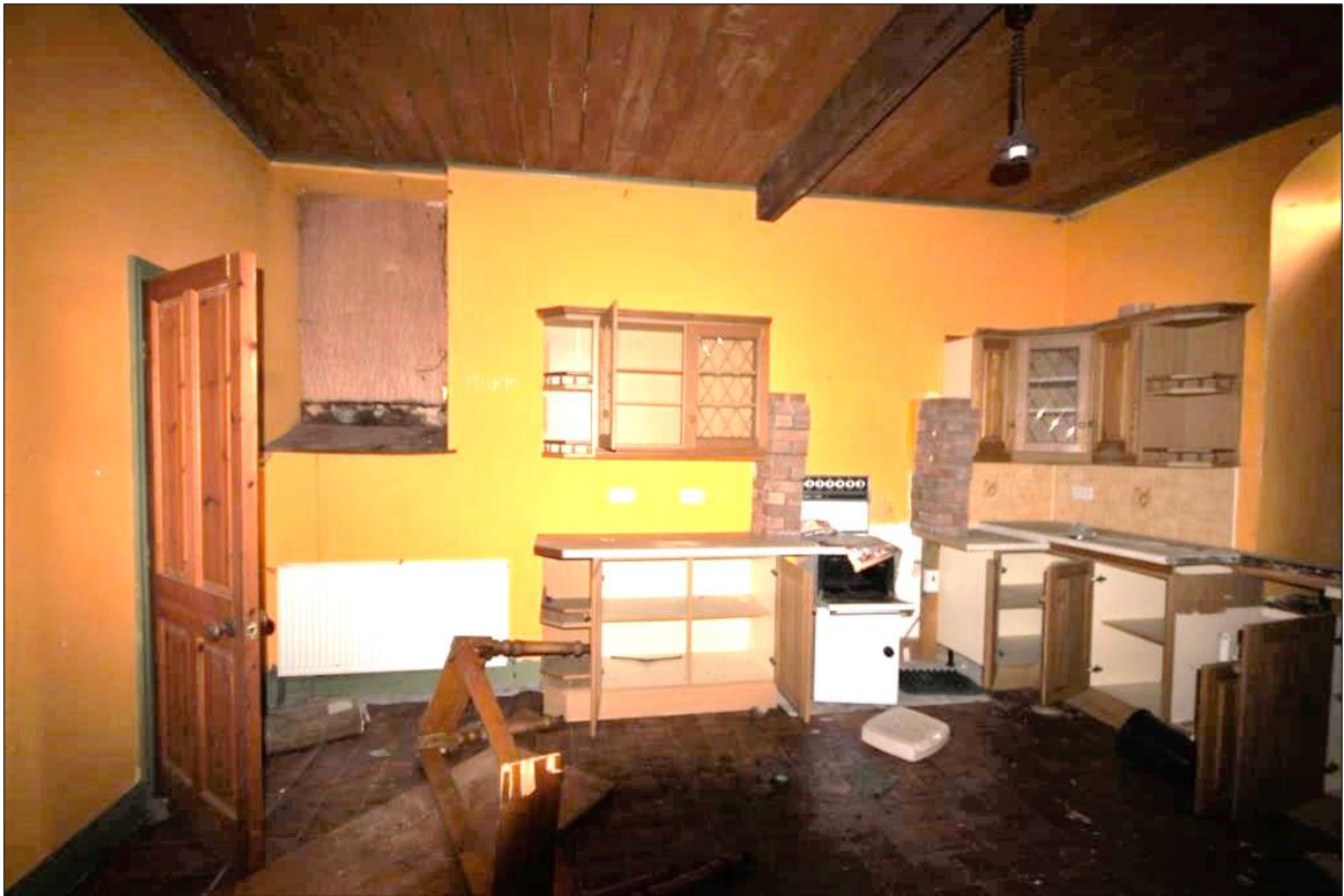
Plate 21: Ground floor room GF04
