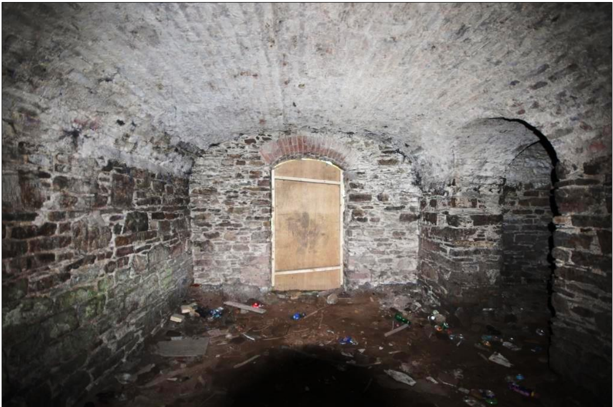
Plate 10: Lower ground floor level LGF01 looking east
