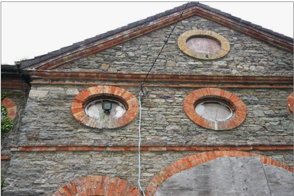
Plate 8: Detail of windows to first floor level on front elevation
