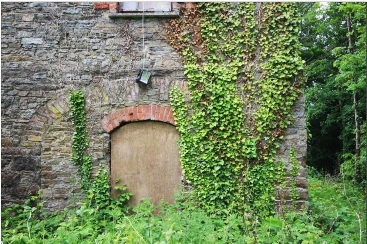
Plate 6: Opening in lower ground floor of eastern elevation
