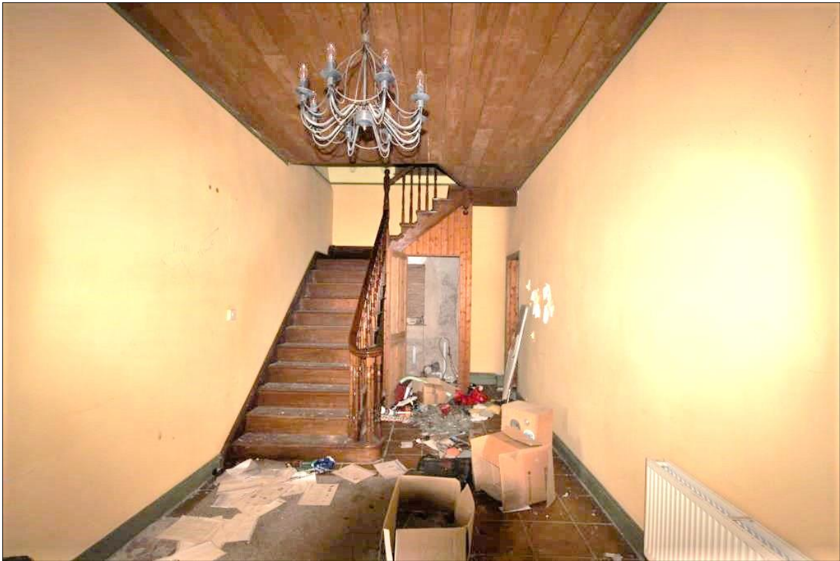
Plate 15: Ground floor entrance hall GF01 looking to rear
