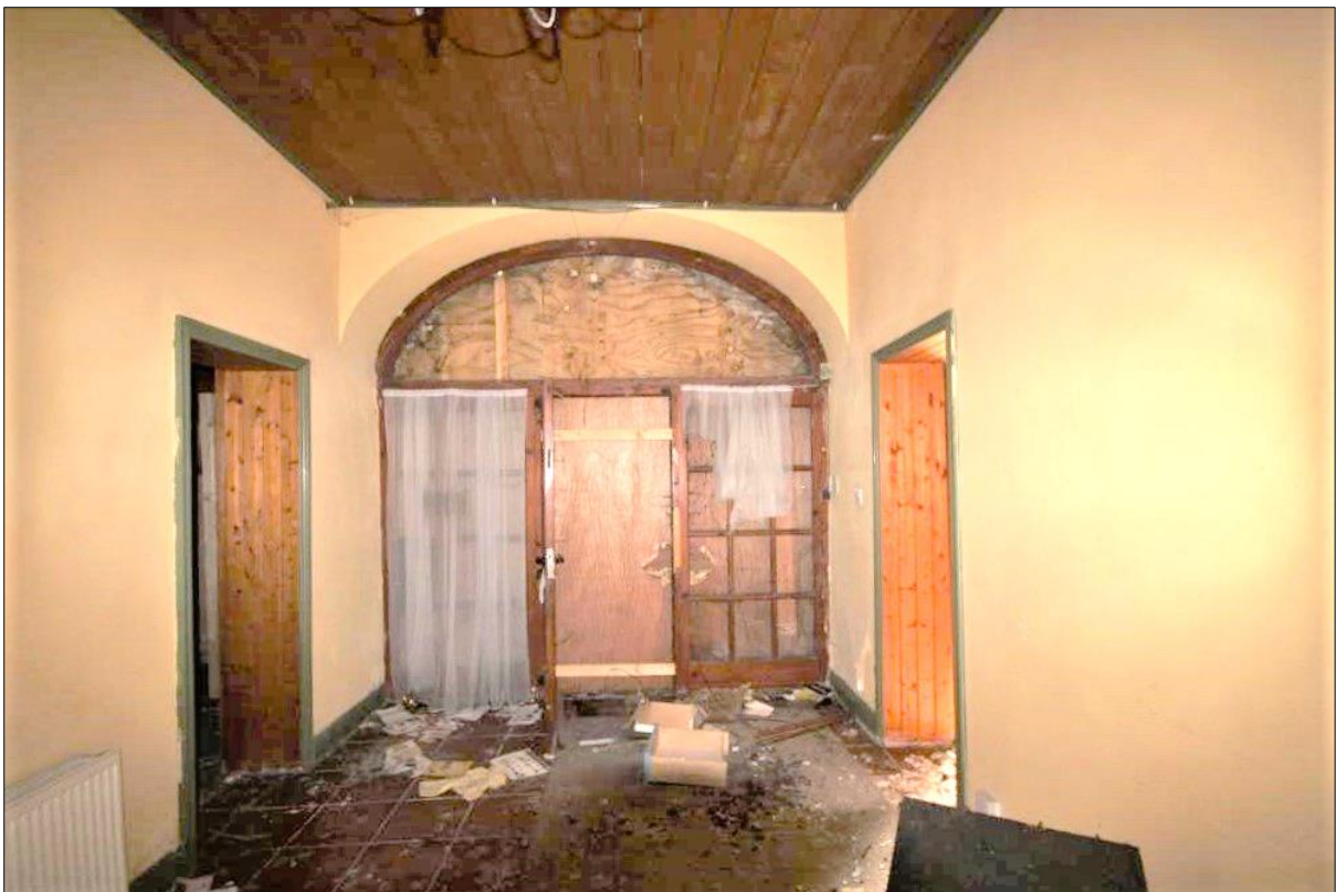
Plate 14: Ground floor entrance hall GF01 looking to front
