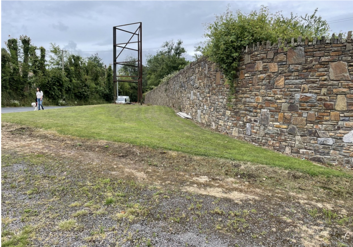
Photo A2 Site boundary along the nearside road edge, looking south.
