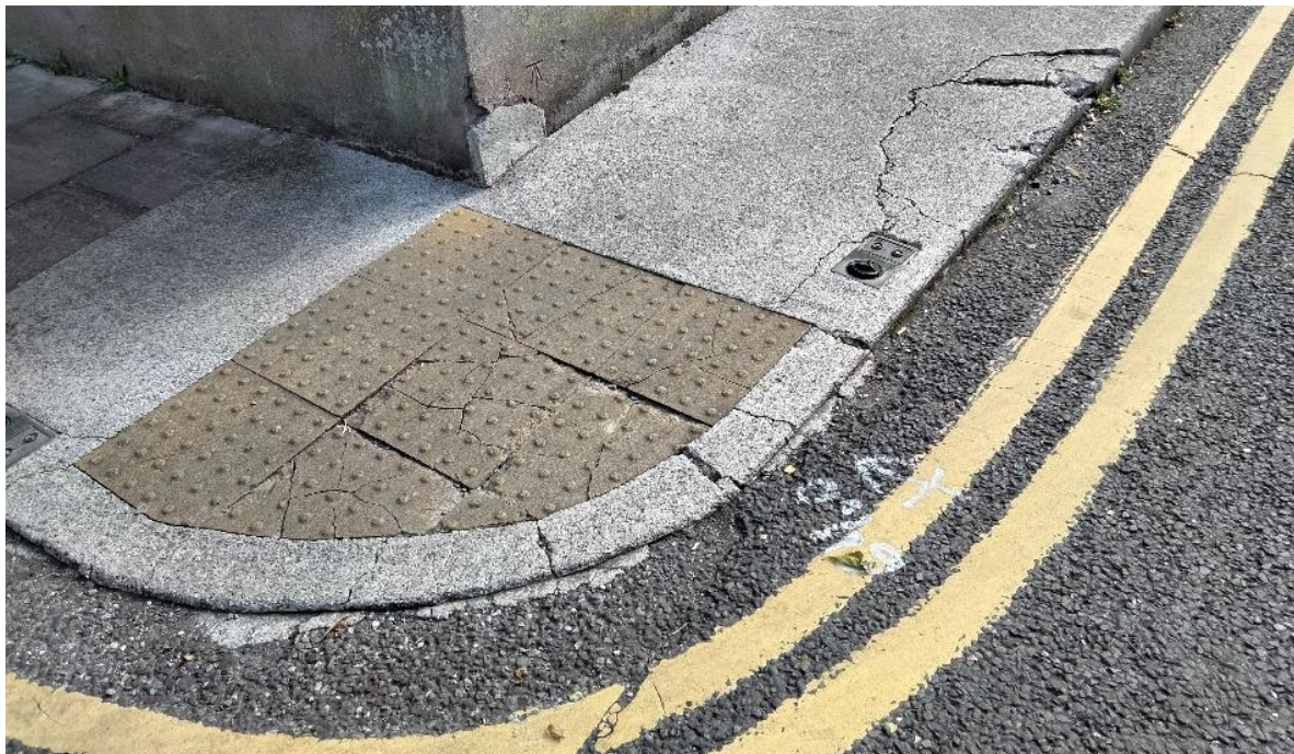
Figure 1-3: Footpath Damage due to Vehicle Overrunning (Corner of Douglas Street and White Street)
