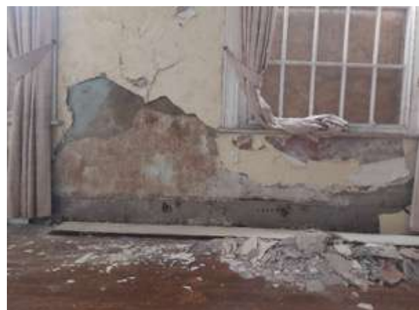
Fig.143: Removed skirting from damp wall (EXG-02)
