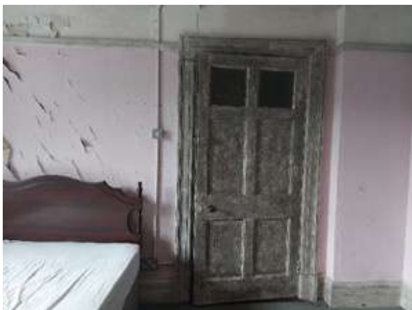
Fig.121: Mould build up on timber door (EXG-05)
