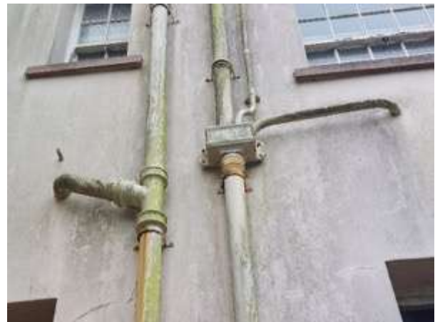
Fig.21: Algae build up on north elevation rainwater goods
