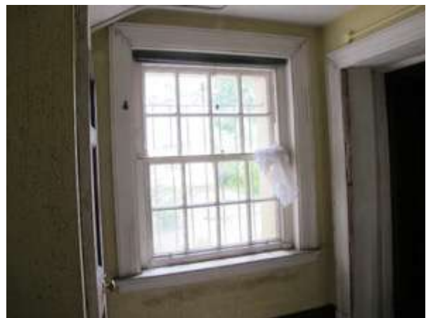
Fig.127: Painted timber ogee horned eight-over-eight sash frame (EXG-13)
