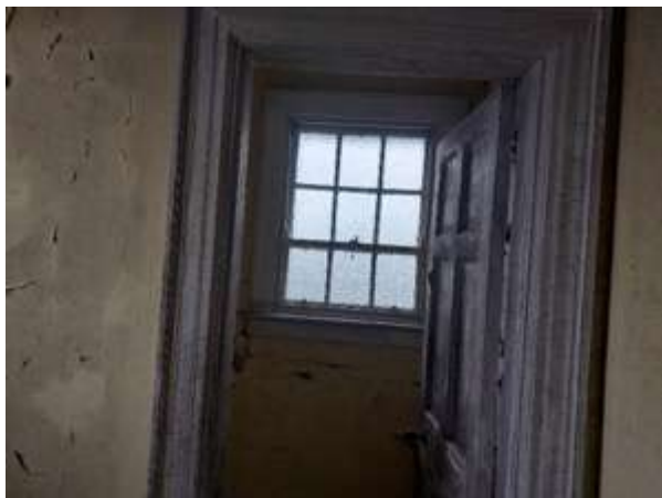
Fig.146: Mould build up and paint damage to timber architrave (EX2-03)
