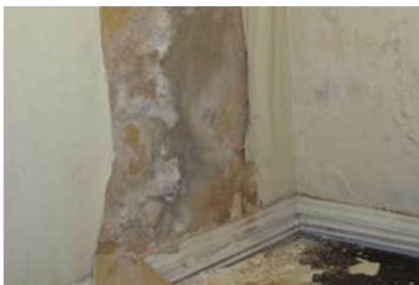
Fig.142: Efflorescence damaging timber skirting (EXG-15)
