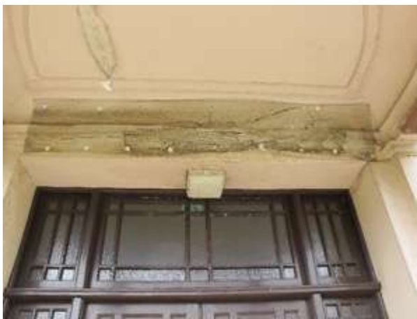
Fig.44: Damage to ceiling currently secured with mesh
