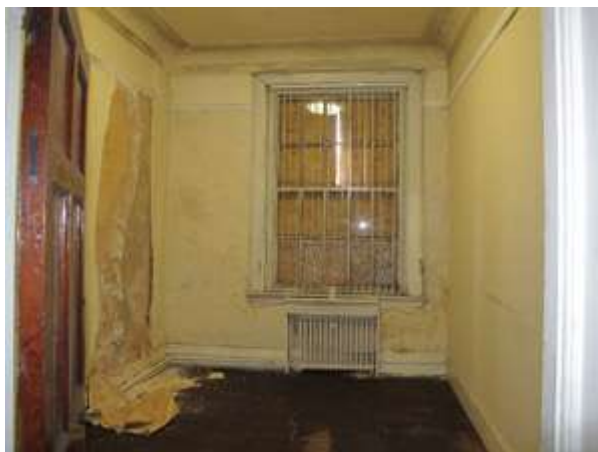
Fig.126: Painted timber ogee horned ten-over-ten sash frame (EXG-15)
