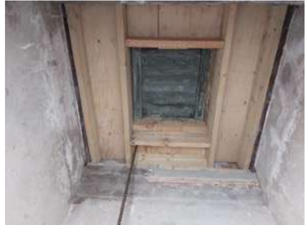
Fig.55: Repairs to platform to final stage. Bell rope remains in situ. Note leaching and efflorescence to walls at high level
