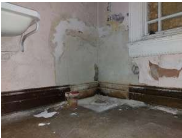
Fig.183: Signs of water ingress and previous repair to wall adjacent to timber frame (EXG-29)
