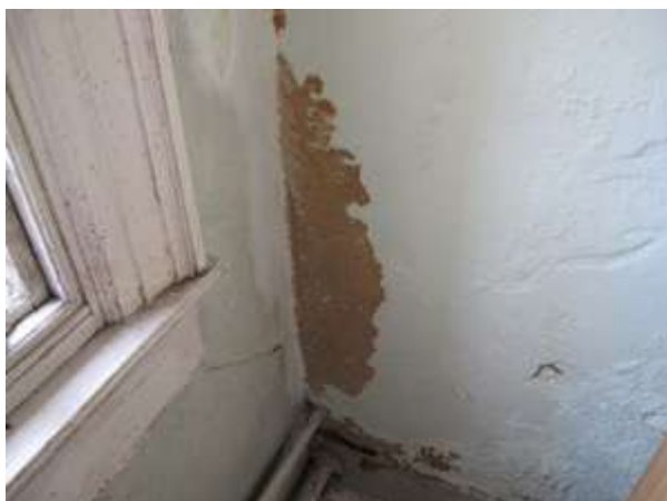
Fig.102: Fungus to second floor wall (EX2-19)
