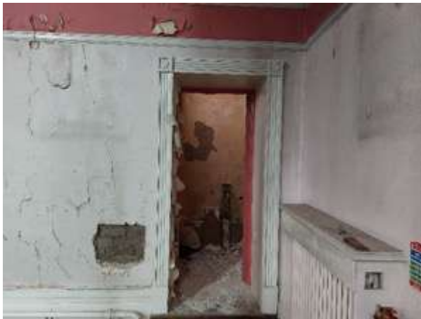
Fig.185: Timber architrave to door in nave
