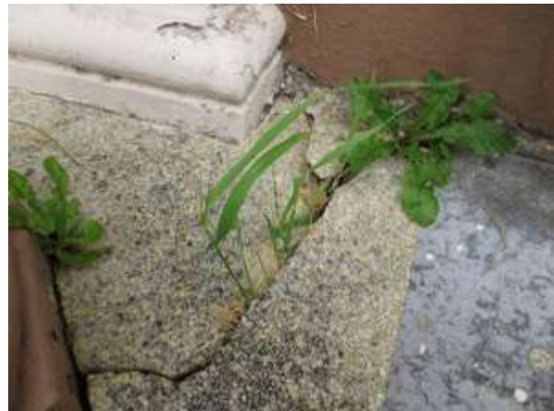
Fig.47: Plant growth in cracked terrazzo
