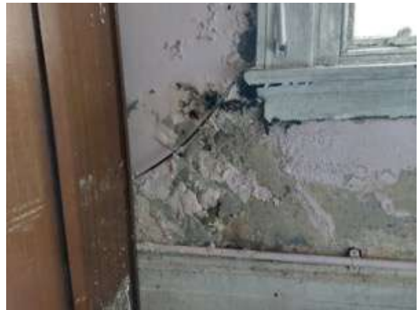
Fig.139: Mould build up around timber sill (EXG-05)
