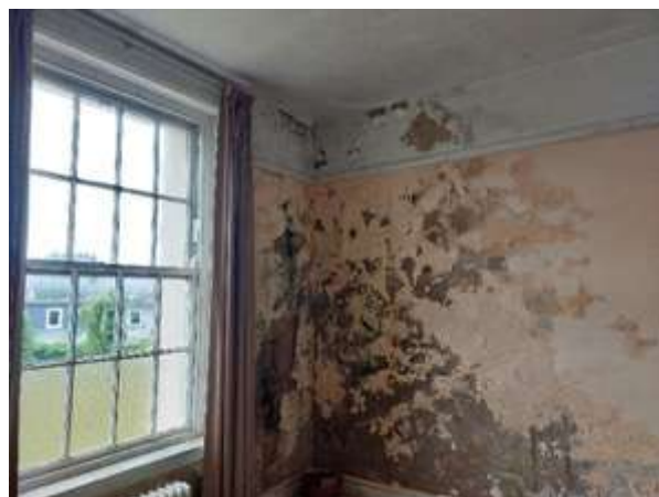
Fig.103: Efflorescence and damp on wall (EX1-23)
