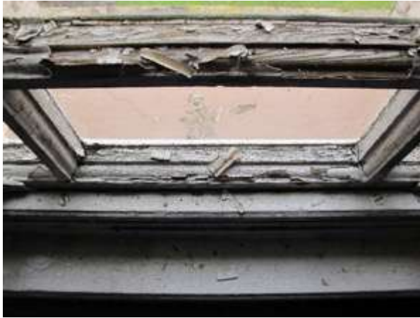
Fig.136: Peeling paint to timber glazing bar (EX2-17)
