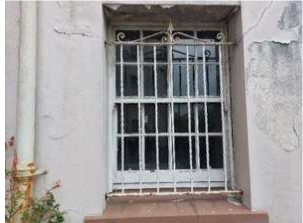
Fig.36: Paint flaking and cracking to north elevation window surround, note decoratively-detailed iron guarding
