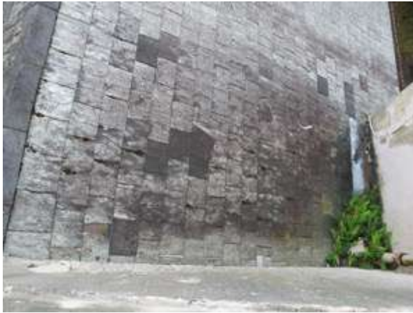
Fig.77: Plant life blocking drainage
