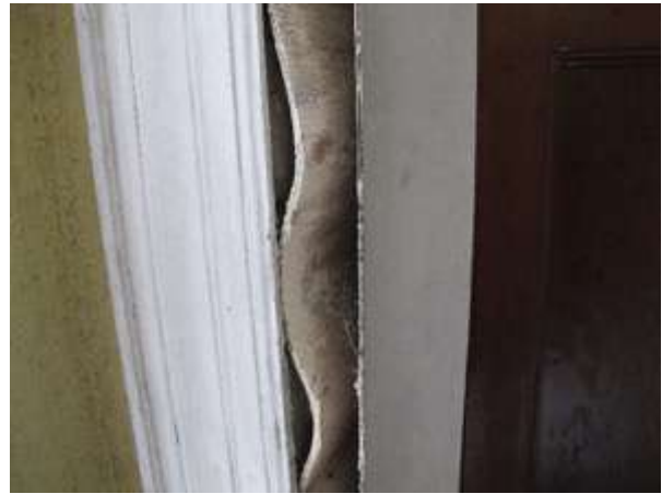
Fig.124: Disintegration of timber door frame (EXG-10)
