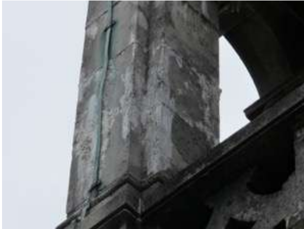
Fig.54: Leached deposits to final stage. Note lightning conductor
