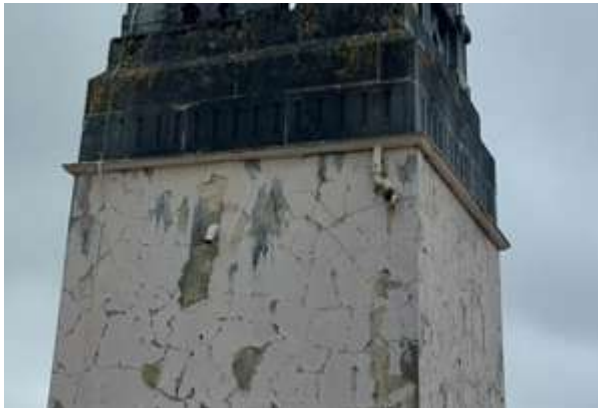
Fig.56: Gutter to bell tower, note missing downpipe
