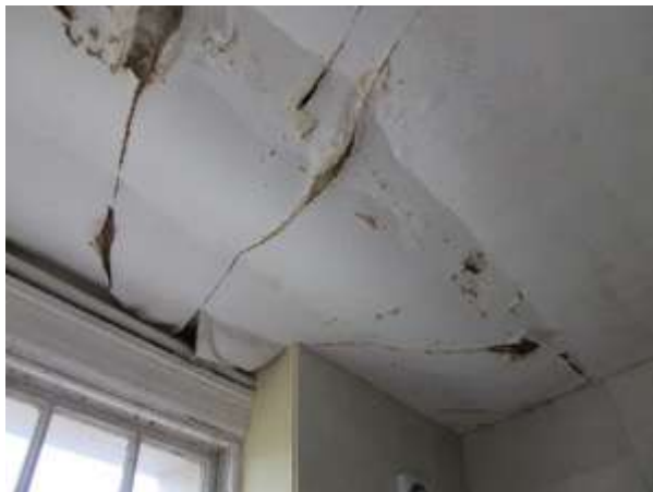
Fig.96: Ceiling sagging and cracking (EX2-10)
