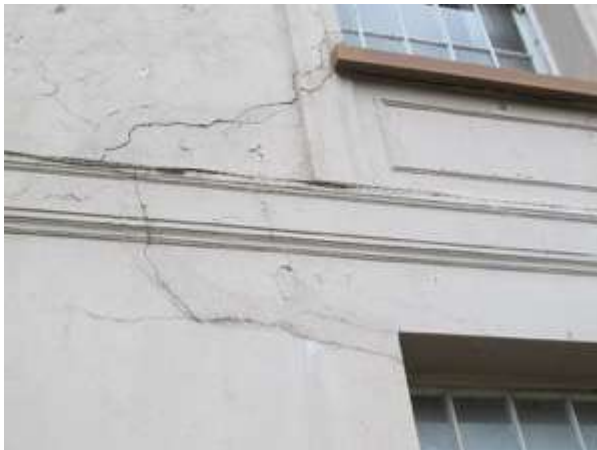
Fig.27: Cracking on south elevation
