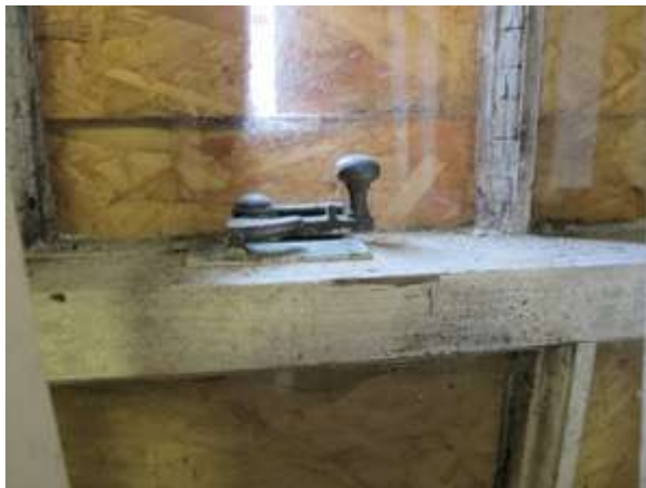
Fig.130: Close up of working features of sliding sash (EXG-16)
