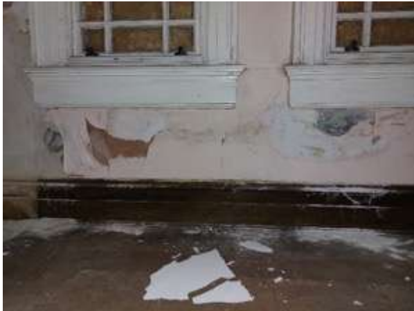
Fig.167: Water ingress and damage to sacristy east wall (EXG-29)
