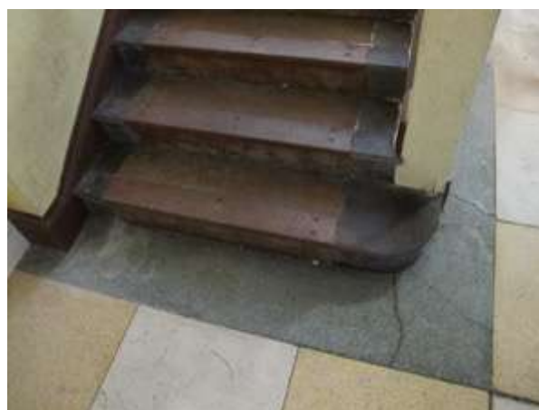
Fig.110: Cracking to ground floor flooring at east staircase (EXG-13)
