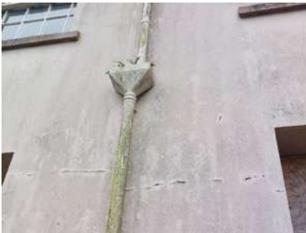
Fig.22: Plant growth in hopper
