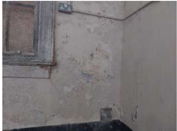
Fig.145: Mould build up to window surround (EXG-19)
