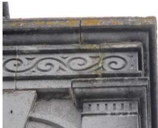
Fig.53: Open joints and cracking to final stage
