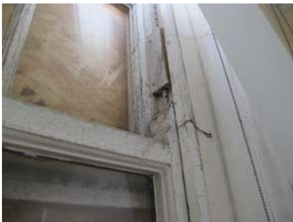
Fig.128: Close up of working features of sliding sash (EXG-16)
