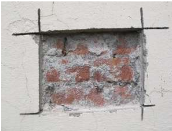
Fig.26: Incision of wall on south elevation
