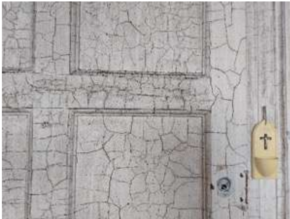
Fig.123: Damaged paint of timber six-panelled door (room EX1-20)
