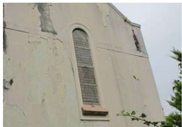
Fig.86: Wire-guard over large stained glass window
