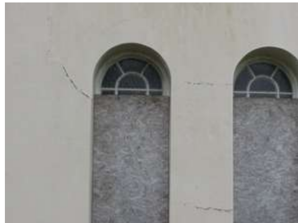
Fig.82: Cracks to render on east elevation
