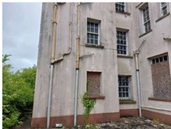
Fig.18: Mix of modern plastic and cast iron down pipes on north elevation
