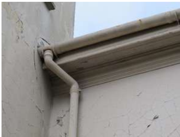
Fig.75: Gutter and down pipe on south elevation
