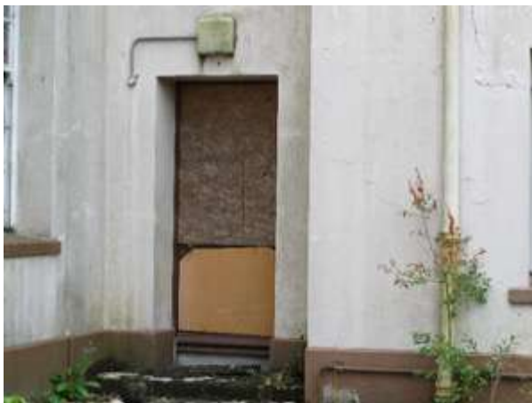
Fig.40: Plywood affixed to door to northwest return
