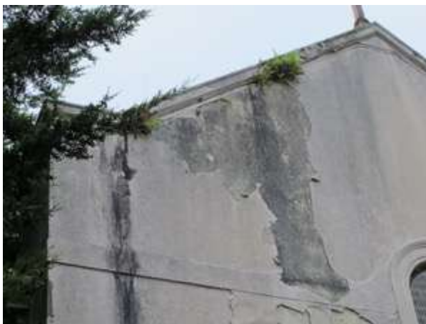
Fig.69: East elevation, damage to exterior wall and plant growth along mouldings
