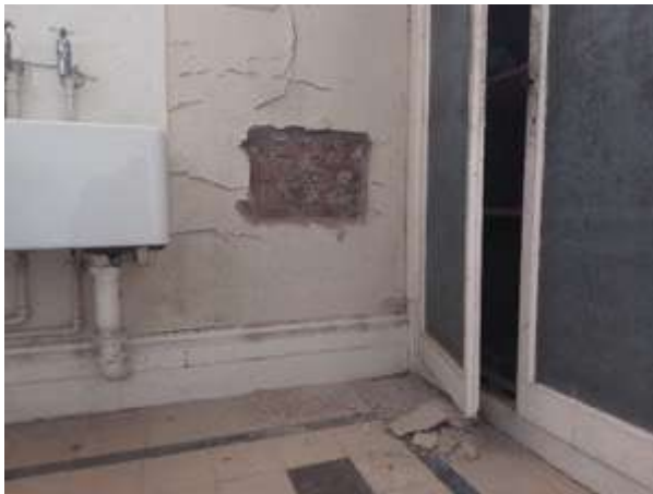
Fig.100: Example of interior wall opening up works showing red brick (EXG-08)
