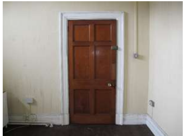
Fig.116: Ground floor six-panelled timber door (EXG-16)
