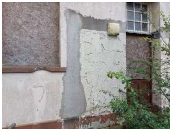
Fig.30: Evidence suggesting previous porch on north elevation
