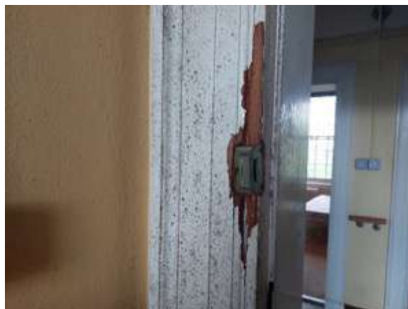
Fig.122: Damage and mould build up to timber frame (room EX1-22)
