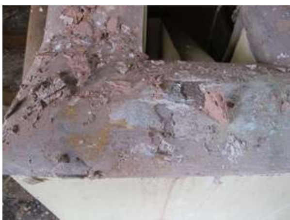
Fig.154: Damage to capping of concrete balustrade of east staircase to second floor (EX2-12)
