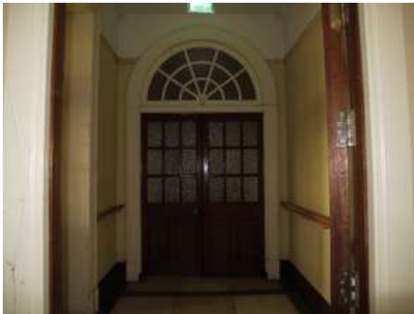
Fig.115: Ground floor corridor pair of timber panelled doors with nine glazed panes to upper portion and semi-circular glazed panelled overlight (EXG-03)
