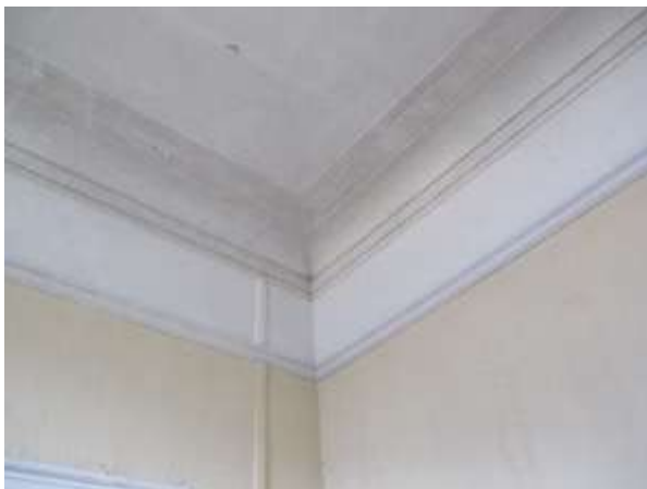
Fig.92: Simple moulded cornice (EXG-16)
