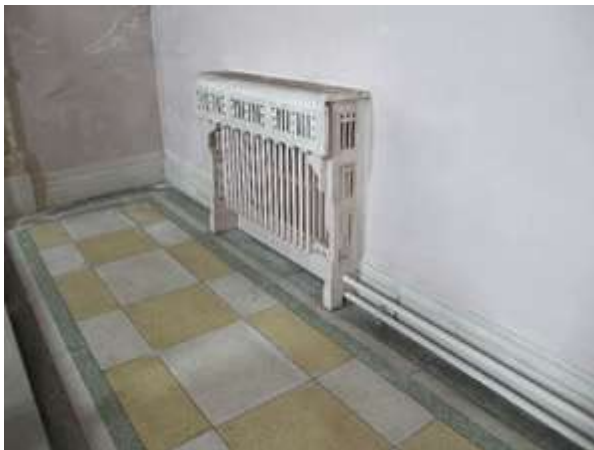
Fig.193: Cast iron radiator with timber cover
