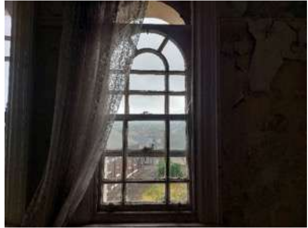
Fig.137: Typical timber sash window to south of second floor
