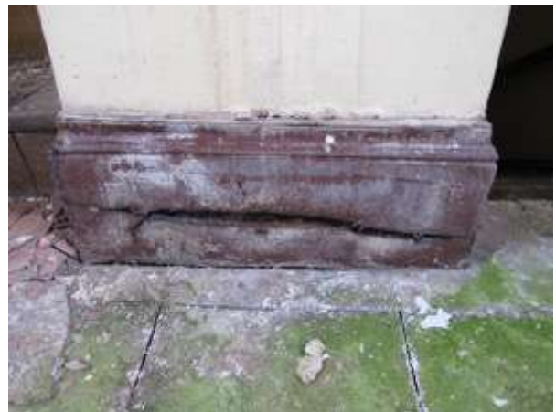
Fig.147: Water ingress and timber decay in skirting (EX2-12)
