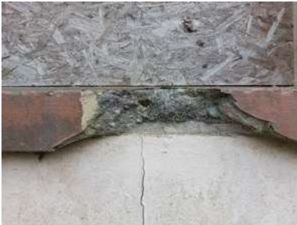
Fig.37: Damaged concrete windowsill
