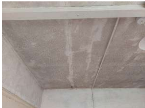
Fig.93: Mould growth and cracking to ceiling (EX2-07)
