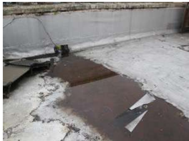
Fig.16: Water ponding (south-west area of roof)
