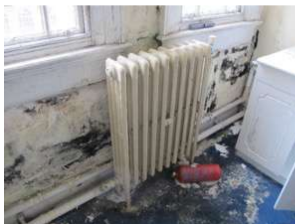
Fig.114: Mould and efflorescence on carpet overlay (EX2-17)
