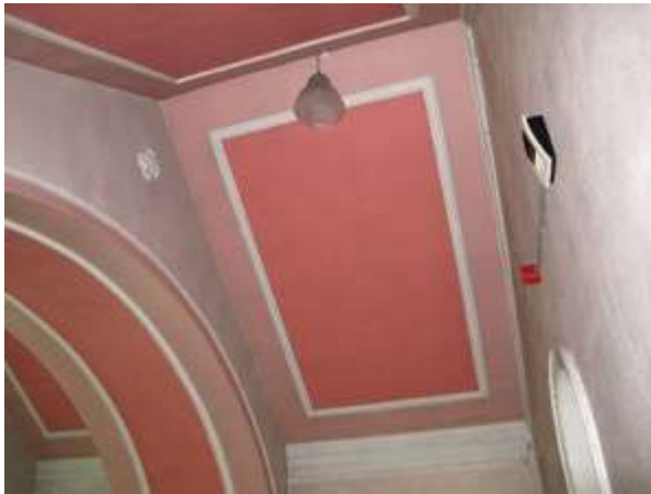
Fig.161: Plasterwork to ceiling and barrel vaulting.
