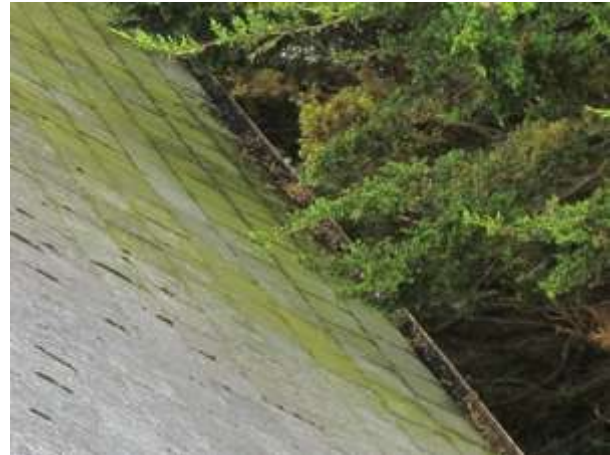
Fig.78: Debris in south elevation gutter
