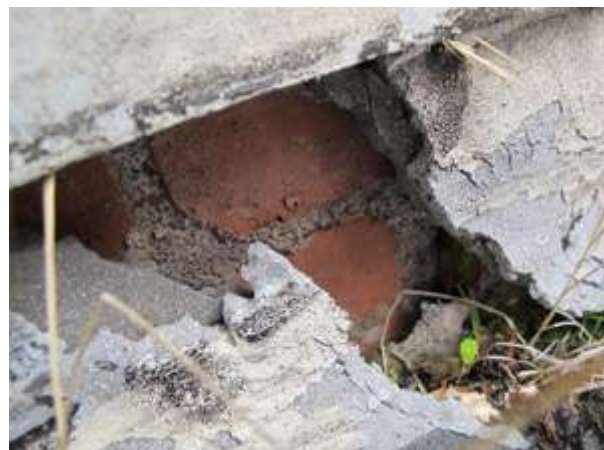
Fig.14: Damaged parapet render exposing red brick
