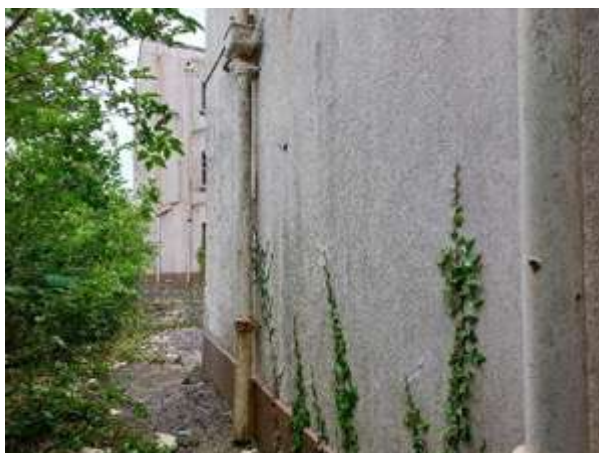
Fig.29: Ivy and algae growth on north elevation
