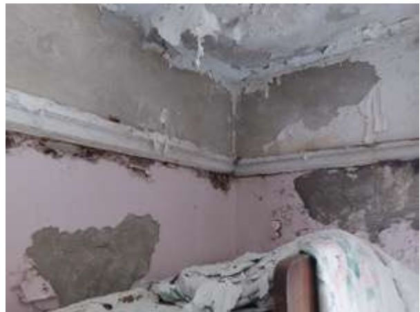
Fig.149: Damaged timber picture rail (EXG-05)
