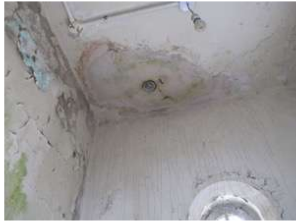
Fig.95: Bell tower ceiling showing signs of water ingress and previous repair (EX2-16)
