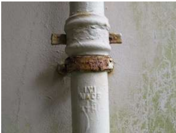
Fig.20: Down pipe on west elevation marked 'I.V.I MADE IN ATHY'
