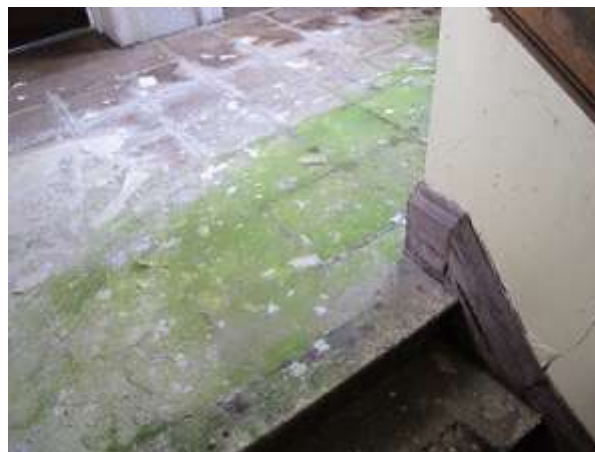
Fig.112: Damage to cork tiles under previously leaking water tank at second floor east staircase (EX2-12)
