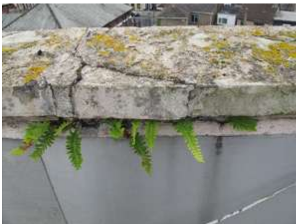
Fig.13: Plant growth and cracking to south concrete coping
