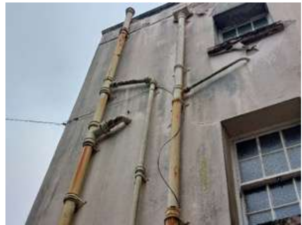
Fig.23: Rust to brackets and down pipe
