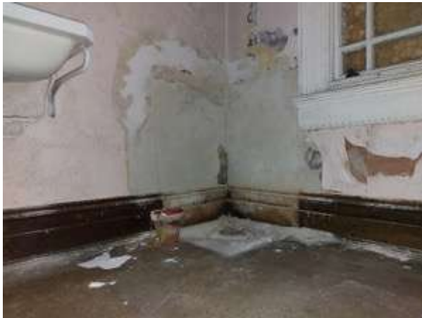
Fig.187: Stained and damaged timber skirting (EXG-29)
