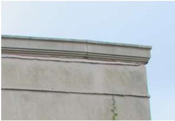
Fig.73: Cracking of concrete coping on sacristy annex
