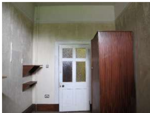
Fig.120: Example of timber panelled door with upper glazed panes (EXG-09)
