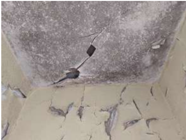
Fig.94: Mould build up and consequent damage to ceiling (EX1-03)
