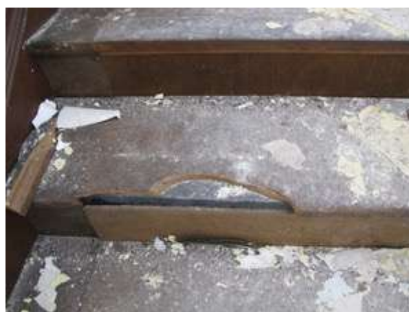
Fig.155: Damage to cork tile on west staircase to roof (EX2-01)
