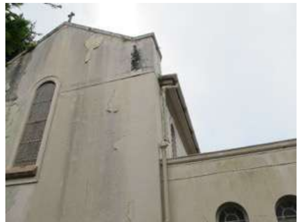
Fig.76: Gutter and down pipe on east elevation
