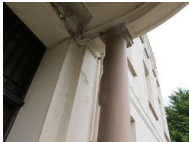
Fig.45: Bulging impermeable paint on column trapping water
