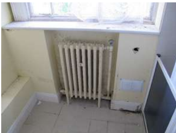
Fig.160: Rusting to radiator (EX2-10)
