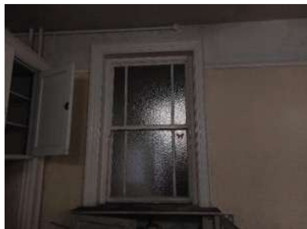
Fig.133: Interior timber ogee sash window (EXG-02) with opaque textured glass
