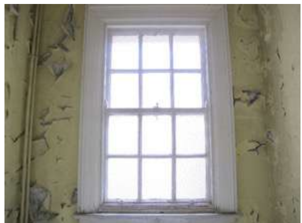
Fig.141: Standard timber window surround seen throughout building
