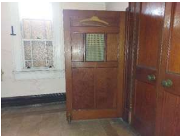
Fig.195: Hinged timber screen wall in sacristy (EXG-29)
