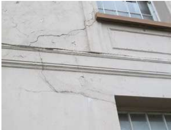
Fig.9: Cracking on south elevation
