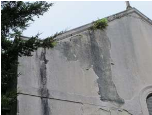
Fig.81: Algae growth on east elevation
