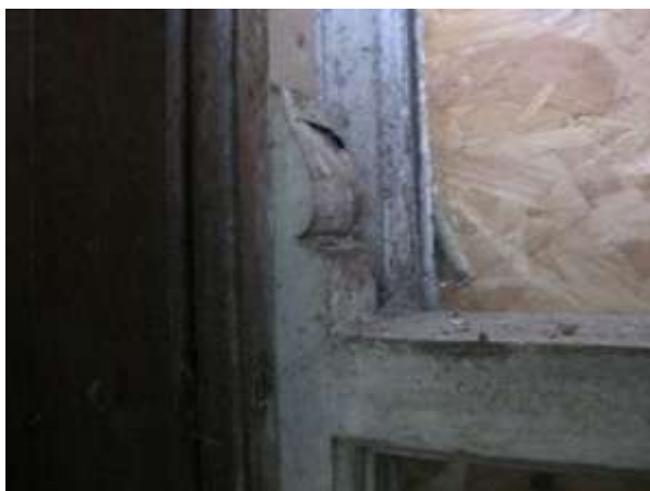
Fig.132: Timber ogee horn (EXG-16)
