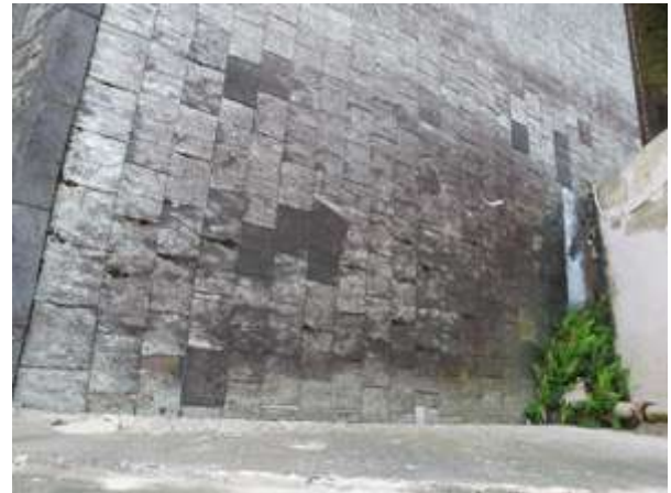
Fig.57: Blocked drainage at bell tower north wall
