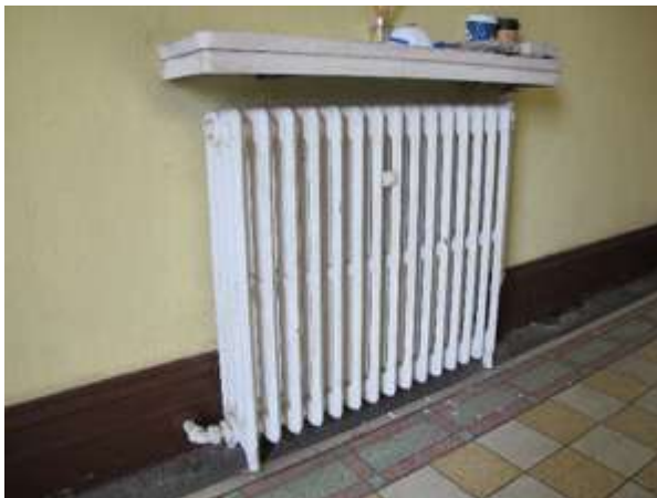
Fig.158: Example of cast iron radiator (EXG-01)
