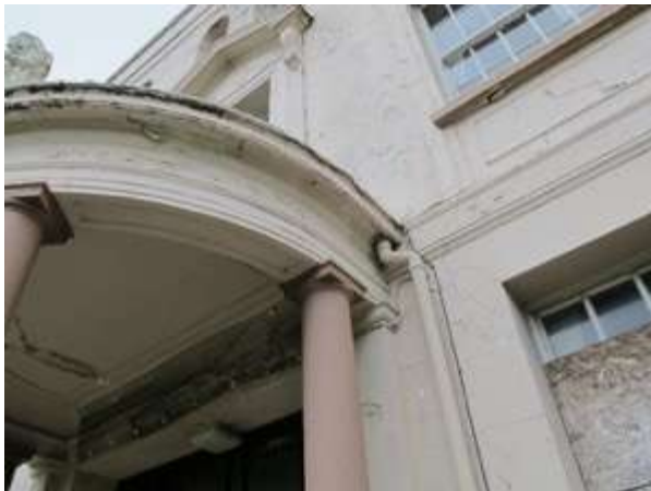
Fig.46: Biological growth to the entablature
