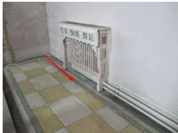
Fig.172: Slight crack to terrazzo indicated with red arrow (south side of altar)
