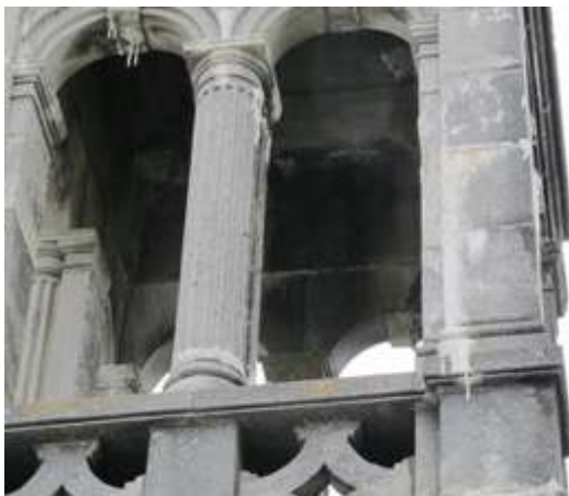
Fig.52: Damp staining, leaching, deposits and stalactite formations to final stage
