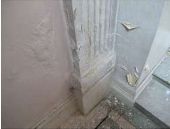
Fig.163: Bubbling to rendered plaster wall and surround
