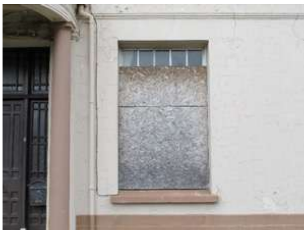
Fig.17: Modern plastic down pipe on south elevation
