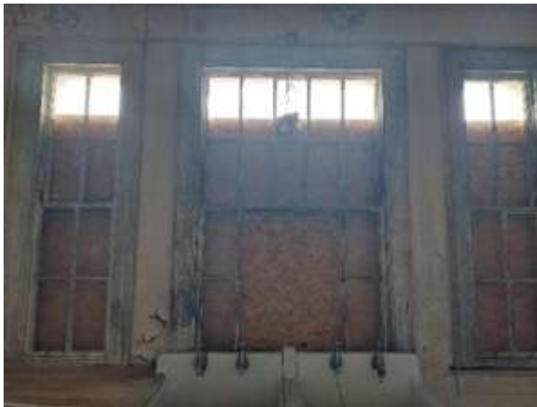
Fig.138: Example of timber sash with missing glazing panes and bars in west annex (EXG-19)
