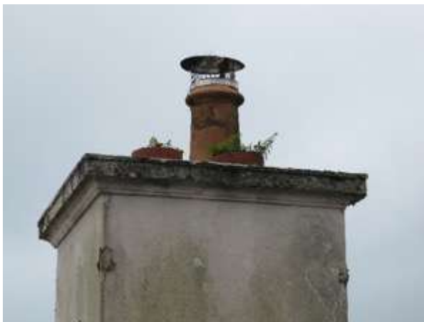
Fig.15: Plant growth in terracotta chimney can
