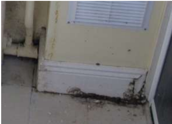
Fig.144: Growth on timber skirting (EX2-10)
