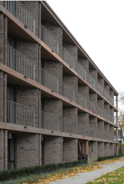
Fig 7 - Steel balustrades
