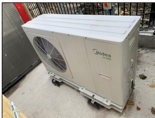
Figure 10: Air-Source Heat Pump
