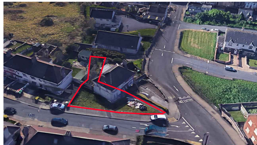
Aerial photo of the site, viewed from the north.
