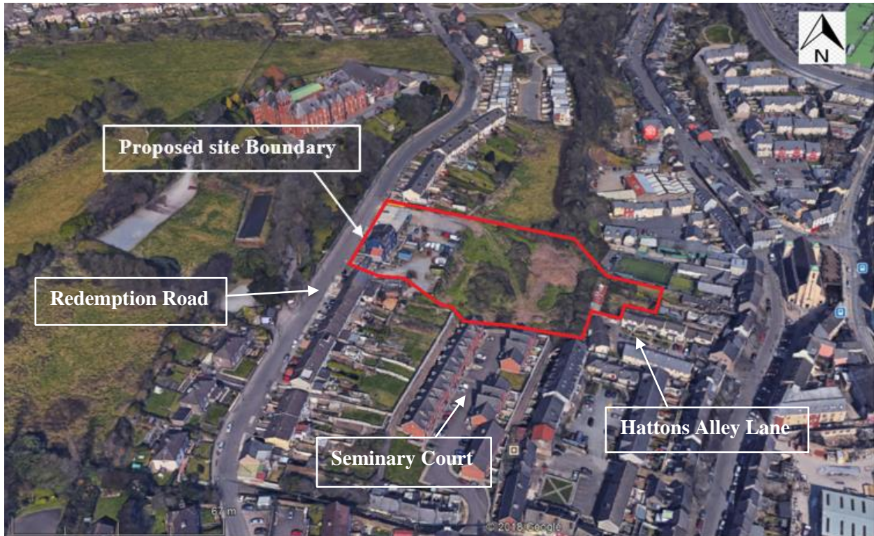
Figure 3. Project site aerial photograph (Data Source: Google Earth, 2018).
