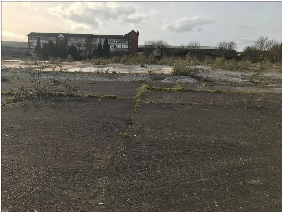
Figure 5. Internal view of the northern section of the site, looking west.
