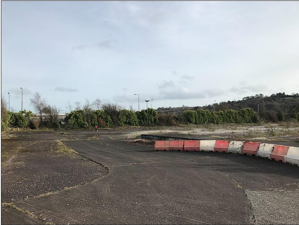
Figure 4. Internal view of the site looking south-east from inside the site entrance on Tramore Road.
