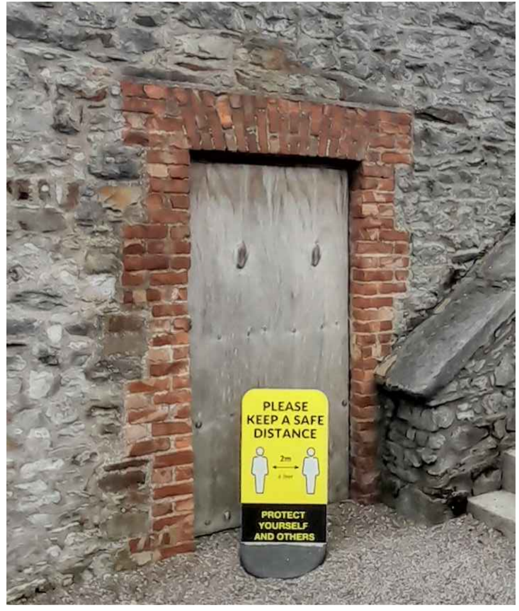
05 EXISTING EXTERNAL VIEW 106
