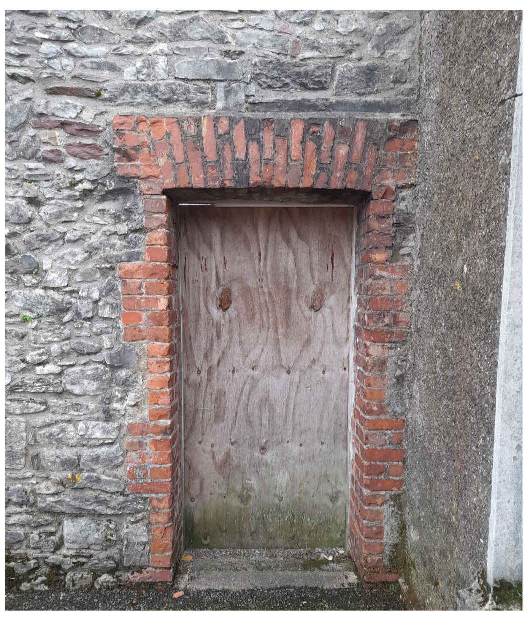
04 EXISTING INTERNAL VIEW 106
