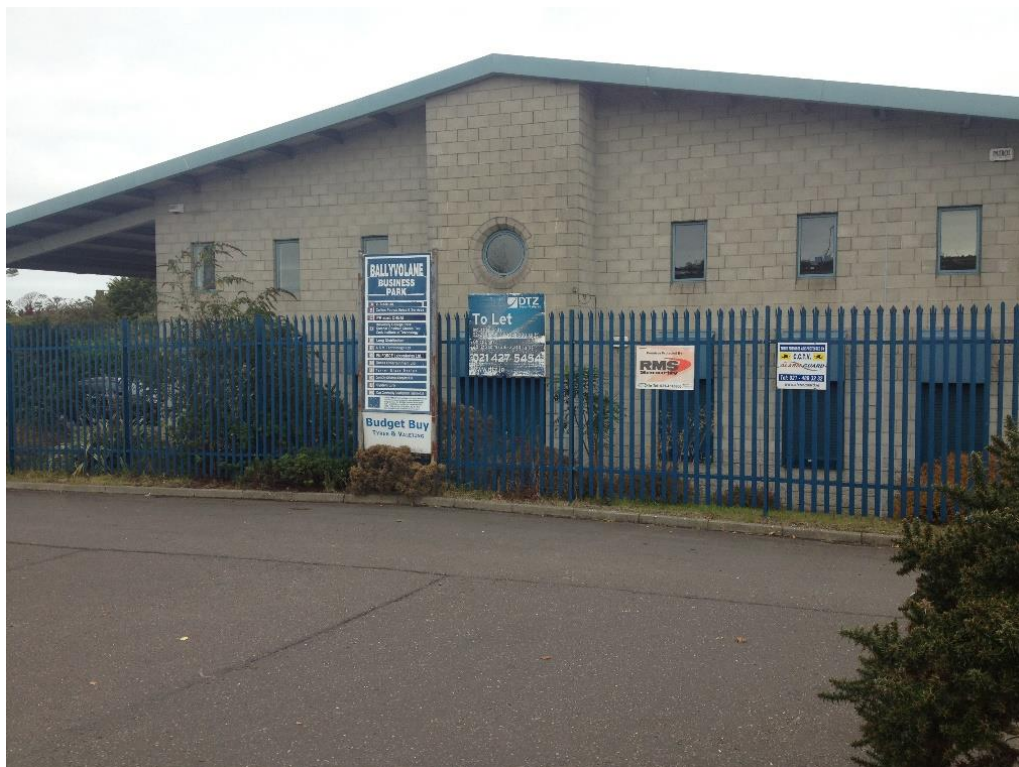
Fig 4 – Ballyvolane Enterprise Centre – Front façade 2016
