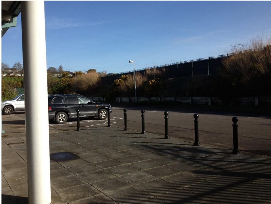
Fig 7 – Northside For Business Campus Eastern boundary fence intact.
