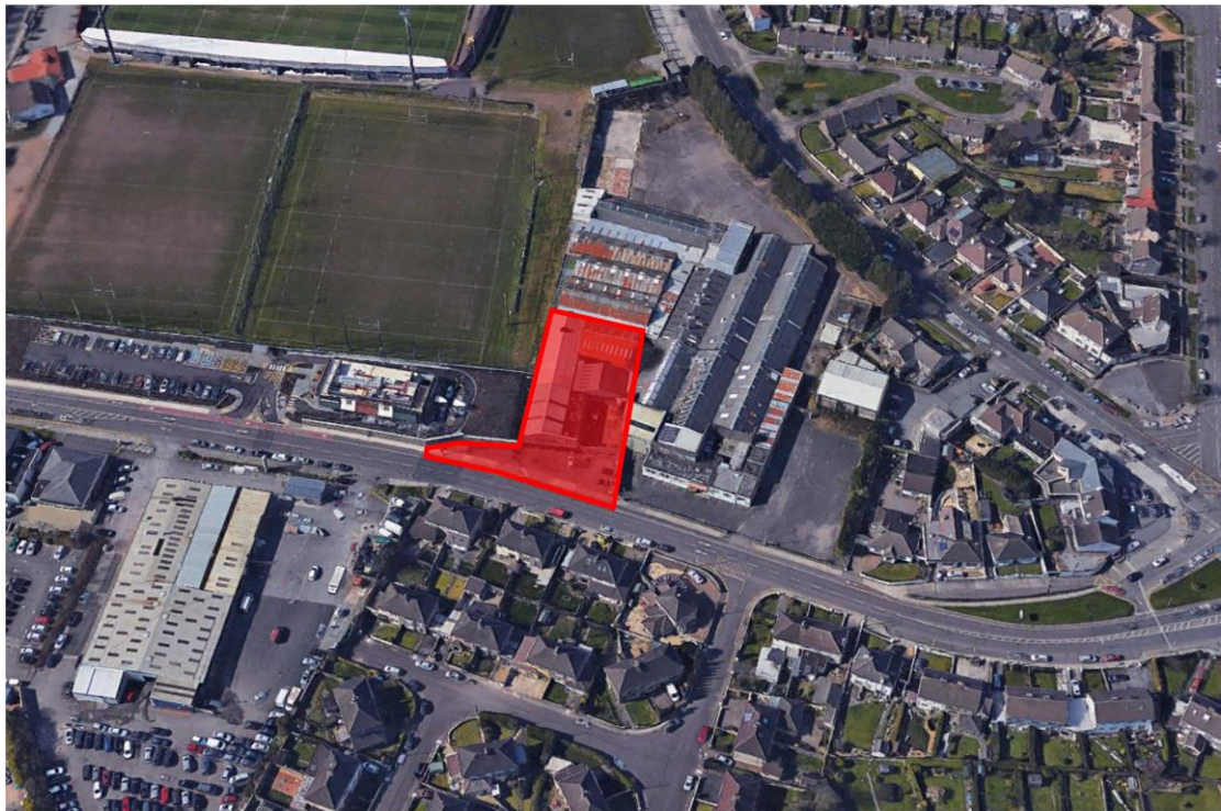
AERIAL VIEW OF SITE FROM THE EAST
