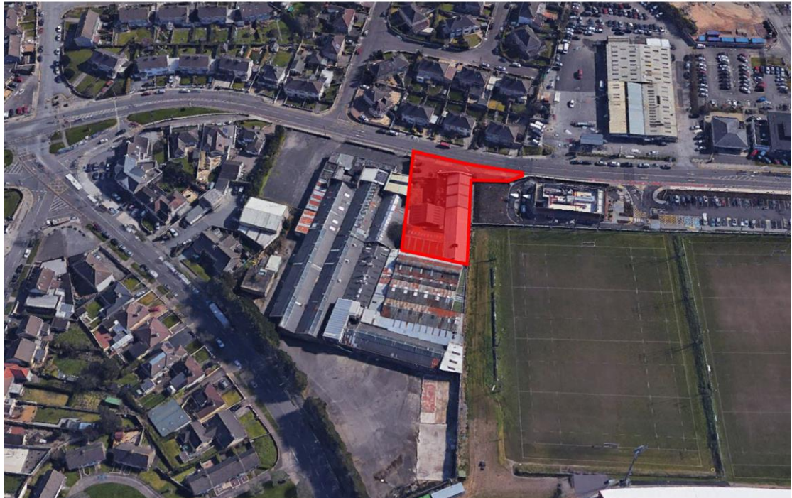
AERIAL VIEW OF SITE FROM THE WEST
