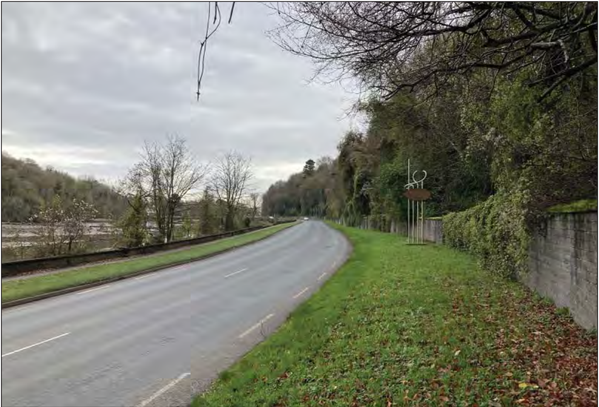
Plate 5 - R639 along the Glashaboy River with eastern footpath and western walls, looking south
