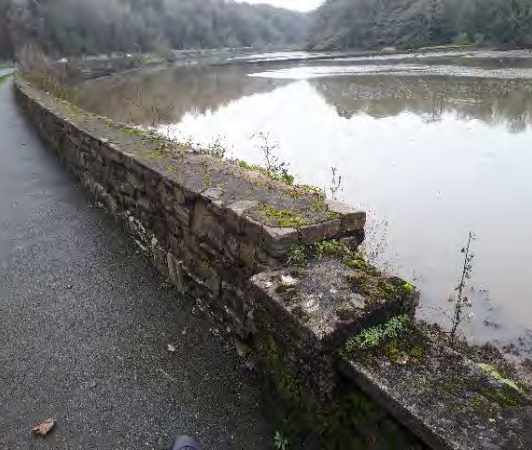
109. General view to stone wall
