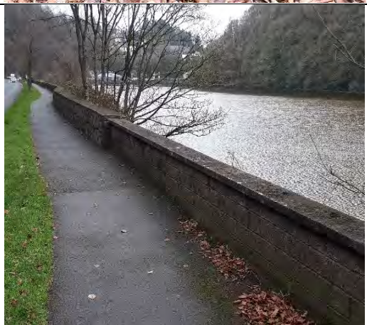
142. General view to wall
