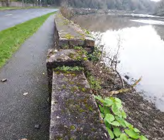
110. General view to stone wall
