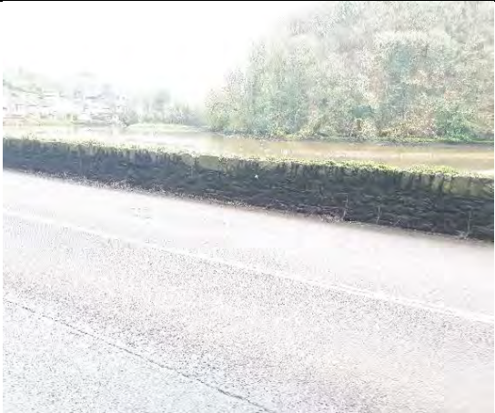
152. General view to the wall
