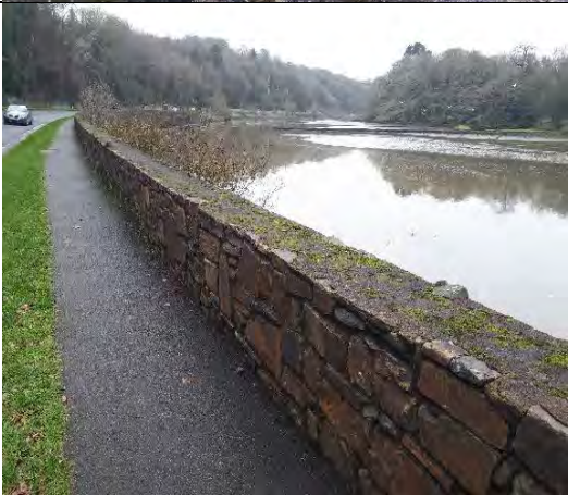
112. General view to the stone wall
