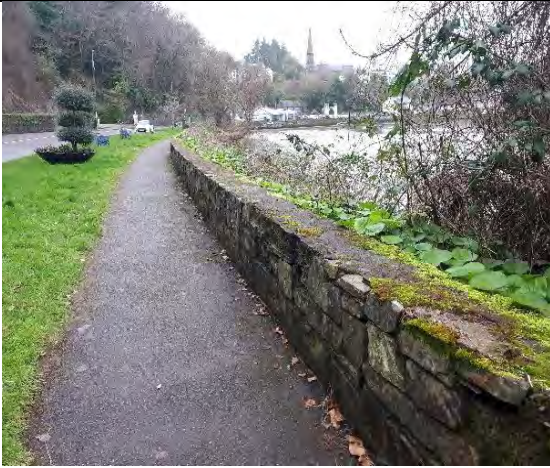
146. General view to the wall
