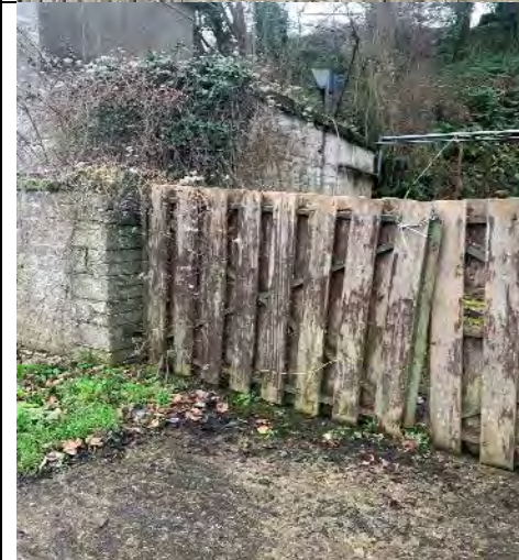
15. Top of pier collapsed
