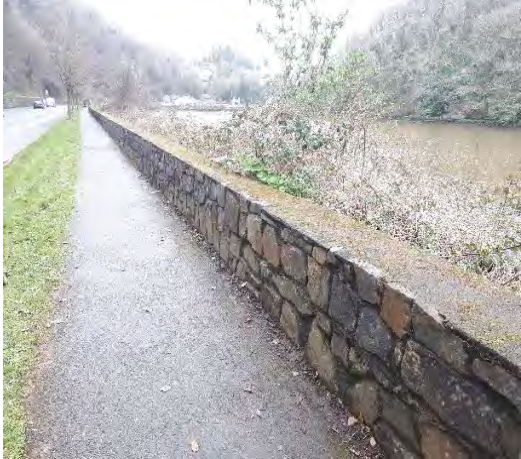
143. General view to wall
