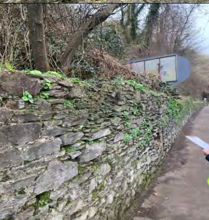
75. General view to the wall & minor vegetation growth present
