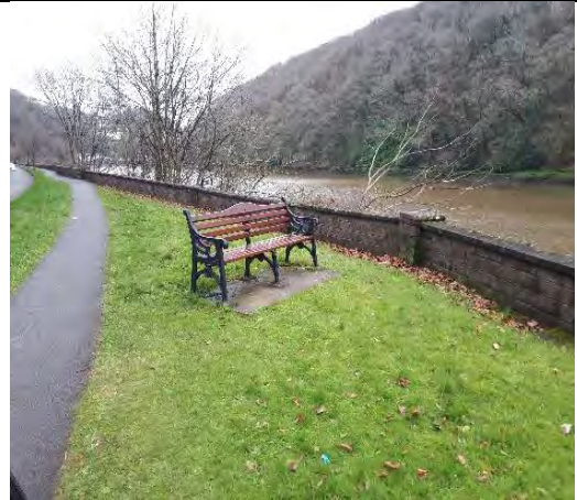
136. General view to wall
