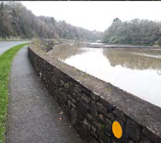
114. General view to the stone wall
