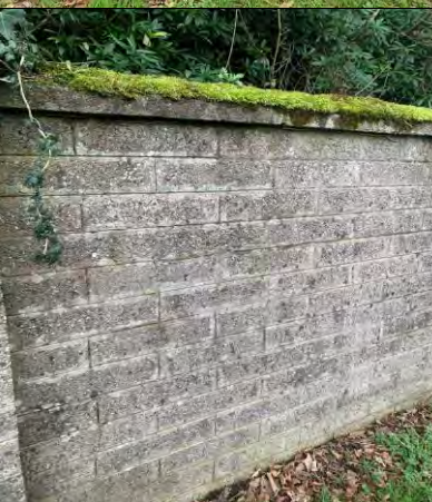
40. General view to the wall
