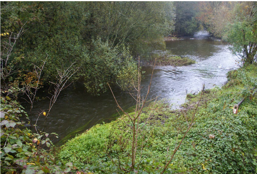
Photo 2: Glyntown Bridge downstream
