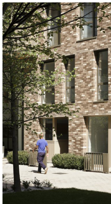
Ground floor patios with railings/ screen planting to public/communal open space (reference image)
