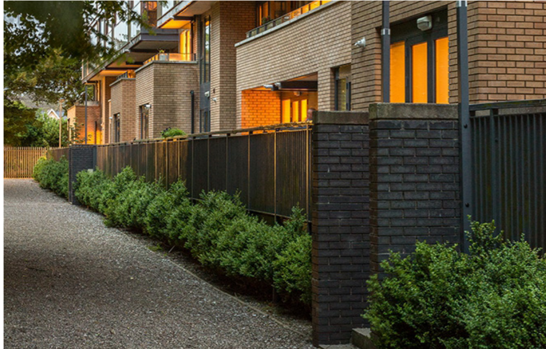
Ground floor patios with railings/screen planting to public/communal open space (reference image)
