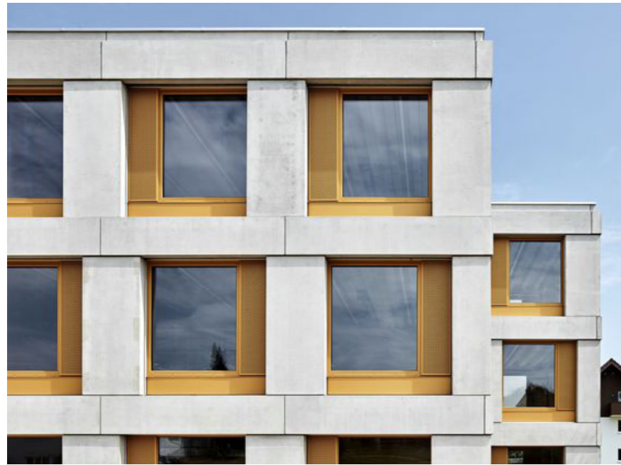
Windows and side panels contrasting with light grey panelised facade (reference image)
