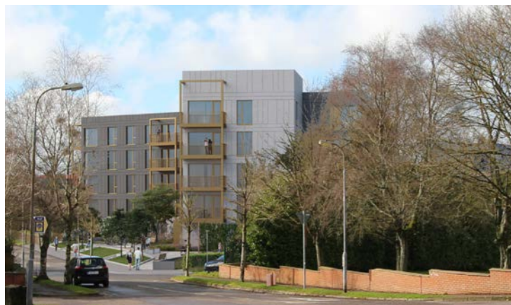
Taller gable element marks scheme entrance
