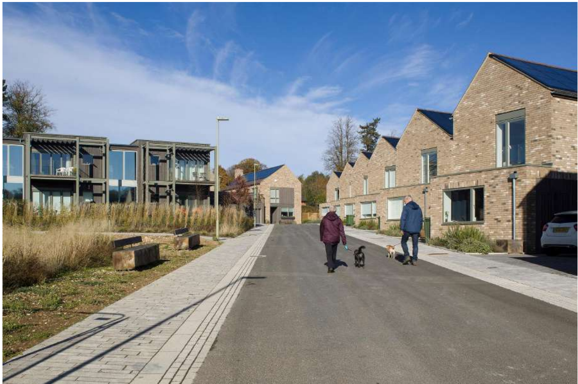
Exemplar image showing shared surface street with asphalt surfacing and cobble stripe edging
