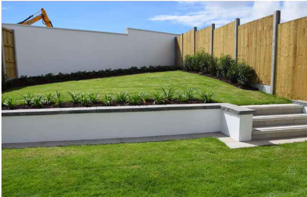
The rear garden boundaries are defined by a Concrete post and timber infill panels
