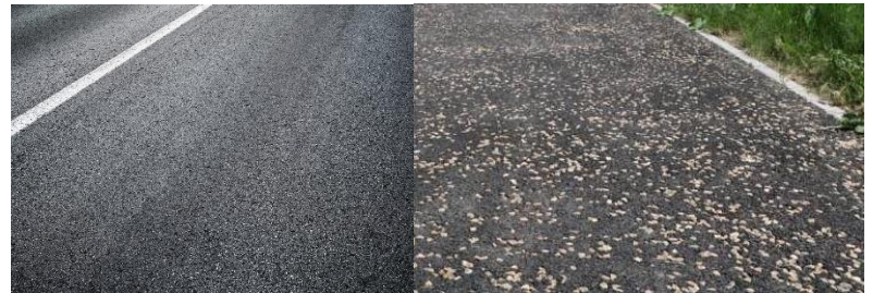
Hot rolled asphalt with variations in colour and texture provided by the inclusion of coloured aggregates or resin bonded surface finishes.
