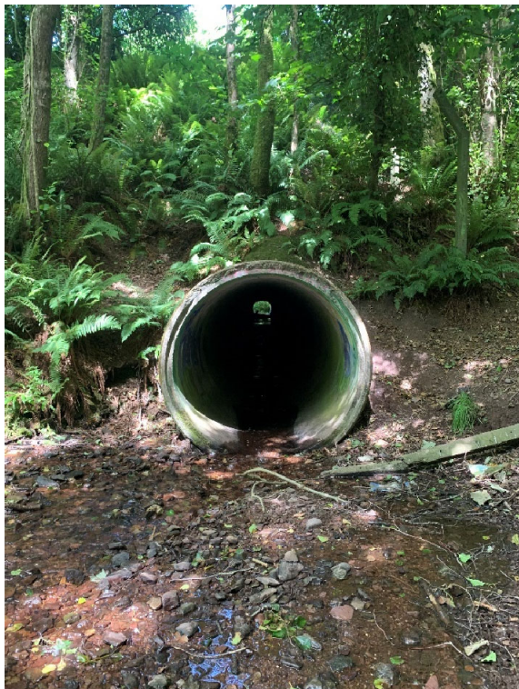
Plate 3-2: Concrete pipe culvert at the Douglas (Lee) stream
