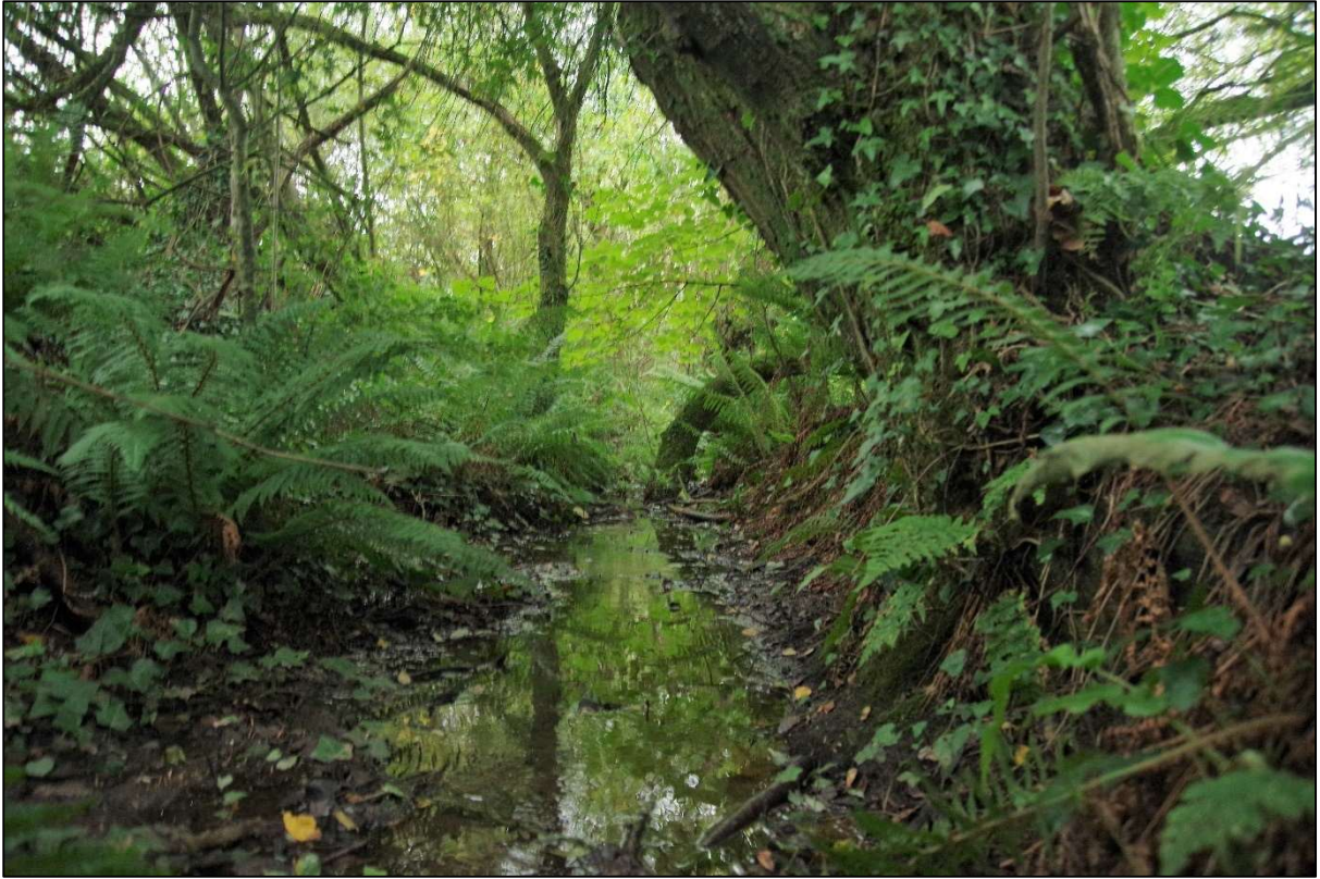
Plate 5: View of drainage ditch within overgrown area
