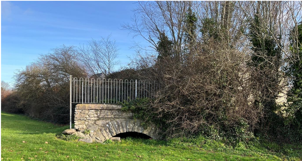
Figure 11: Railway bridge located to the rear of Carriganarra Estate
