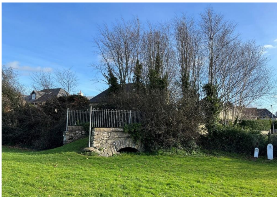
Figure 9: Railway bridge located behind 51 Carriganarra Estate
